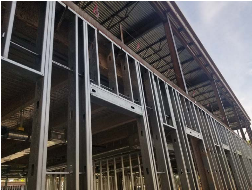
Exterior Window Framing
