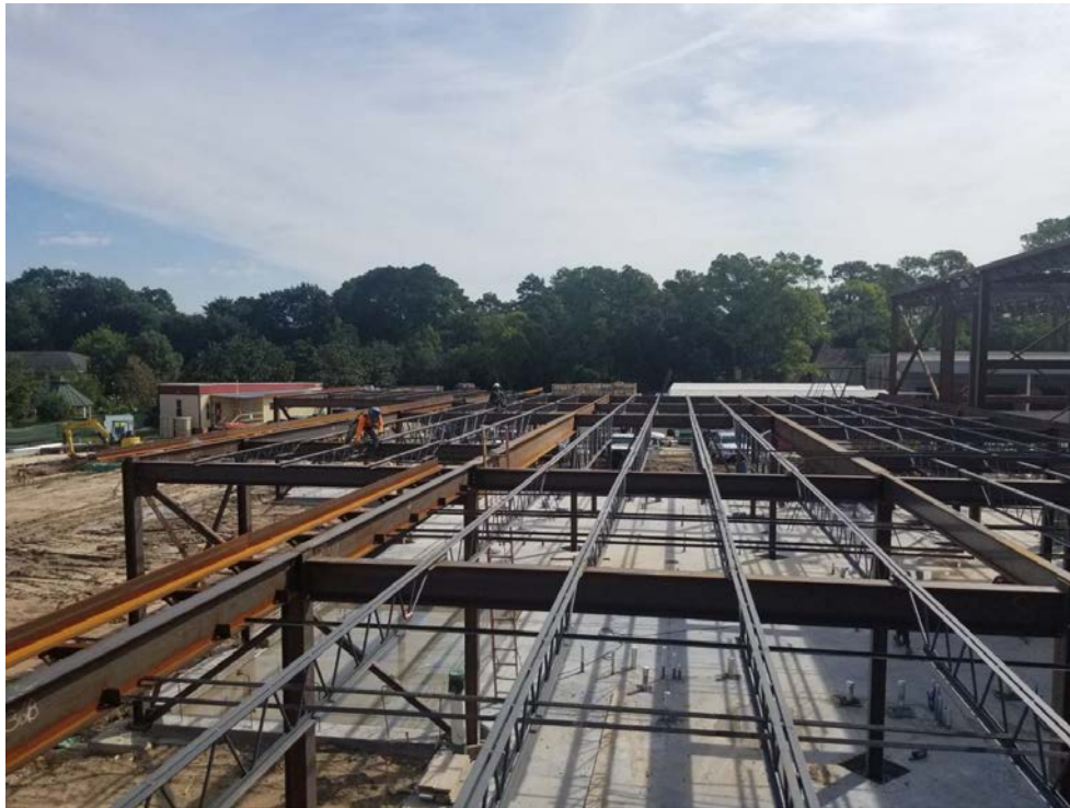
Roof Framing at Kitchen
