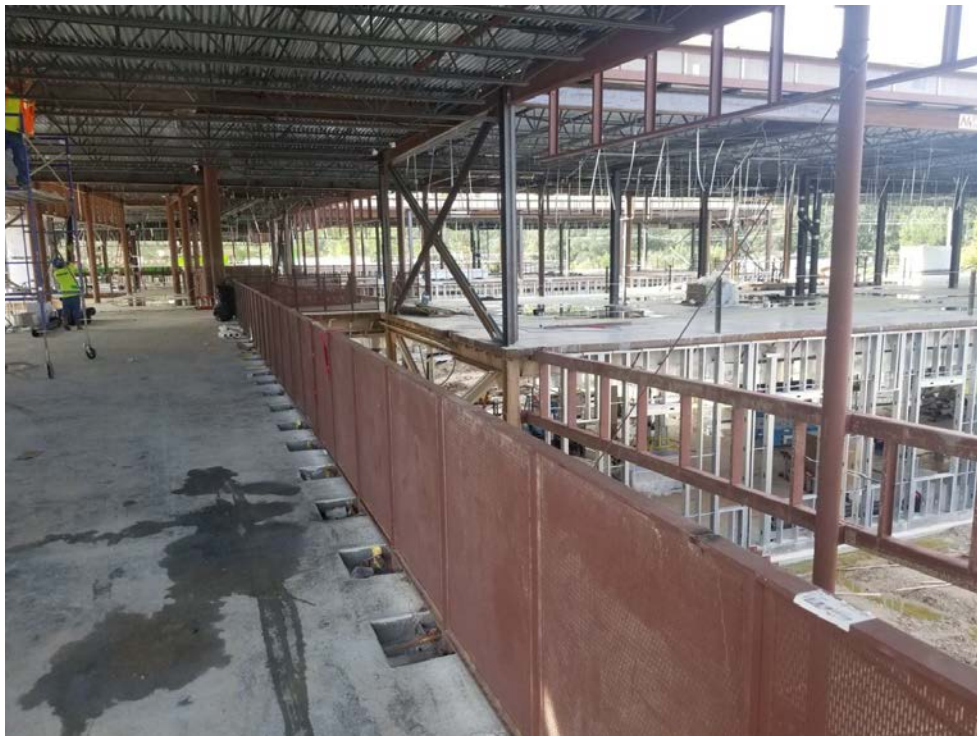
2 nd Floor Guardrail
