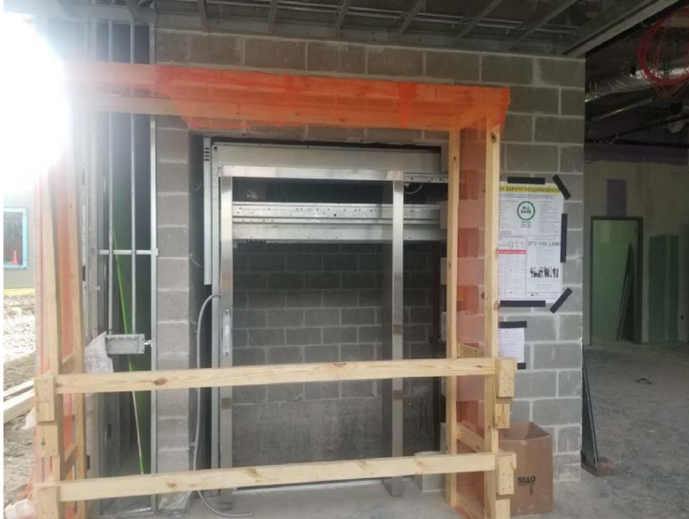
Elevator Installation
