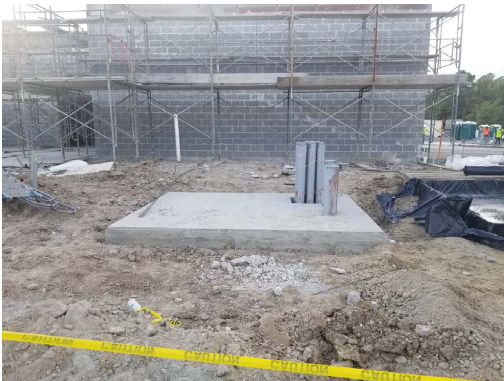
Transformer Pad ready for Equipment
