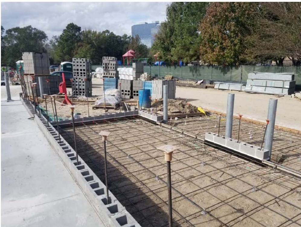
Slab and Wall Prep at Exterior Storage Building
