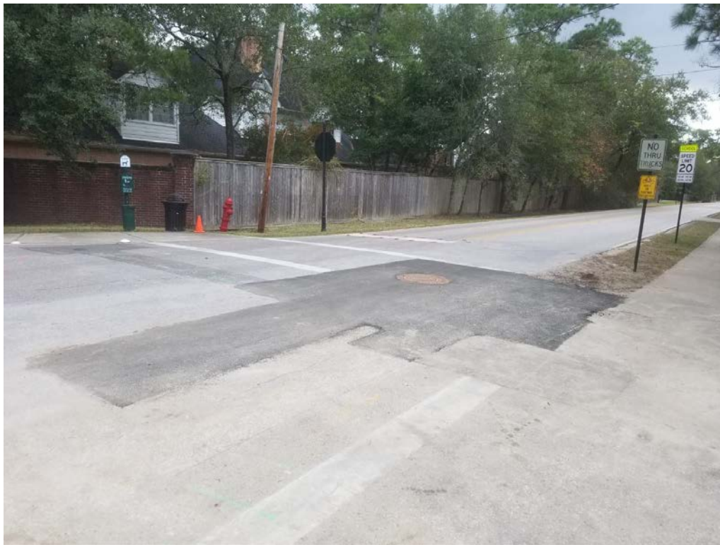
Street Patching at Underground Force Main Connection
