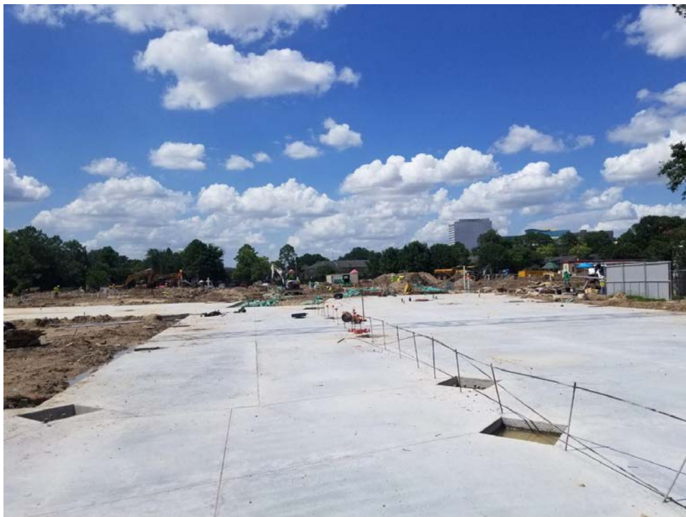
Area A & B Slab
