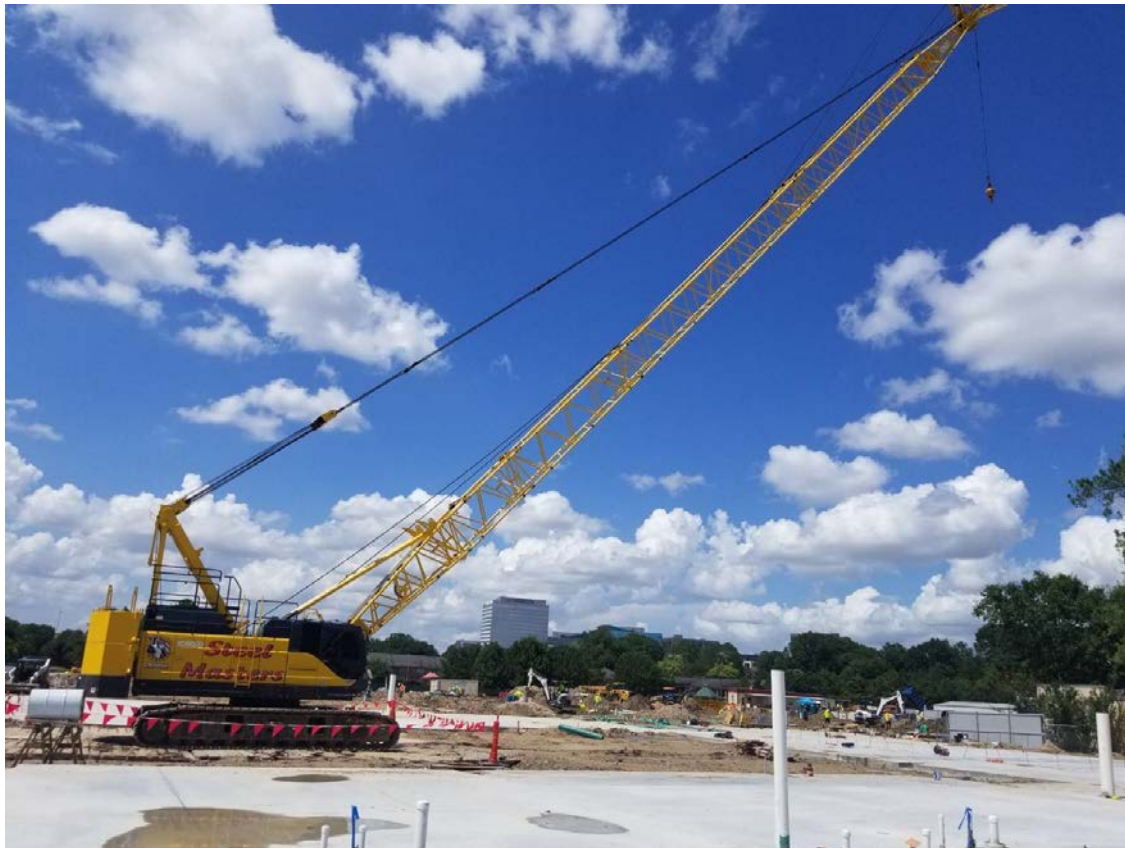
Crane ready for steel erection
