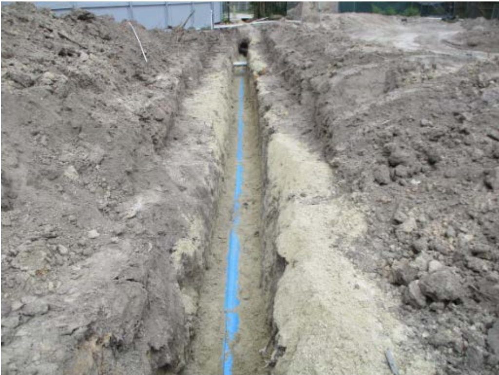
Water Line Installation
