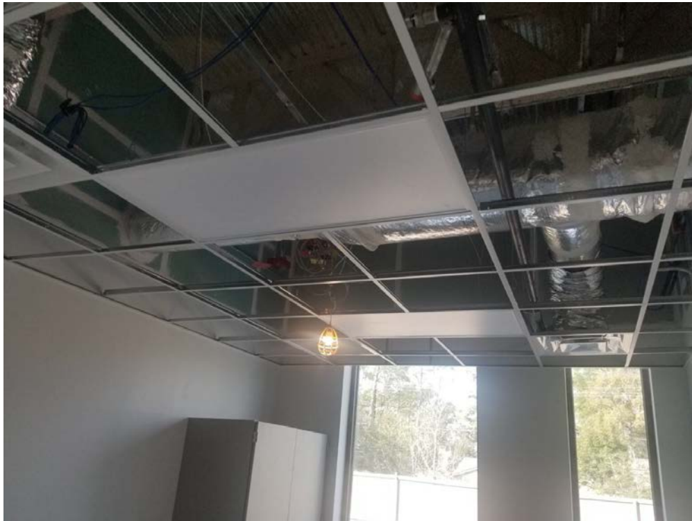
Ceiling Grid Install
