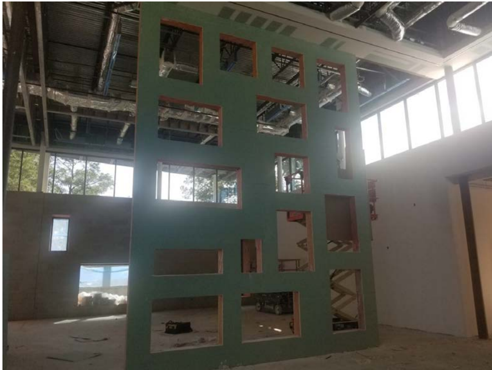
Jenga Wall Framing
