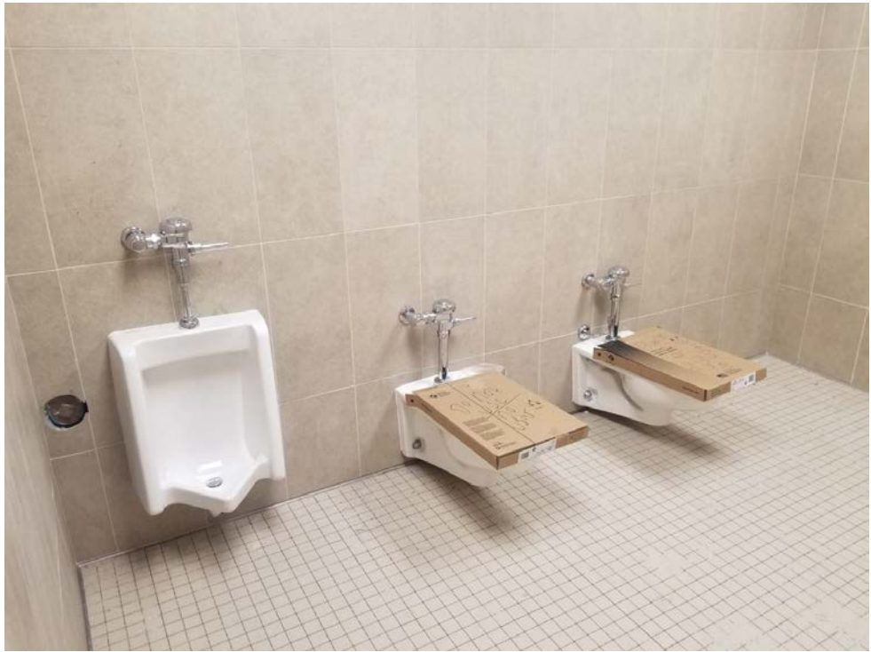
Restroom Tiling with Fixtures
