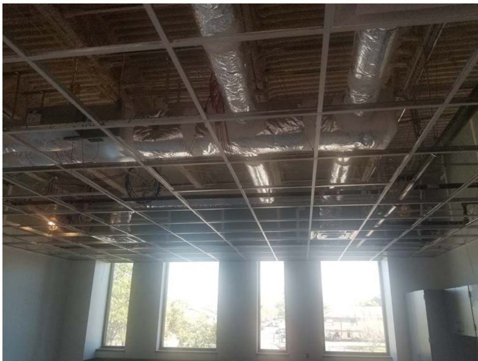
Classroom Ceiling Grid
