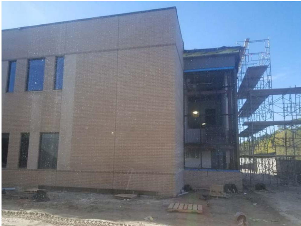
Classroom Wing Exterior at Stairs
