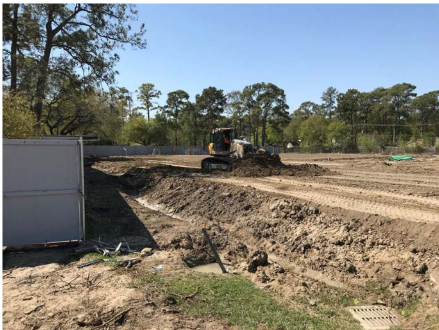
Grading for the Building Pad
