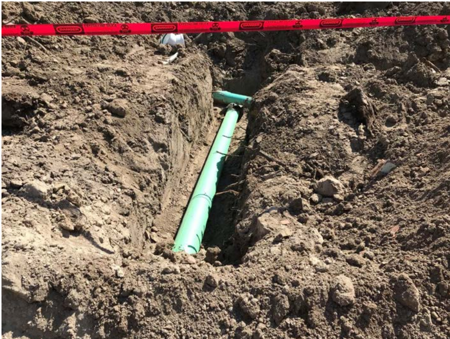
Underground utility installation
