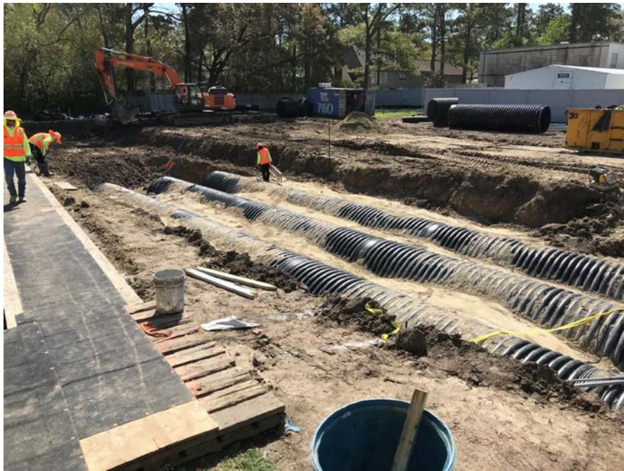
Storm Detention Install
