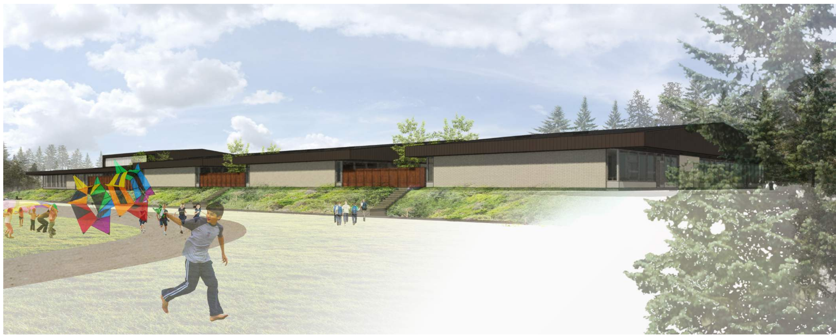
VIEW FROM TRACK + PLAYGROUND
