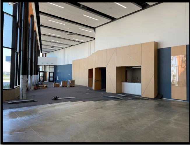
Finish carpentry and carpet flooring is nearing completion in the PAC Lobby
