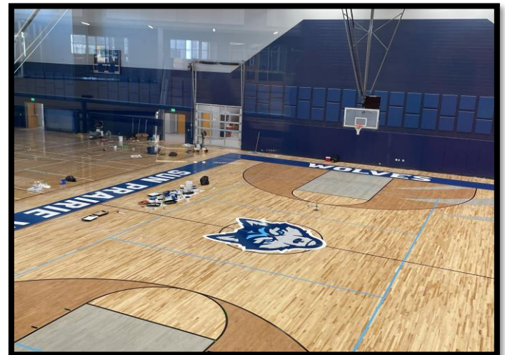
Striping is nearly complete at the Competition Gym. The floor will be sealed next week
