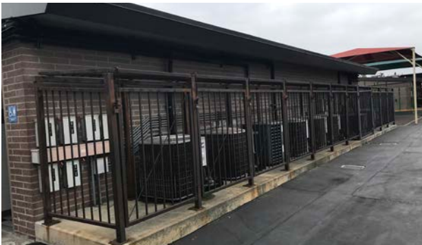
Mechanical unit condensers along back of Restroom building.
