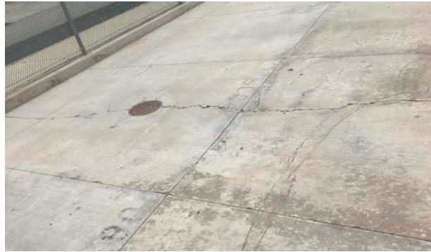
Cracked concrete panels.
