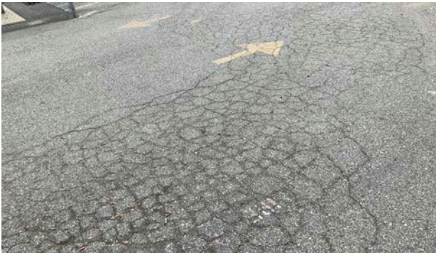
Cracking/degraded asphalt.
