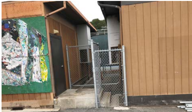
Missing handrail.
