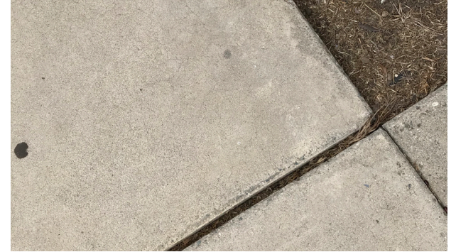
Degraded joint sealant.
