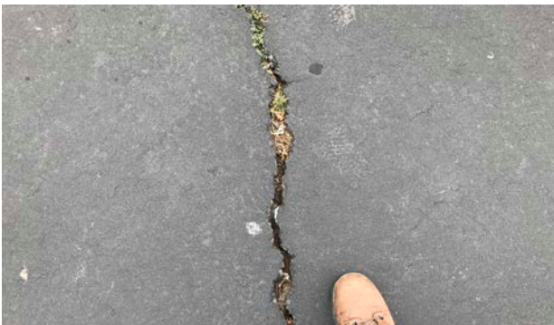
Large cracks in asphalt paving.
