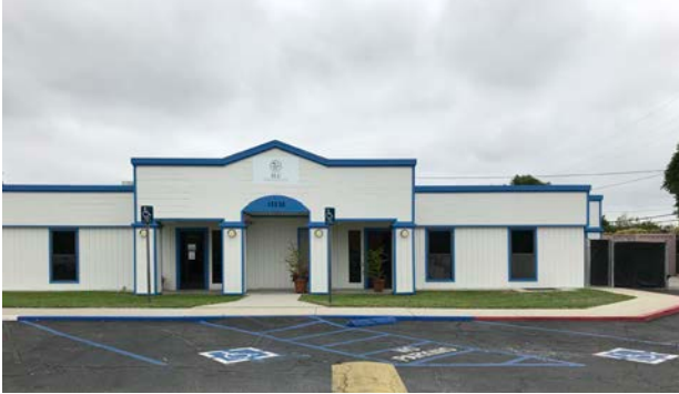
ADA stall length is non-compliant.
