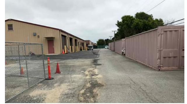
Degraded asphalt paving.
