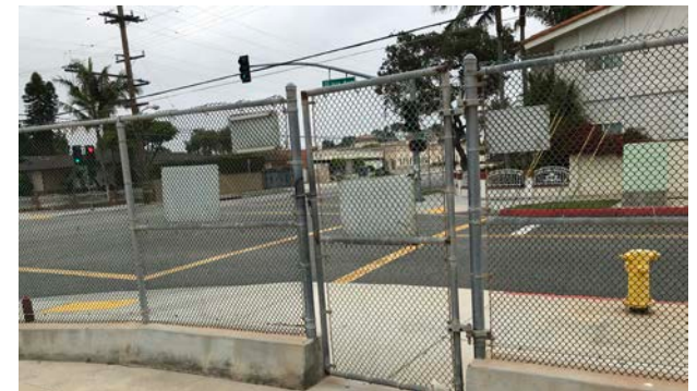
Gate missing accessible hardware.
