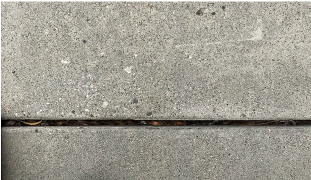
Eroded joint sealant.
