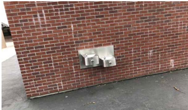
Missing cane detection rail.
