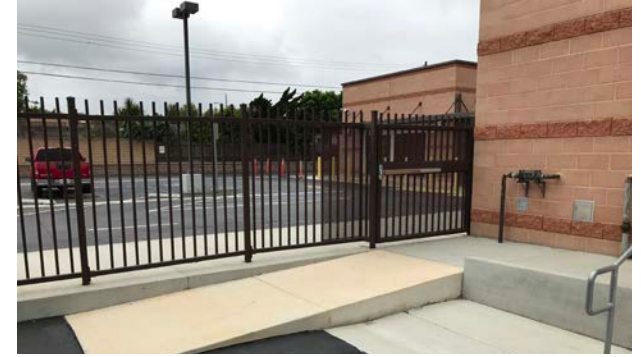
Missing handrails.
