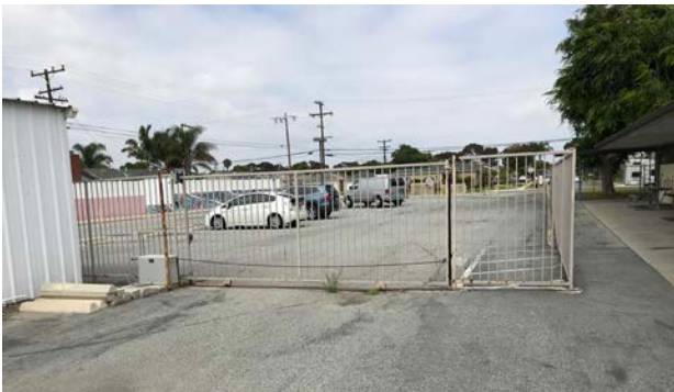
Tube steel fence/gate rusting.
