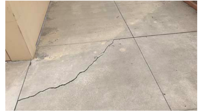
Cracked concrete panel.
