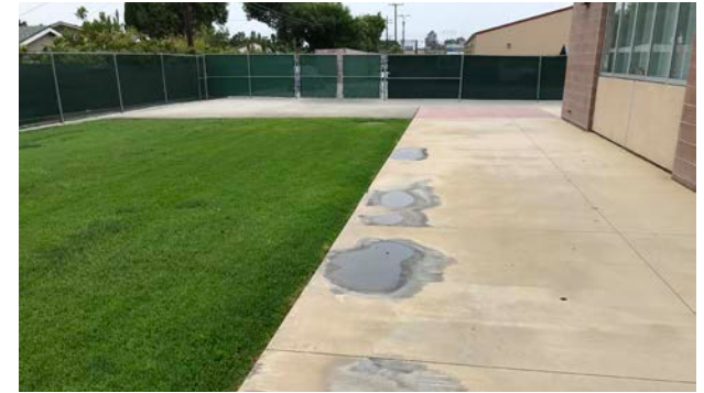
Low spots on paving.
