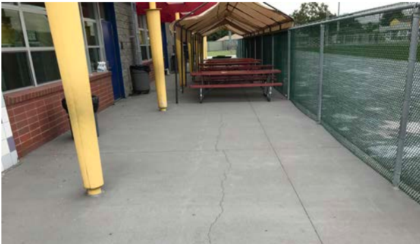
Cracked concrete.
