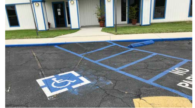
Compliant curb ramp and landing missing.
