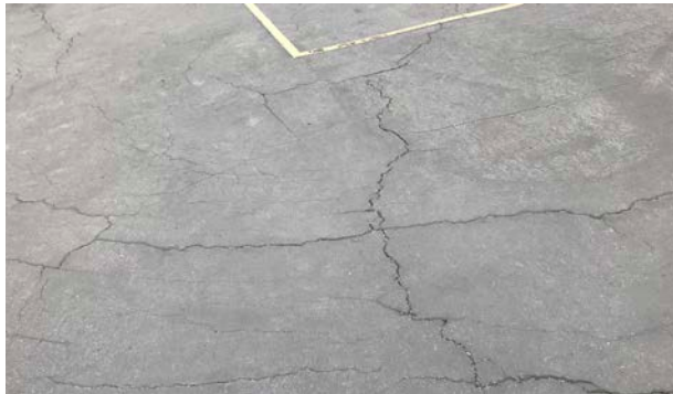
Crack asphalt paving.
