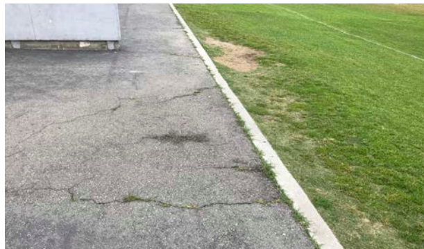
Degraded asphalt paving.
