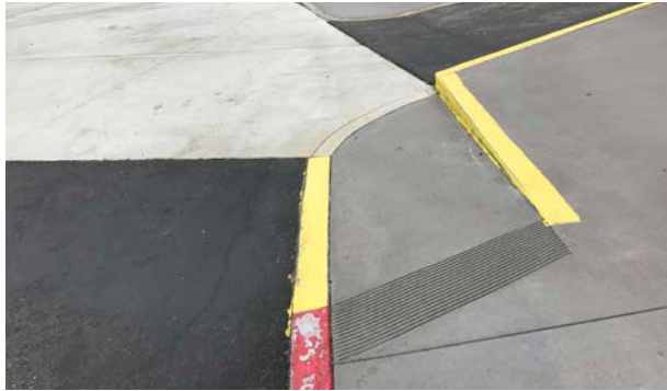
Truncated dome missing.
