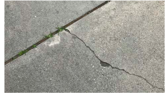
Cracked concrete.
