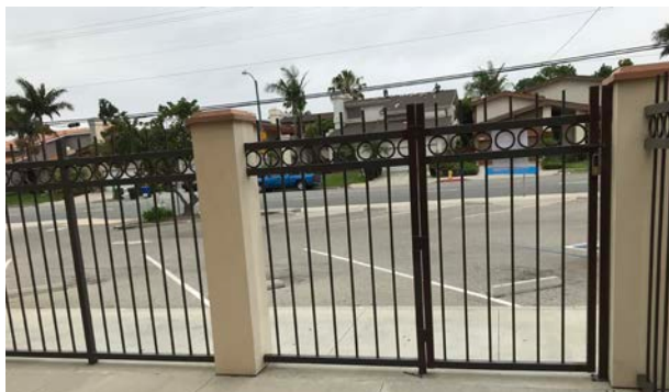
Tube steel fence in good shape.
