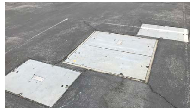
Rainwater infiltrates electrical boxes.
