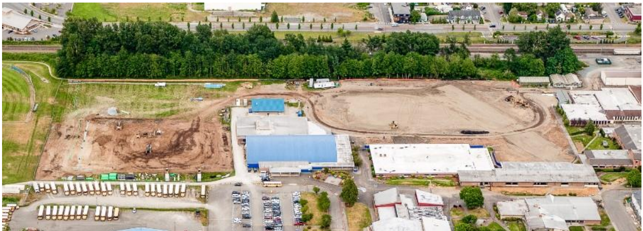
This is an aerial project photo from June 2021...
