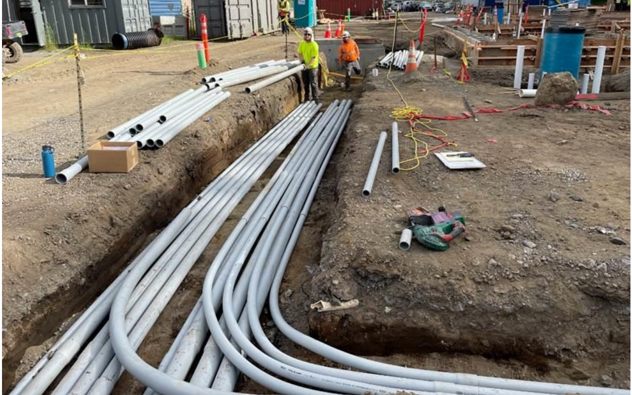
Underground electrical piping that will serve the CTE Village
