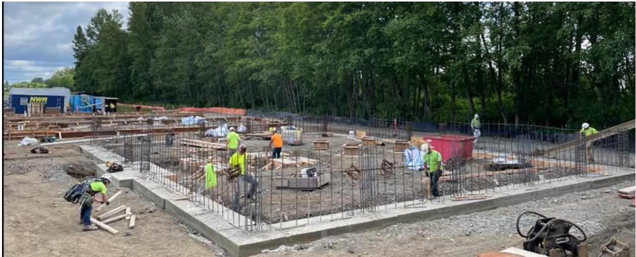
Ongoing foundation work at the CTE Village
