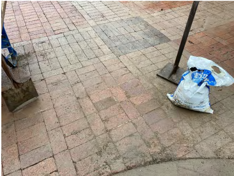
Photo 8: Pavers restored upon drilling of boring LB-02.
