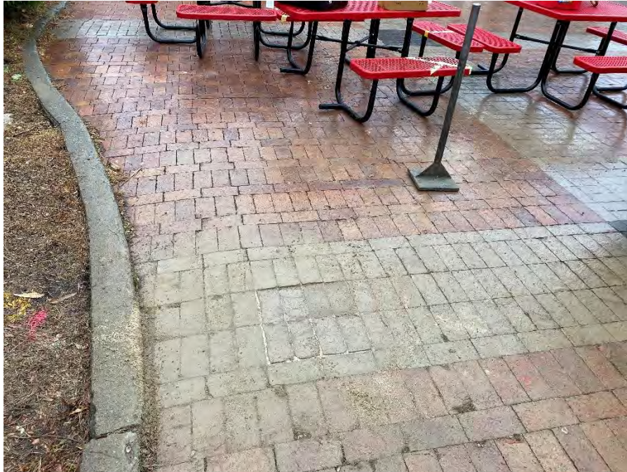
Photo 7: Pavers restored upon drilling of boring LB-01.
