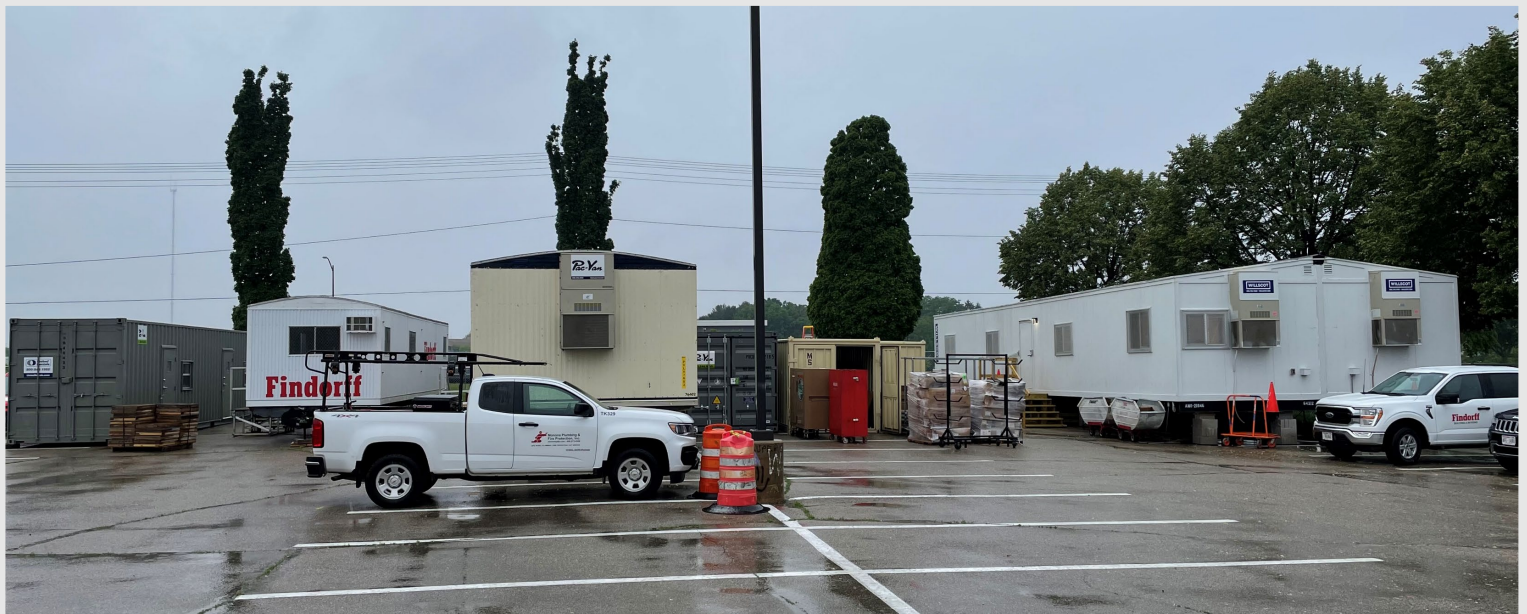
The west end of the south parking lot is quickly filling with construction materials and trailers
