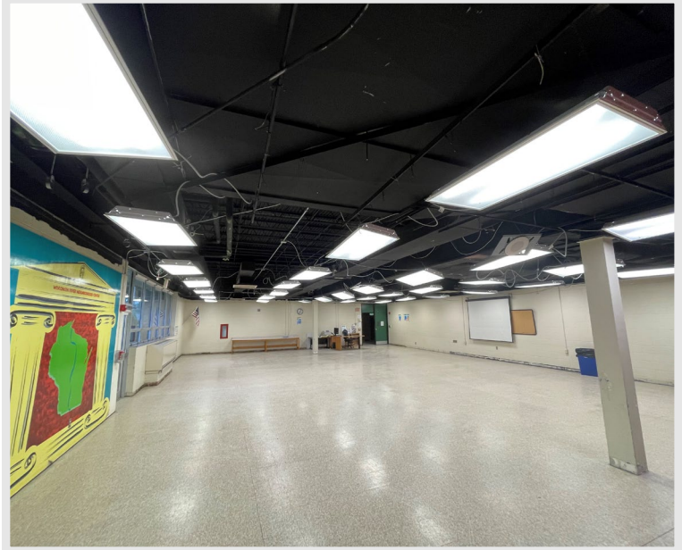
Ceiling removal is complete in a few areas of the school
