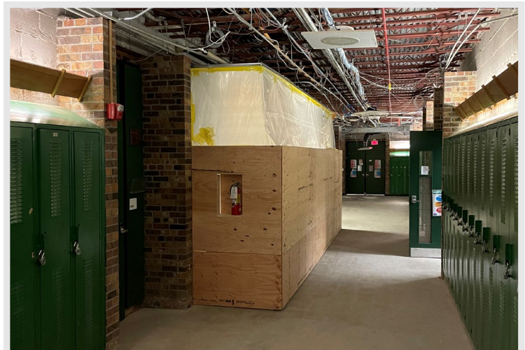
Ceiling removal and bathroom demolition have started on the first floor
