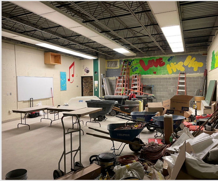
In the music room, ceilings were removed, and demolition of the existing walls is starting soon to make way for a new reconfigured layout
