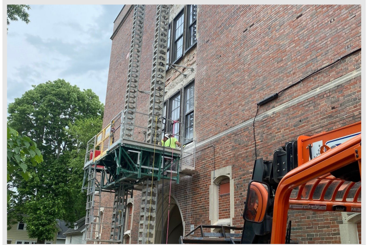
Construction crews are creating temporary access openings for the first phase of classroom renovations on the second and floors
