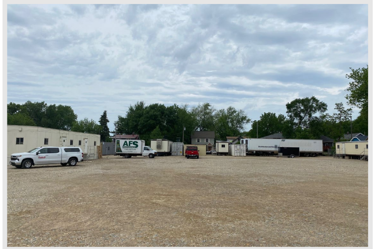
Construction trailers and equipment storage containers are on site at East High School
