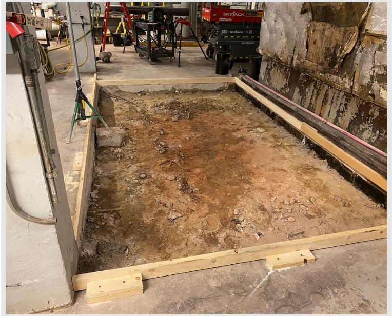
Preparing space for new boiler equipment to be installed
