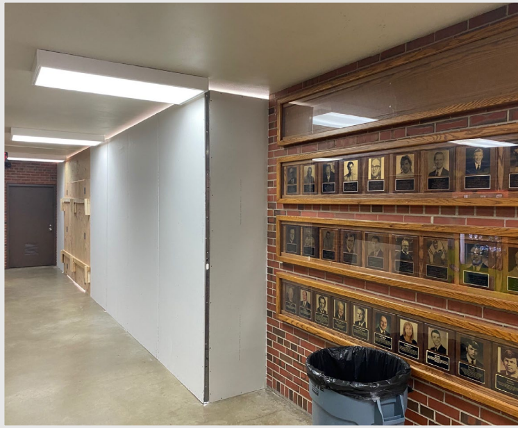
Temporary walls around the courtyard area ensure safety for students and staff during construction
