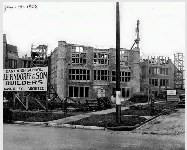
Historic photo of construction work at East High School on the corner of East Washington Avenue and 5 th Street
