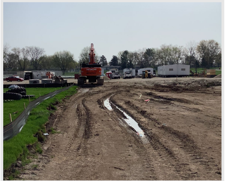
Construction trailers are on site and gravel is laid to prepare the site for construction activities
