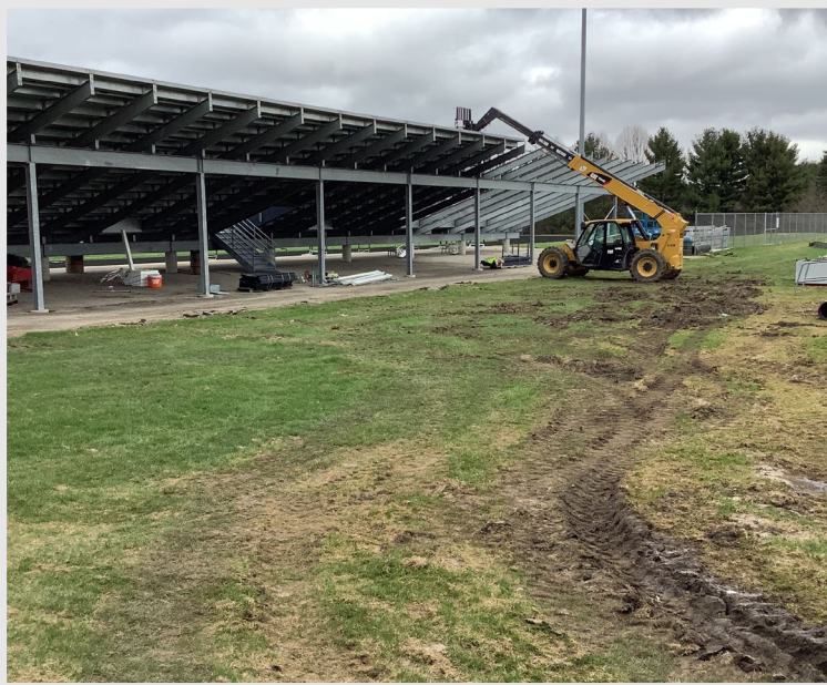
Removing exterior stadium bleachers in preparation for construction this summer
