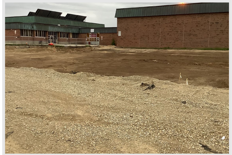
Preparing the site of the new athletic addition for excavation after Memorial Day
