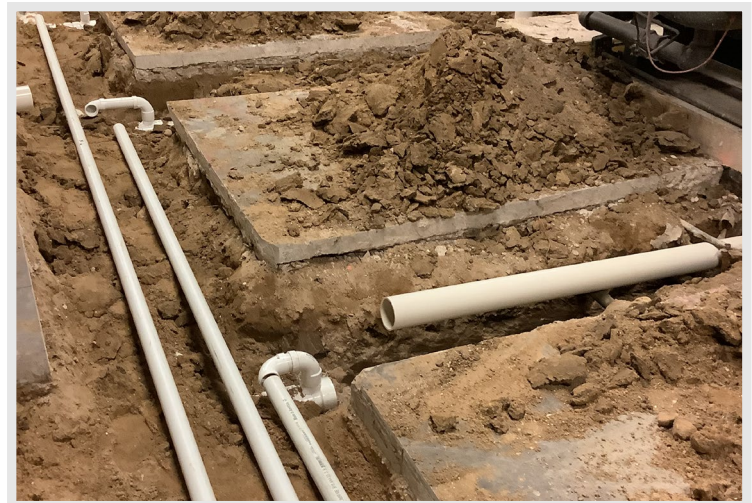
Concrete is cut and new pipes are installed in the boiler room
