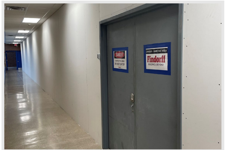
Temporary walls outside the library space ensure safety for students and staff during construction.
