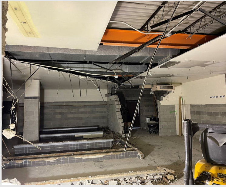
The old gym locker rooms were demolished to make room for new classrooms and instructional spaces.
