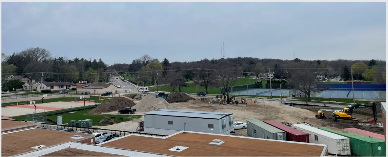
Piles of rocks and dirt placed on the football field are crushed to create gravel for construction activities.
