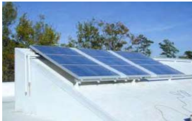
Solar collectors mounted on north-facing roof monitors
