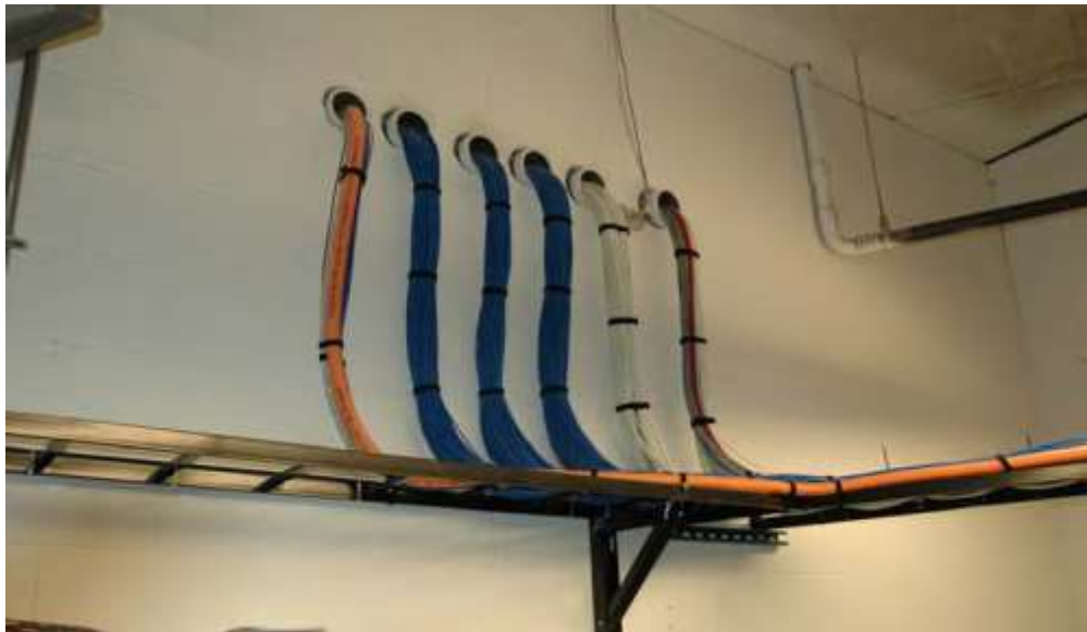
Figure 2 -- Typical Communications Room Cable Conduits
