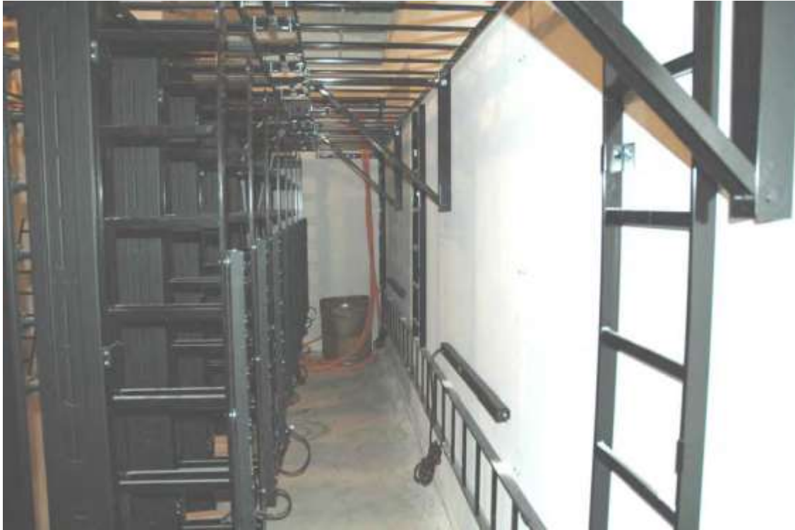
Figure 3 -- Typical Communications Room Overhead Cable Ladder and Backboard
