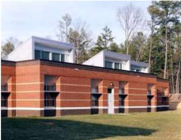
a) South-facing daylighting roof monitors
