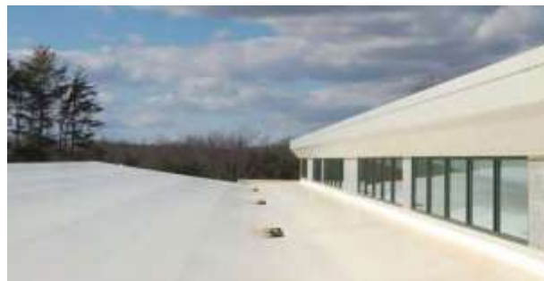
a) White roof in front of roof monitor windows reflects daylight deeper into the spaces.
