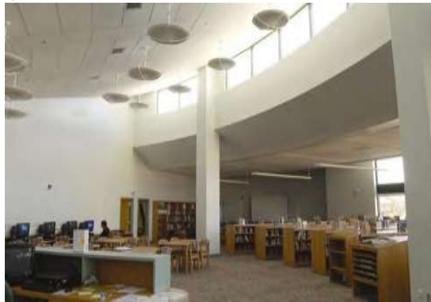
High north clerestories provide daylighting to a media center
