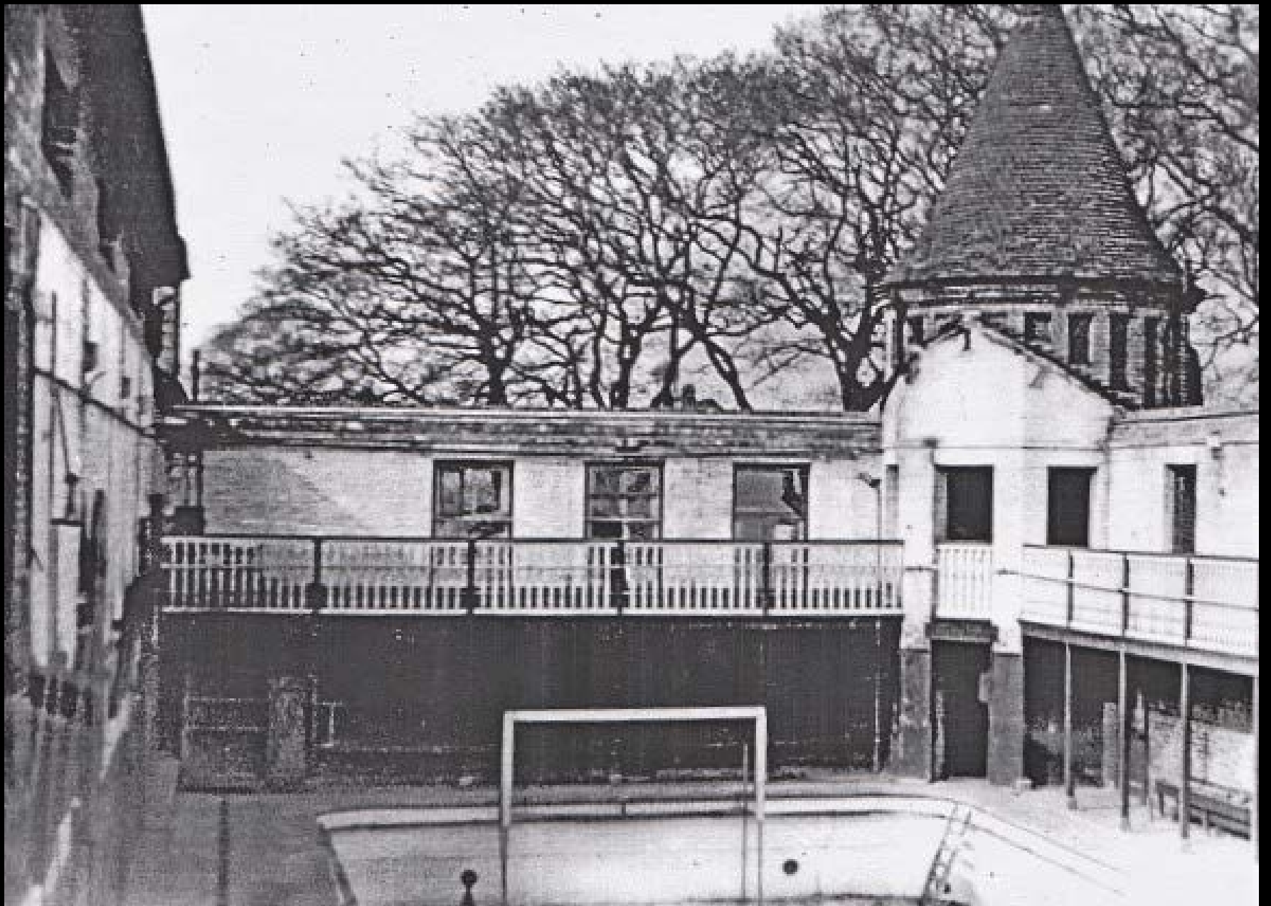
The old swimming pool roofless after bomb damage
