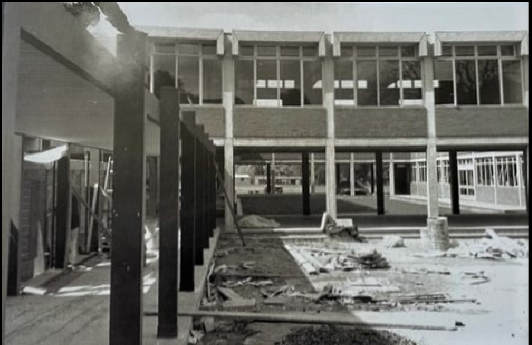
Christison Hall under construction
