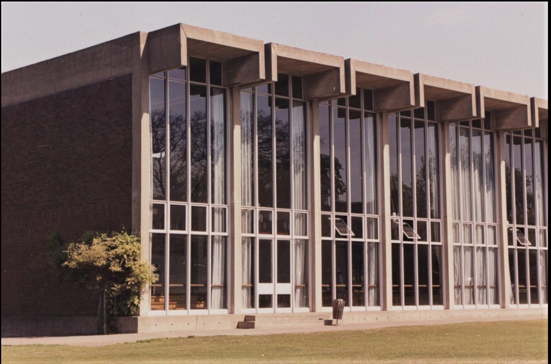
Christison Hall main elevation - 1970s
