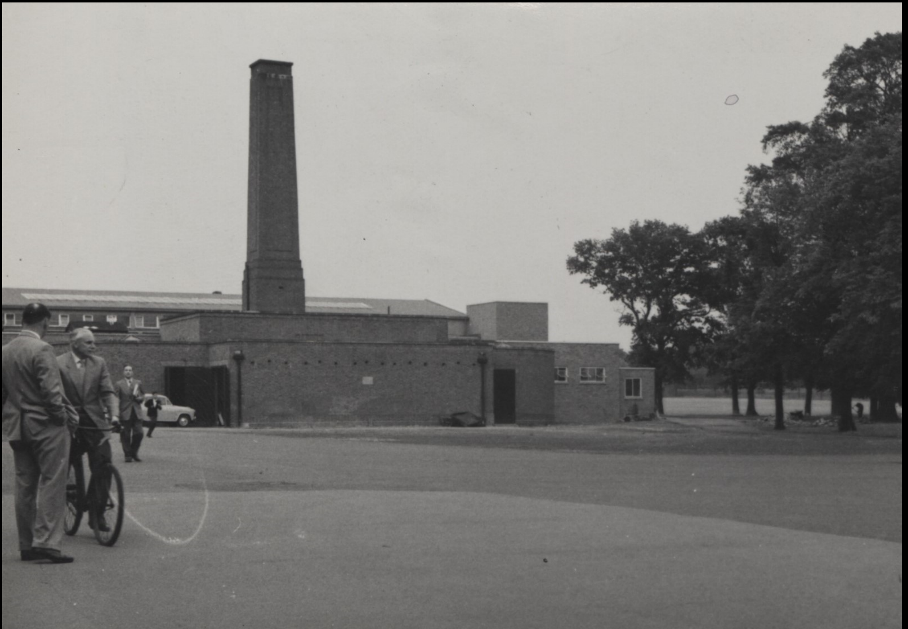
The squash Courts & the boiler house – built 1938-39
