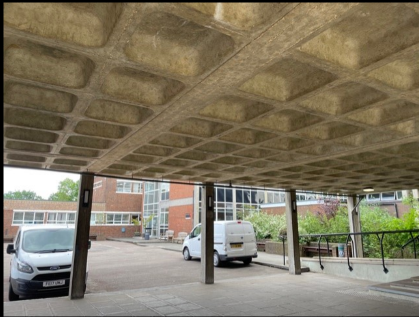
Christison Hall entrance area & main staircase - 2010
