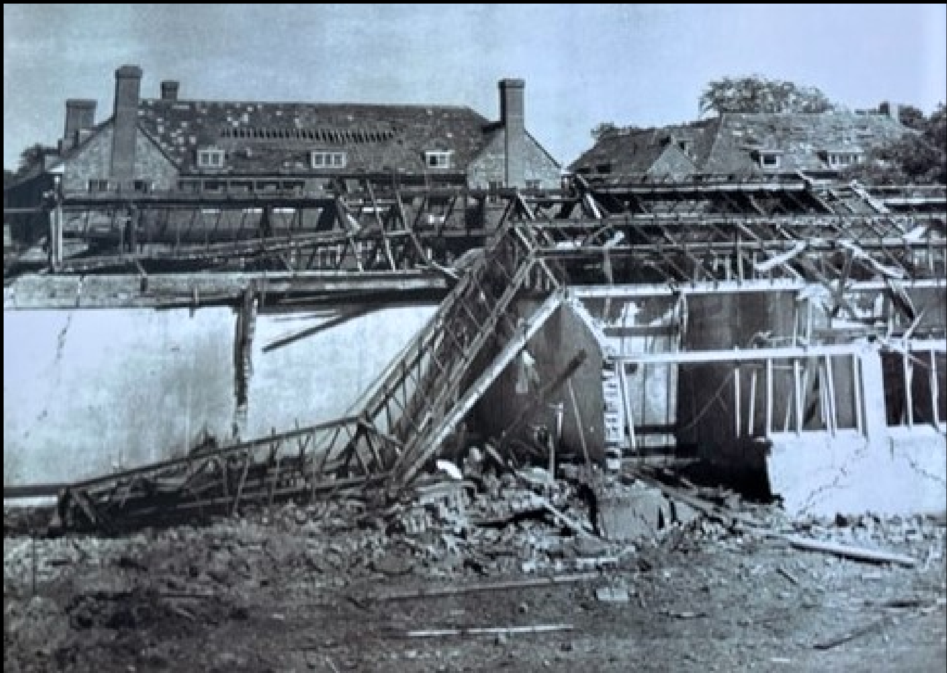
The old fives courts demolished after V1 bomb damage 10/07/1944
