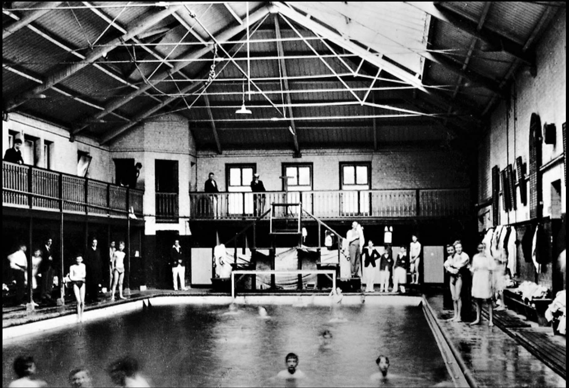
The old swimming pool interior
