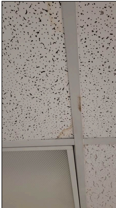
2 - View of water stained ceiling tile
