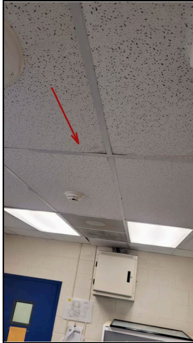
1 - View of water stained ceiling tile
