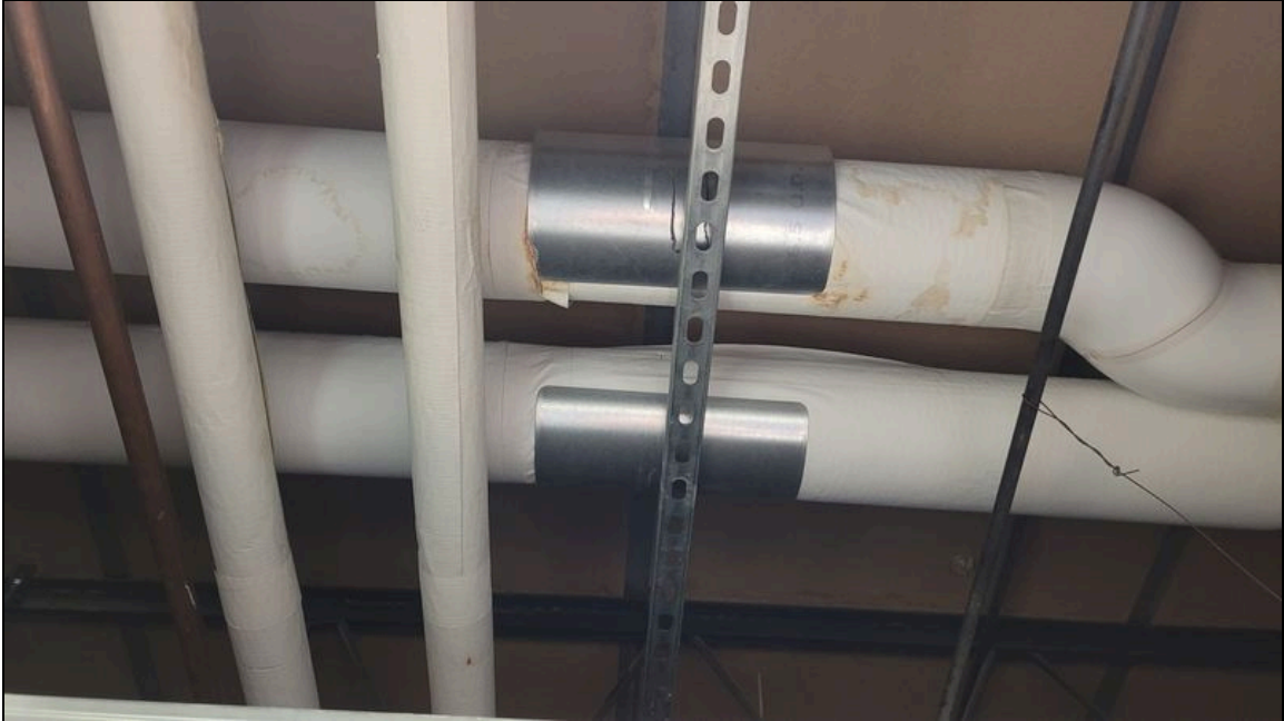
3 - View of water staining on pipes
