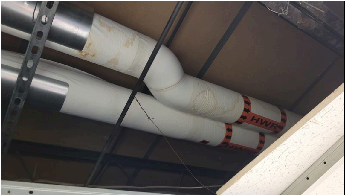
4 - View of water staining on pipes
