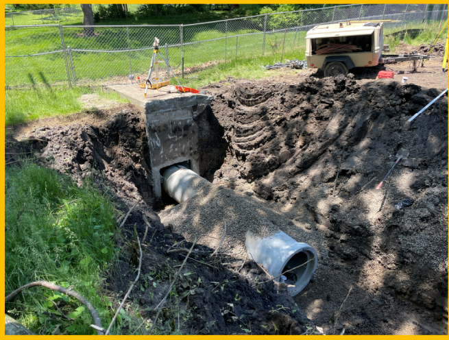
Continued Storm Sewer Install
