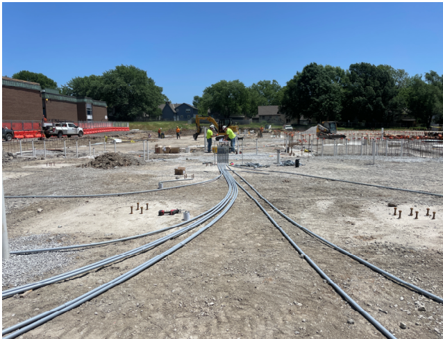
Plumbing & Electrical Underground
