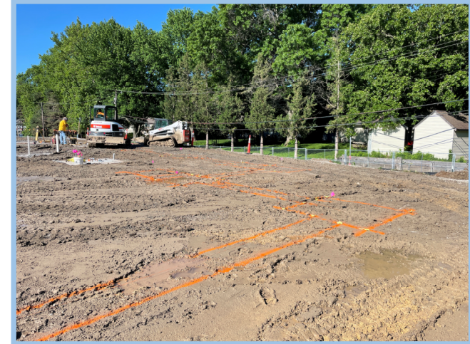
Continued Footing Layout and Excavation
