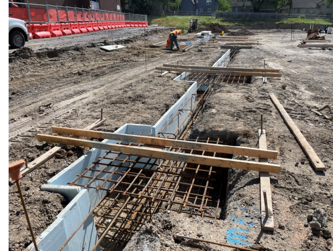
Continued Footing Formwork & Prep
