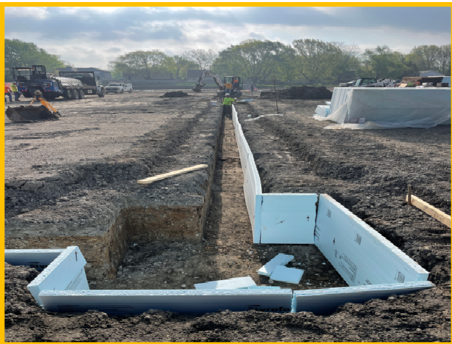
Foam Board Install
