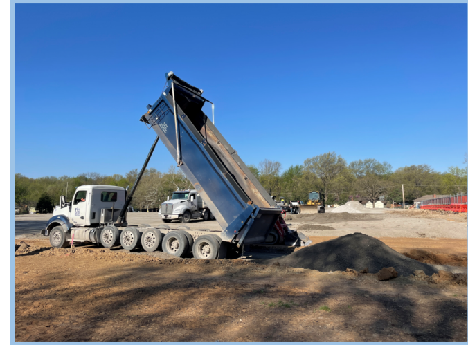
Raising Grade At Laydown Area
