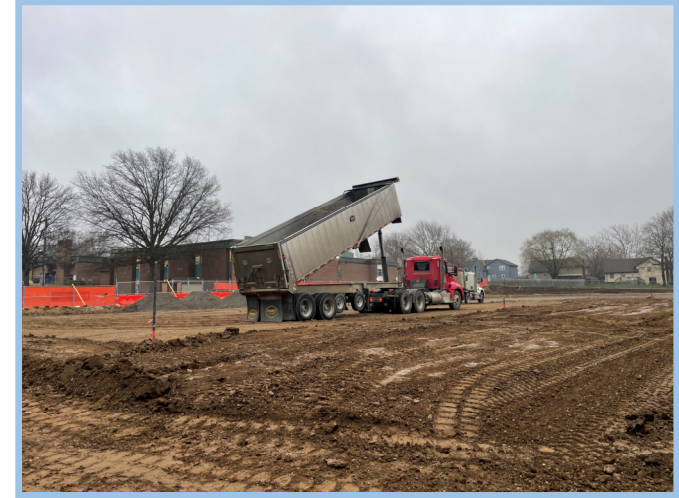
Imported Material For Building Pad
