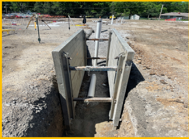
Plumbing Underground Sanitary
