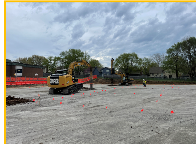
Completed Aggregate Piers
