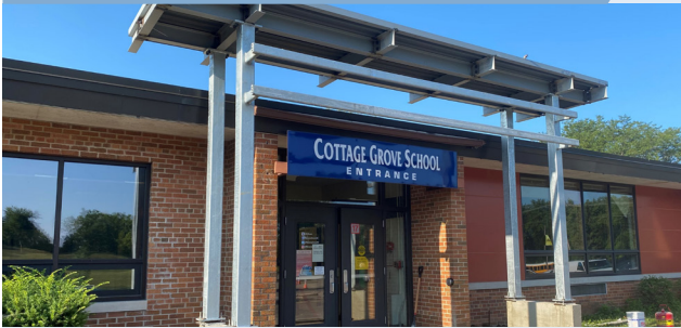
Renovations on track to be completed by the start of the 2021 school year.
