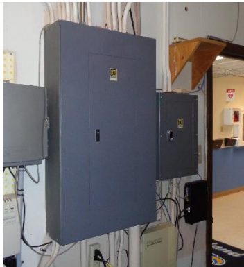
Figure 26: Square D Type NQOB in Storage/Lost and Found
