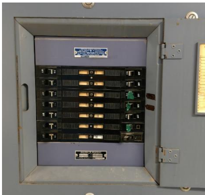
Figure 8: Existing Square D Type NQB Panelboard
