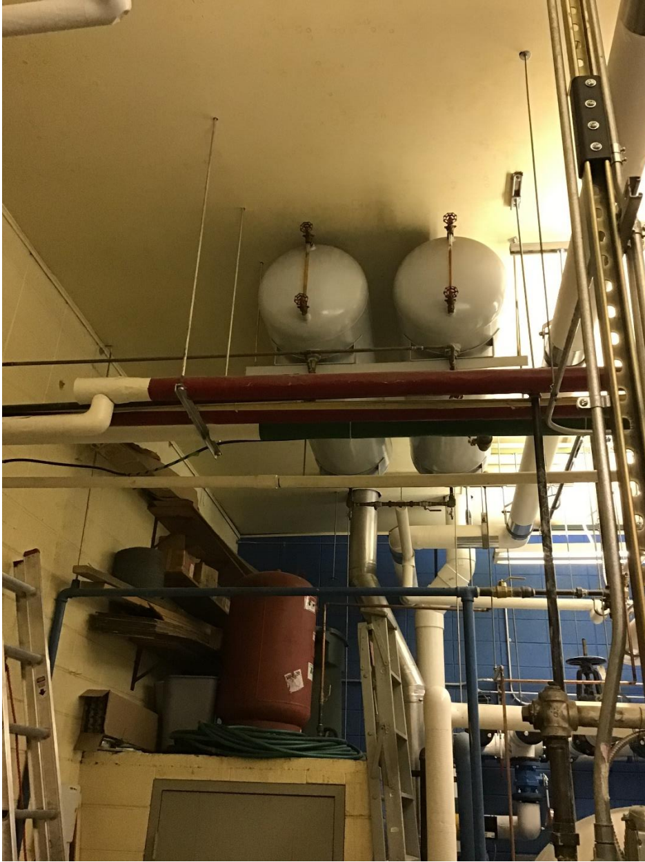
Baffle tanks and new expansion tank.
