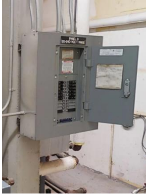
Figure 5: Existing Square D Type NQOD - Panel D
