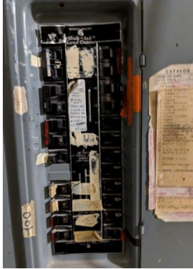
Figure 33: FPE Stab-lok® Panel near Auditorium (Interior)
