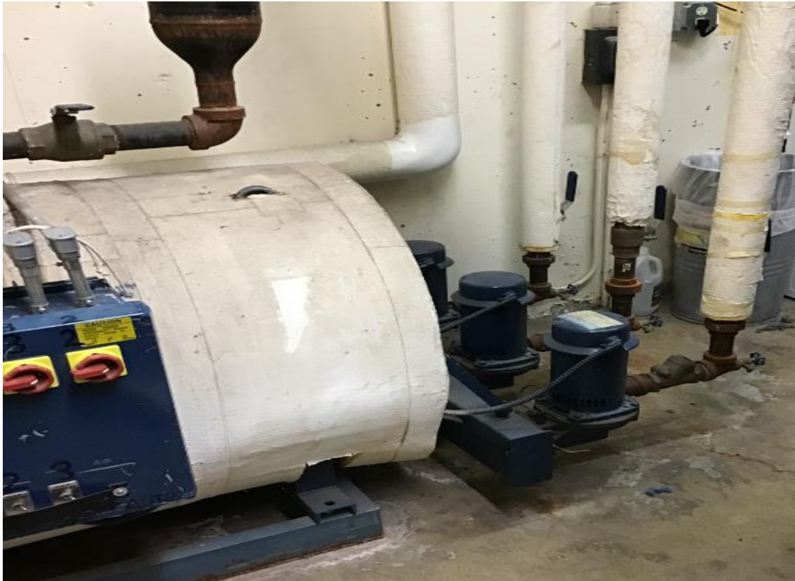
Condensate tank and pumps
