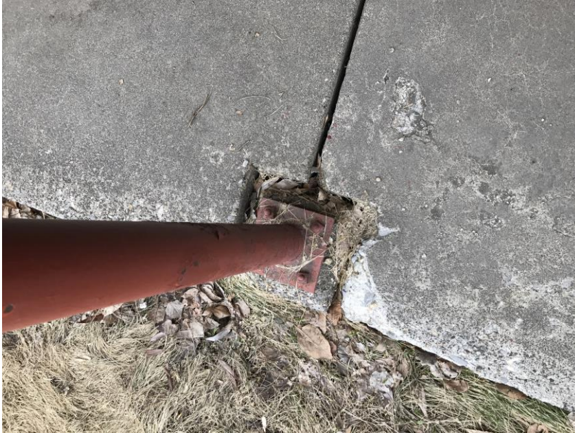
Column Base Deterioration
