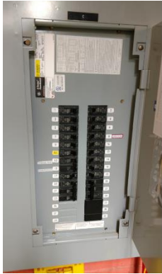
Figure 18: GE A-Series Panel C
