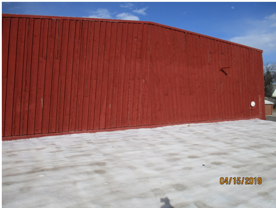
Overview of wood wall on the south side of the gym. Wall is taking on moisture.
