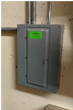
Figure 4: Square D Type QO Load Center
