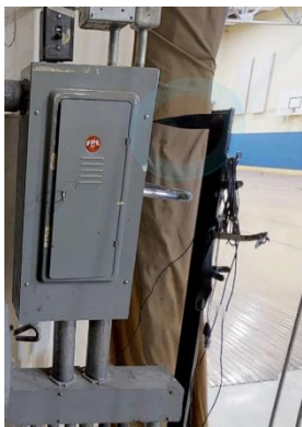
Figure 32: FPE Stab-lok® Panel near Auditorium
