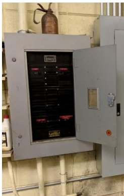
Figure 16: Westinghouse Type P-H Panel in Boiler Room
