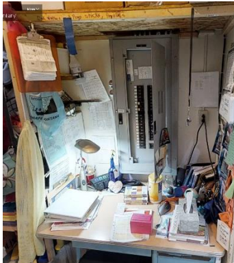
Figure 28: Desk Located in the NEC Required Working Space
