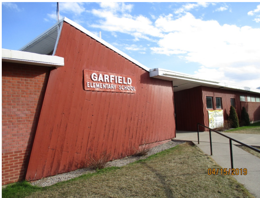
Overview of main entrance wood wall. Wood wall is taking on moisture.
