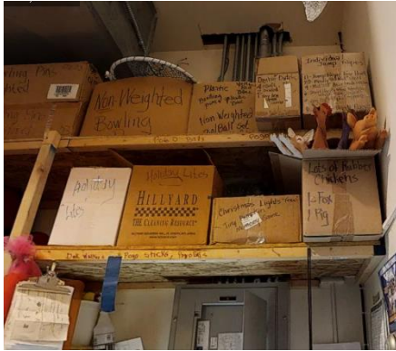
Figure 29: Shelving located in the NEC required Working Space
