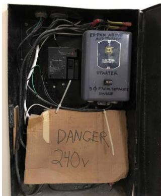
Figure 37: Starter Panel in Basement near Elevator (Interior)
