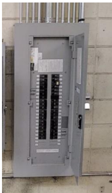
Figure 19: GE A-Series Panel M
