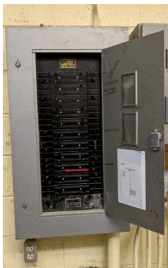
Figure 17: Westinghouse Type NLAB Panel in Boiler Room
