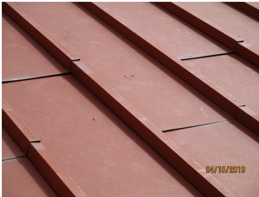
Ice damming backing up under seams and leaking into the building.
