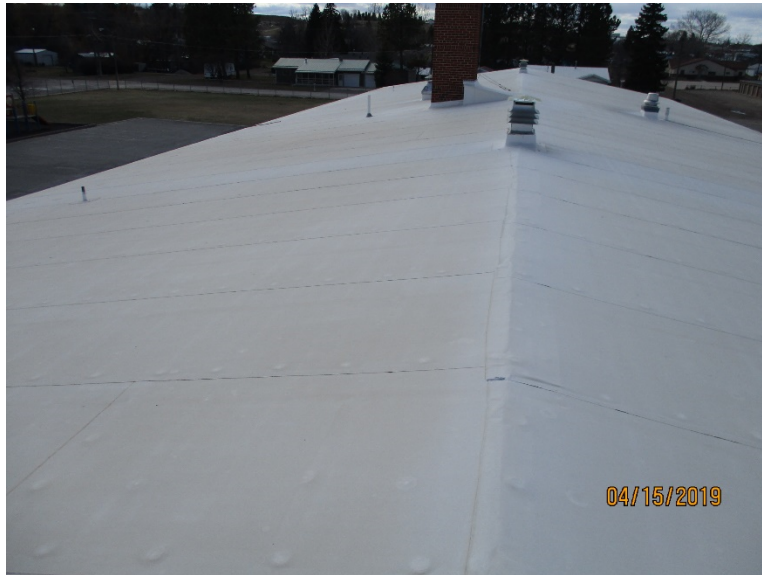
Overview of roof section 2 Hypalon roof.
