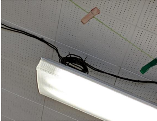
Figure 10: Example of Exposed Wiring
