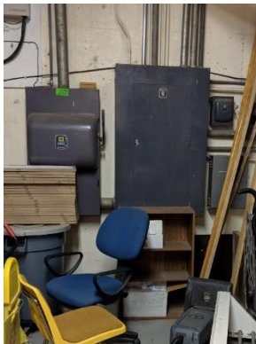
Figure 6: Existing Square D Type ML Panelboard
