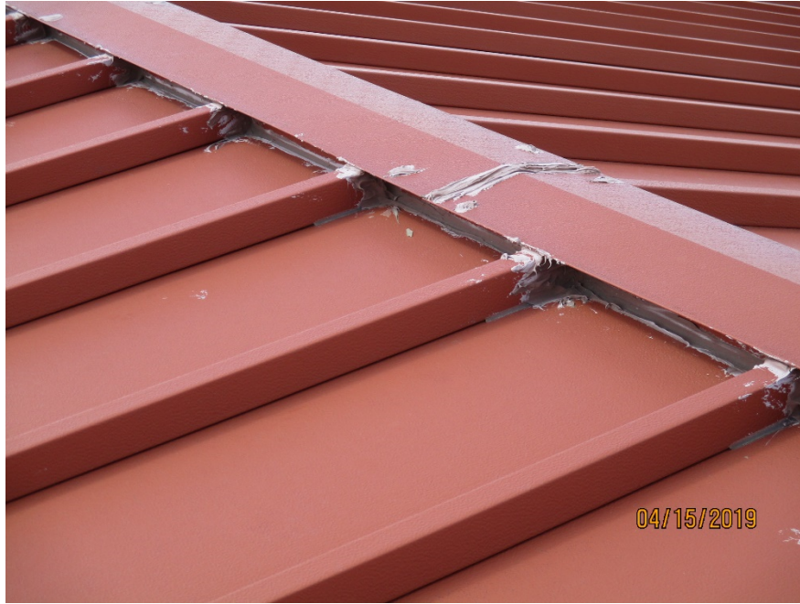
Sealant work at ridge in order to keep it dry.
