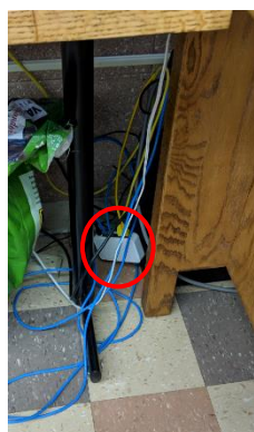
Figure 21: Ethernet Switch Used to Provide Additional Ports
