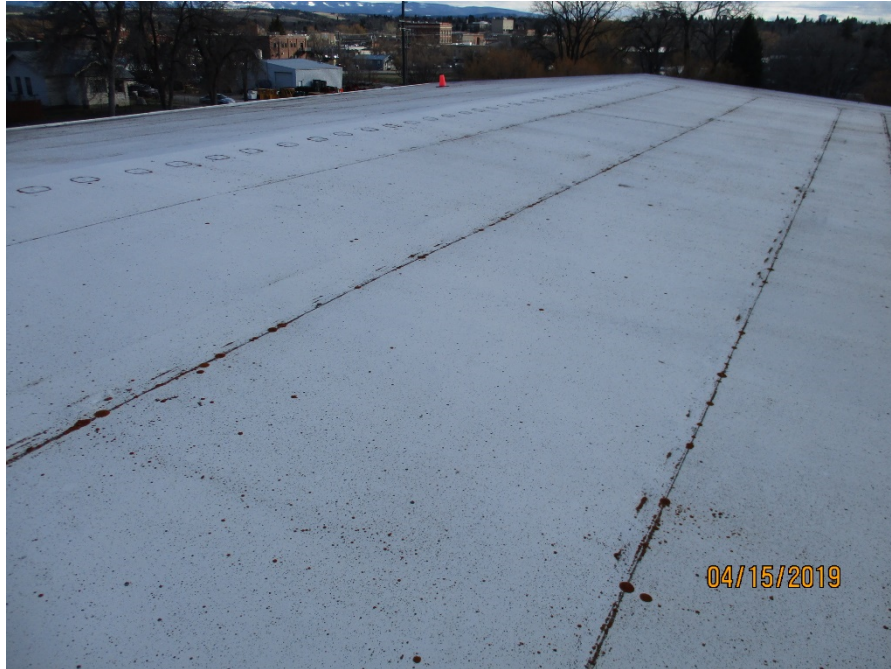
Overview of roof section 5. Single Ply Hypalon
