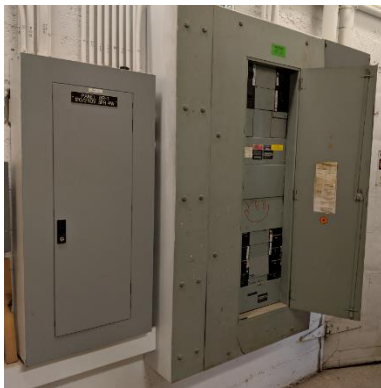
Figure 31: GE A-Series Panel (Left) and Westinghouse MDP
