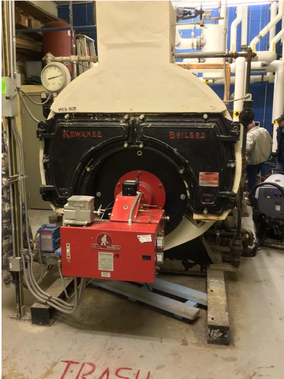
Existing back up boiler.
