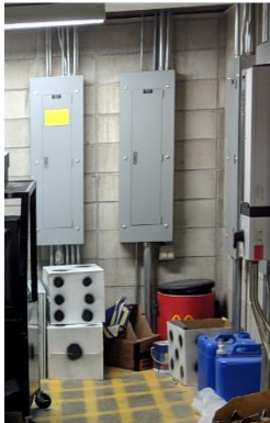
Figure 45: Typical GE NLAB Panels
