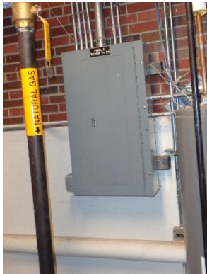
Figure 25: Square D Type NEQD Panel in Boiler Room
