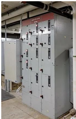
Figure 46: Typical GE 8000 Line MCC
