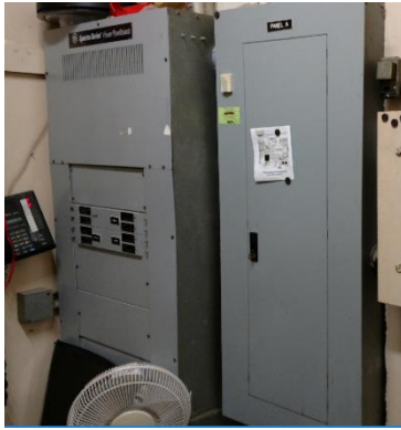
Figure 24: Spectra Series and A-Series Panels in Custodian Office
