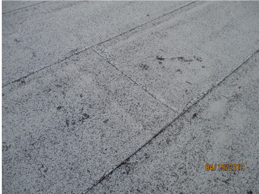
Hail damage is evident on roof surface.
