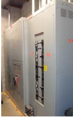
Figure 44: GE AV-Line Main Distribution Panel
