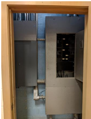
Figure 14: Square D Type NQOD (left) and Westinghouse MDP (right)
