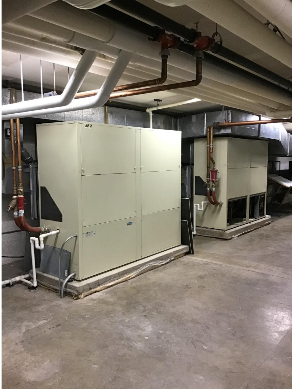
Water source heat pumps
