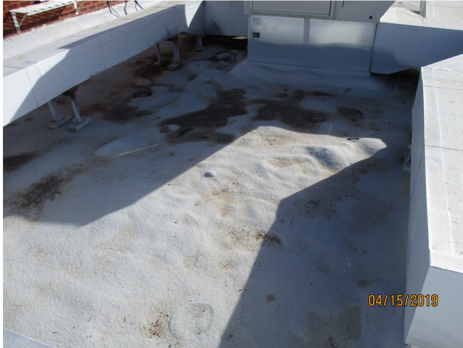
Foam blisters on roof section 4.
