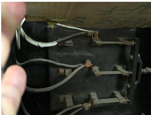
Figure 38: Knife Switches behind Cardboard
