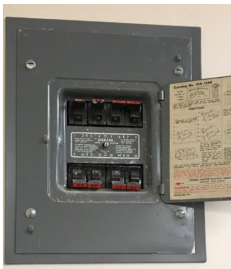
Figure 35: FPE Stab-lok® Panel in Basement near Elevator (Interior)
