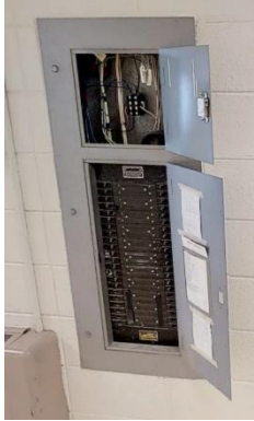
Figure 15: Westinghouse Type NLAB Panel in South Hall
