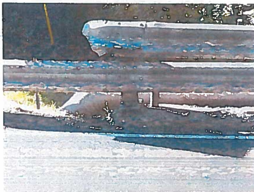
Collision damage at southeast MBR
