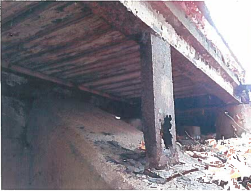
Deteriorated Sidewalk support
