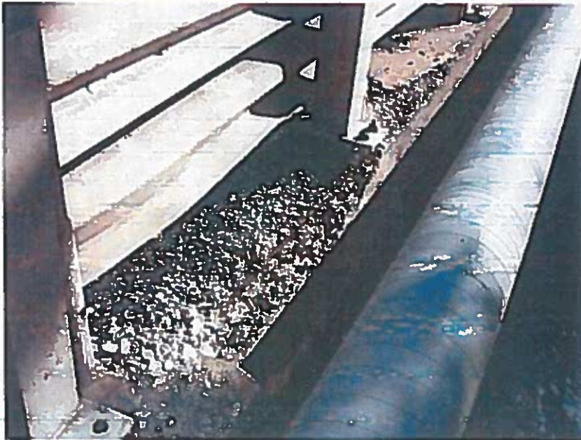
Severe scale on south railbase
