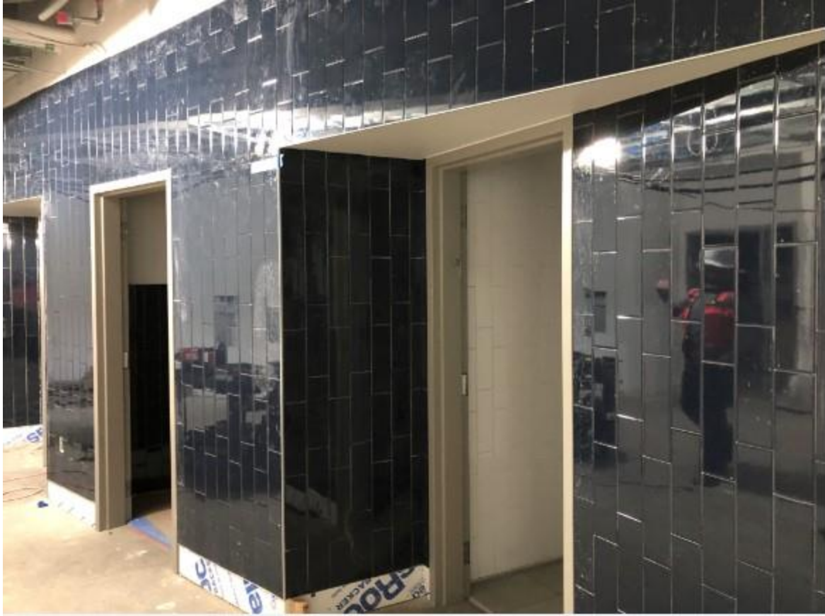
Tile installation on the first floor of the Academic Wing
