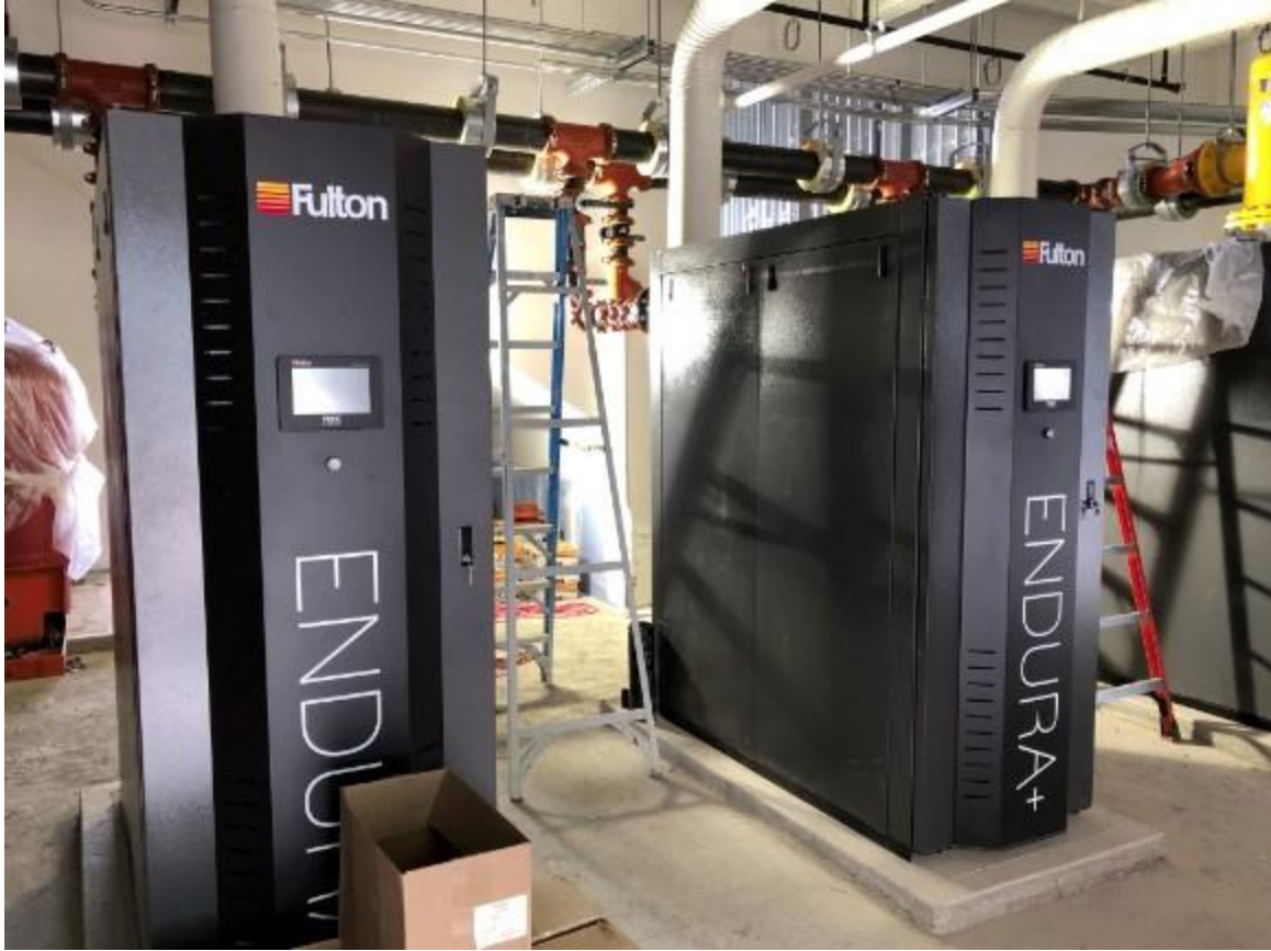
Boiler installation in the Academic Wing
