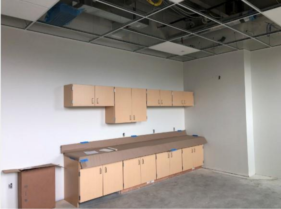
Cabinet installation in the Academic Wing
