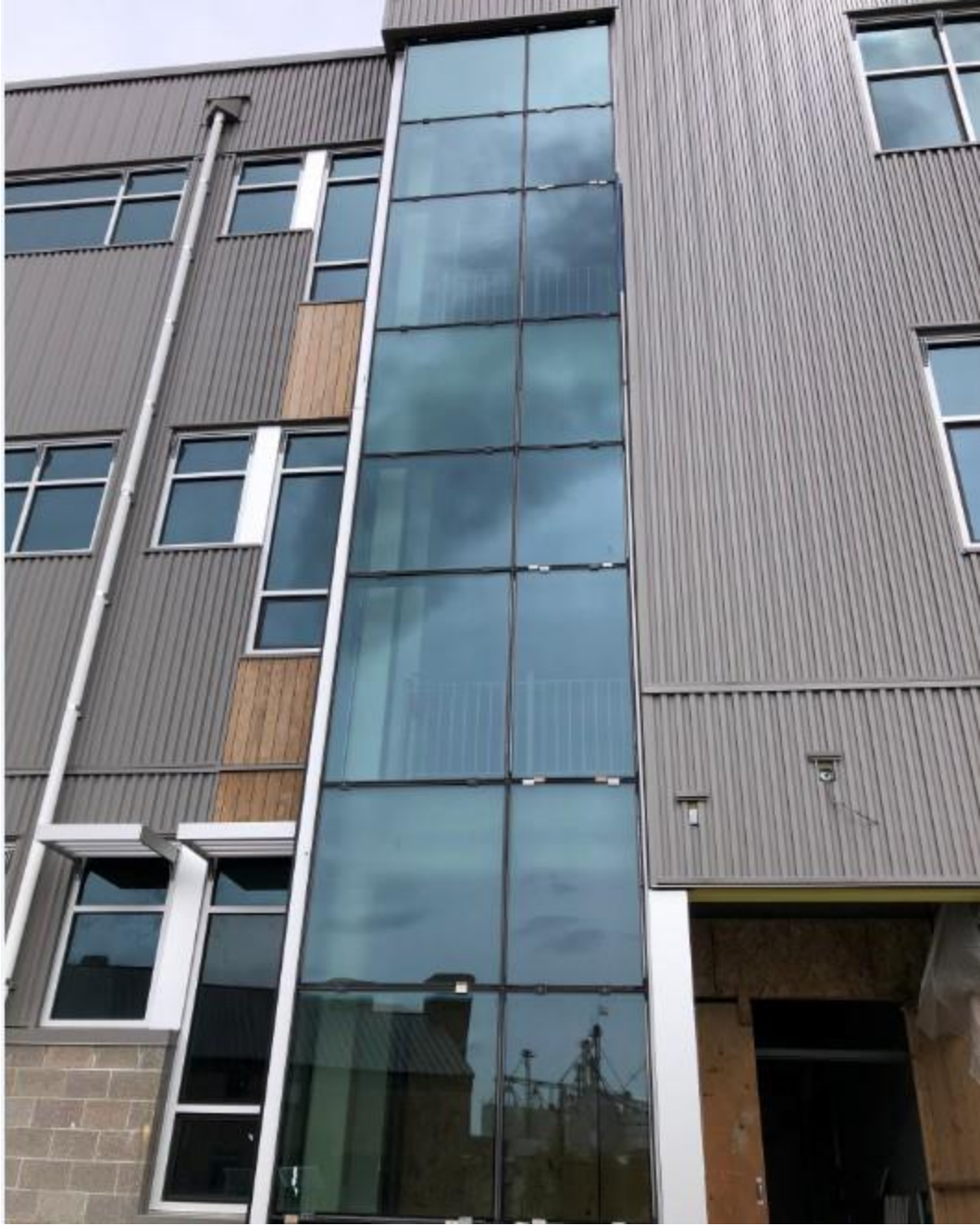
Glass installation on the exterior of the Academic Wing
