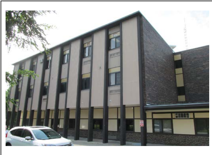
Photo 1- North Elevation of Existing High School
