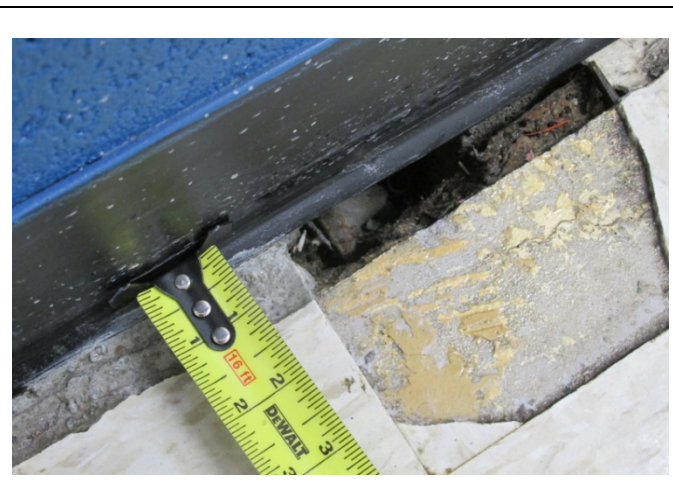
Photo 4 – Expansion joint between wall and floor (Enlarged)
