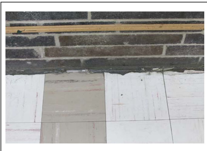
Photo 3 – Expansion joint between wall and floor
