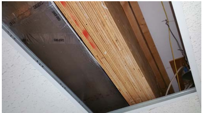
Photo 12 – Typical Modular Roof Framing
