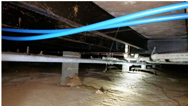
Photo 11 – Crawl Space Framing
