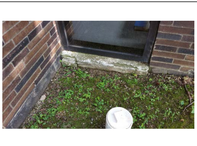
Photo 6 – General condition of exterior concrete
