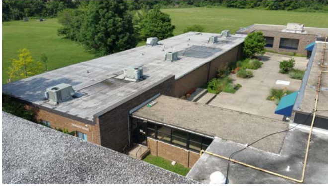
Photo 7- View of McKinney Middle School from High Roof
