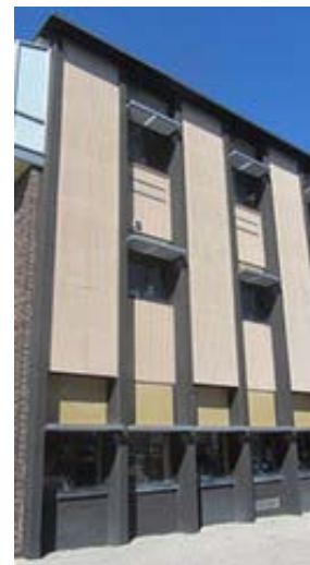
1963 Original Construction Three Story Structure
