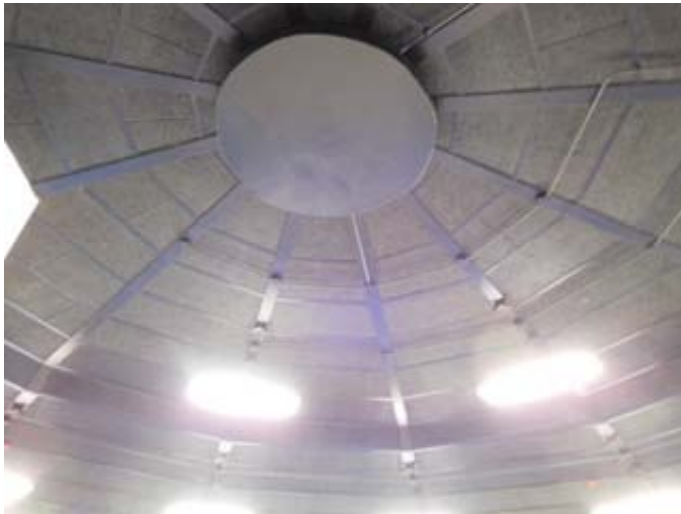
1963 Original Construction Music Room Roof Structure
