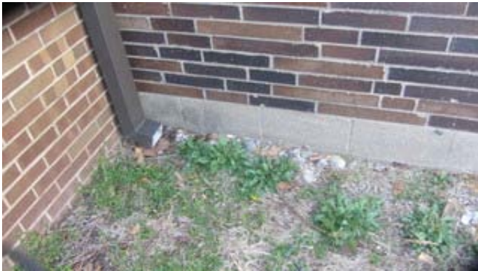
1963 Original Constructiton Exposed Foundation
