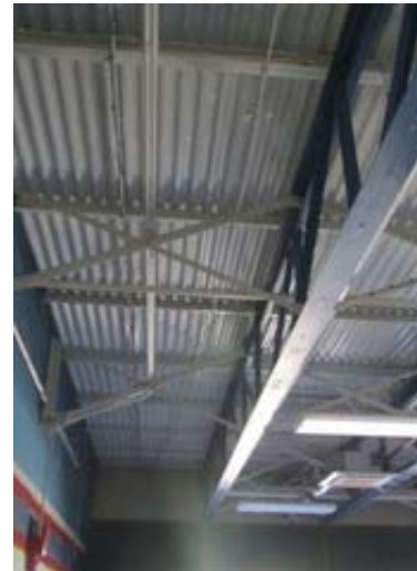
1963 Original Construction Student Dining Roof Structure
