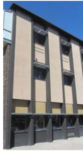
1963 Original Construction Classroom Windows
