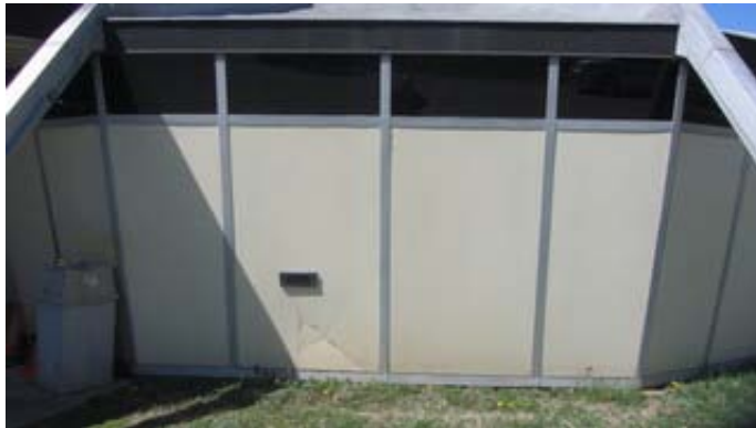
Insulated panels at 1963 Original Construction Music Room
