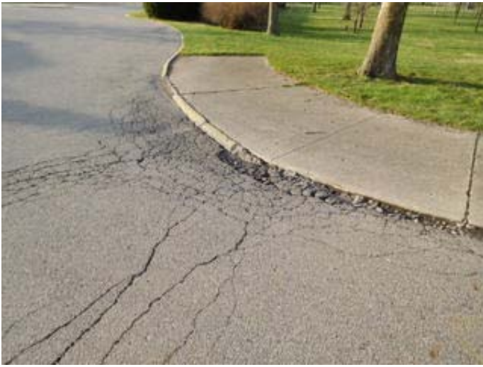
Asphalt, Curb, and Sidewalk Condition
