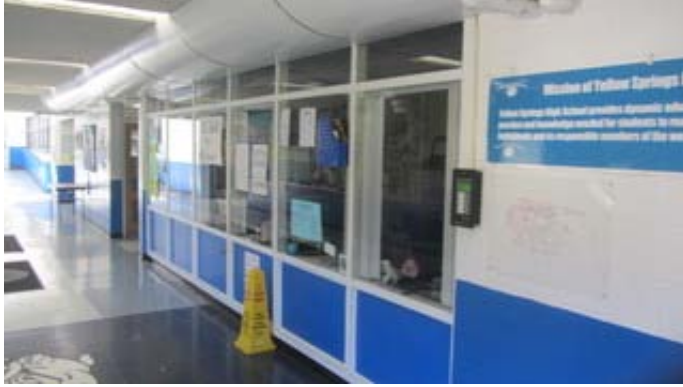
1963 Original Construction Interior Glazing
