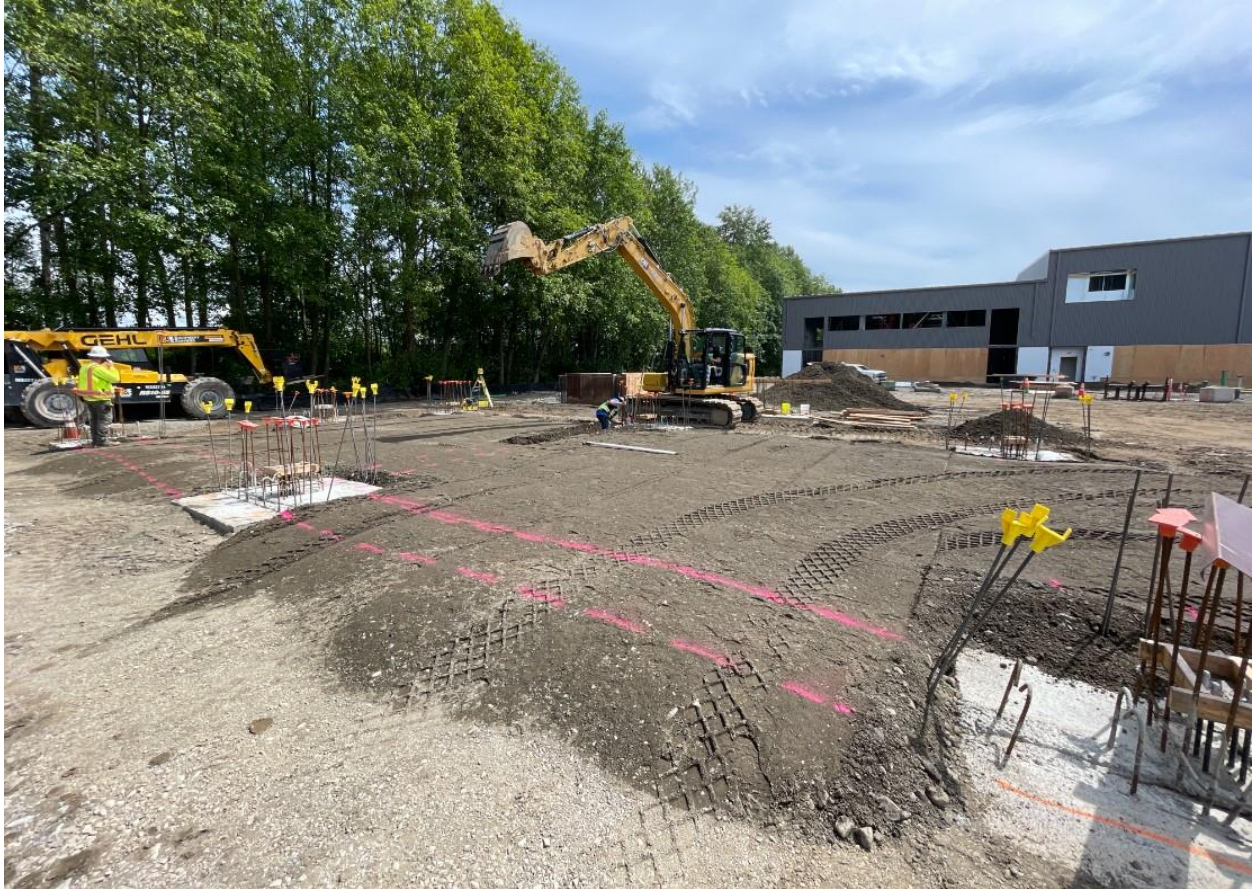
CTE Village foundations and groundwork moving along
