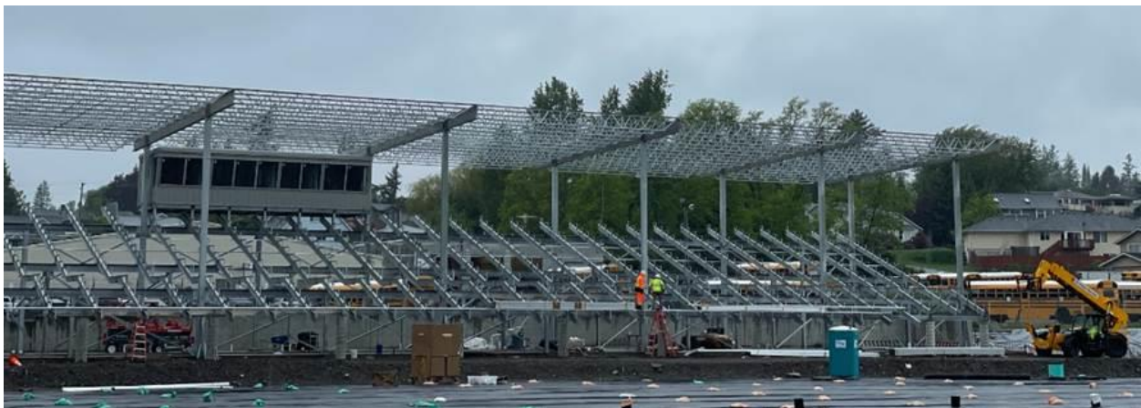
Grandstands making good progress
