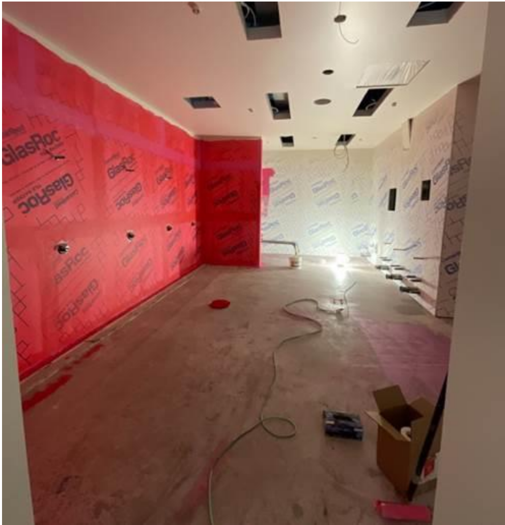
Main locker room bathrooms are just about ready for tile
