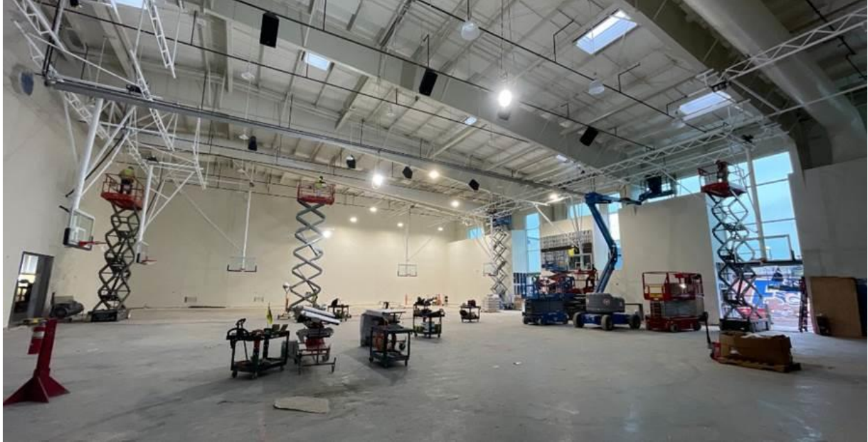
Basketball hoops and speakers being installed in Main Gym
