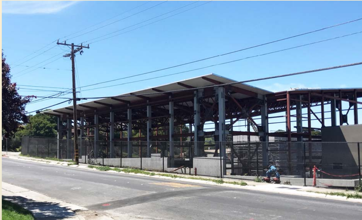
Gym Decking being Completed
