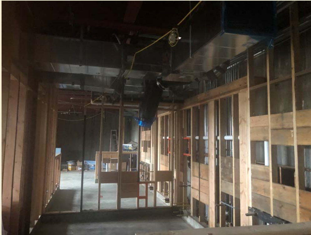
Framing of Locker Room Restrooms Completed
