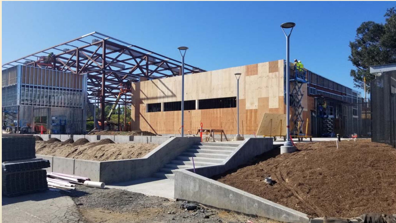
View from fire lane towards locker rooms and Gym
