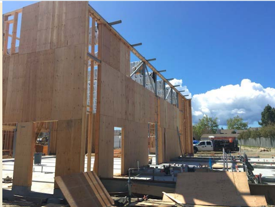
MPR Exterior Framing
