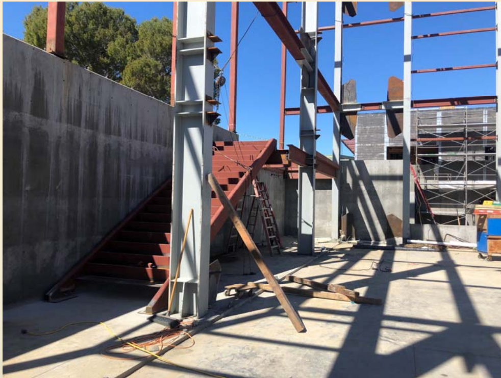
Steps being Installed to Parking Level from Gym
