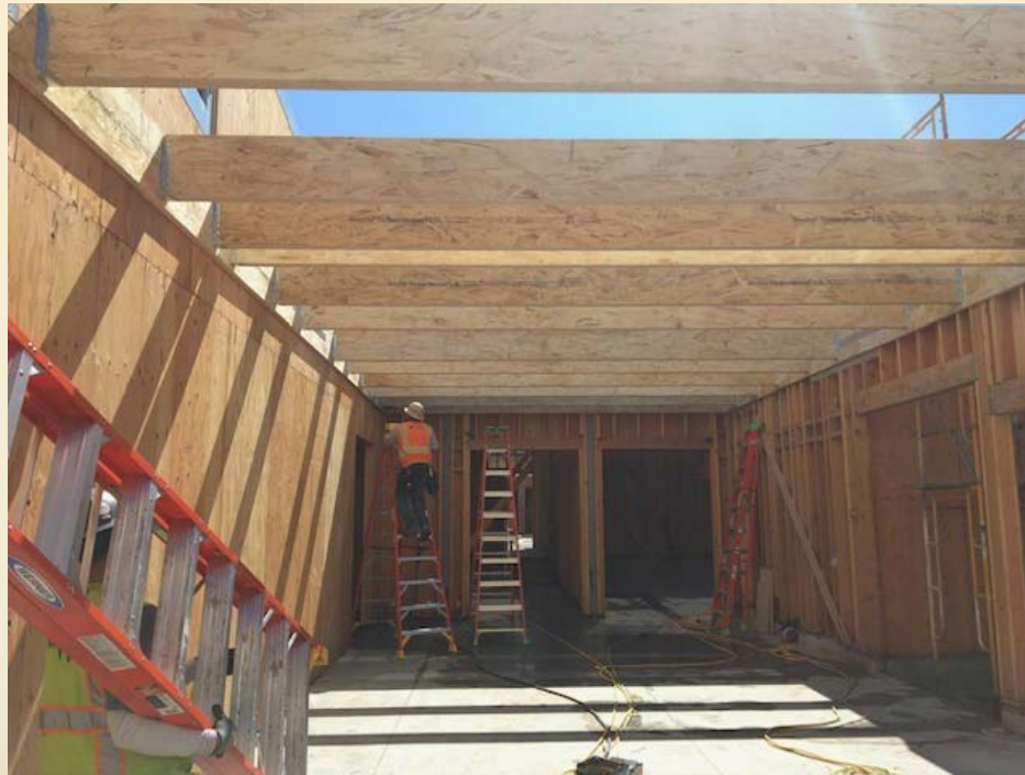
Installing Glue-Lam Beams
