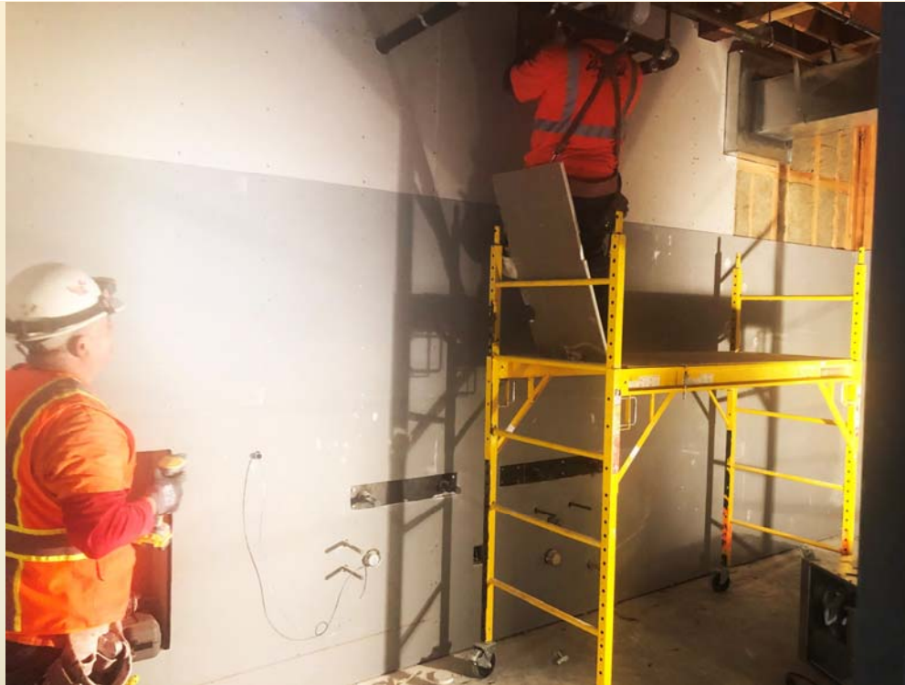
Dry wall being Installed in Gym Restrooms
