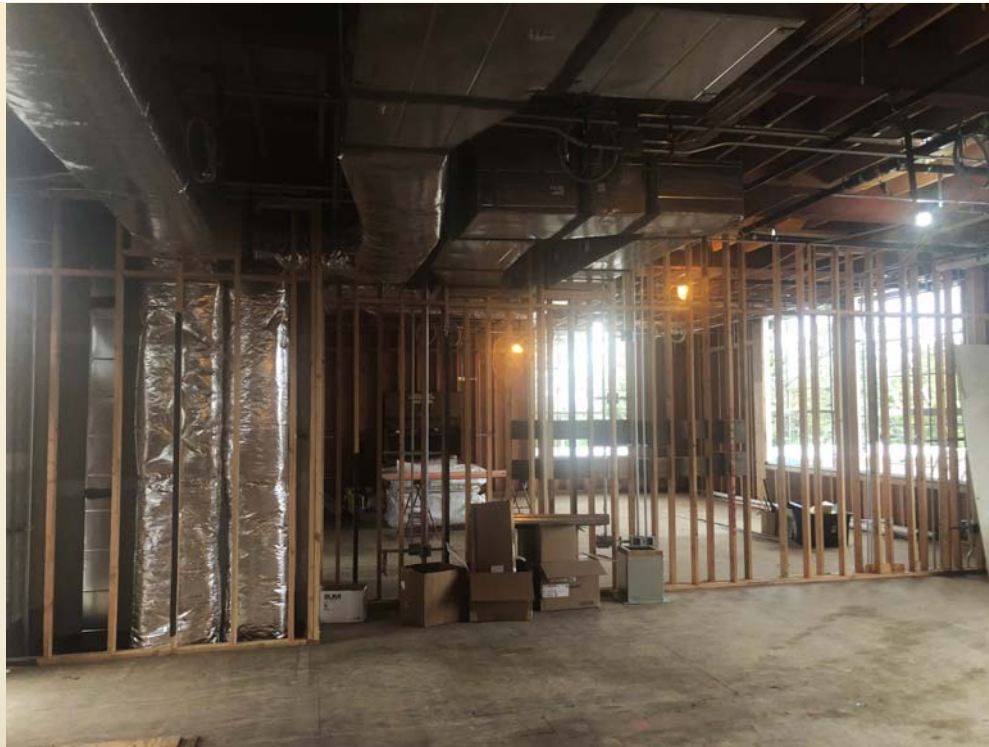
Classrooms Framing Completed
