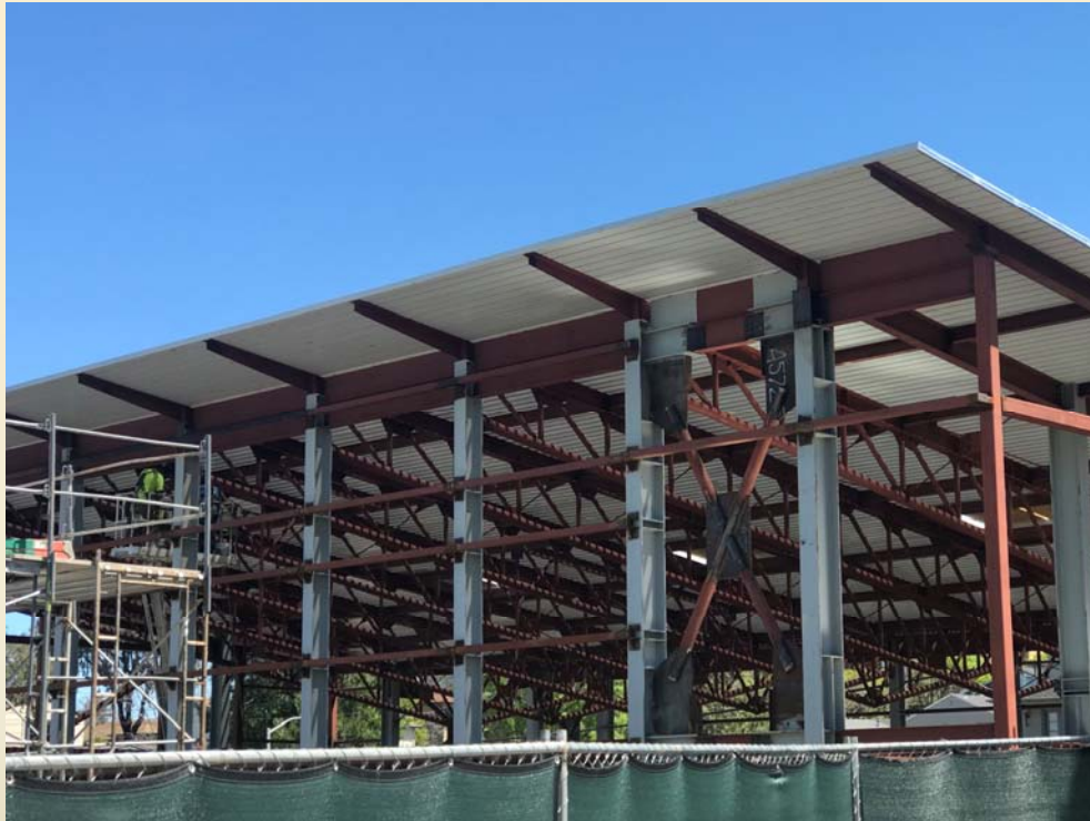
Brace Framing being Installed
