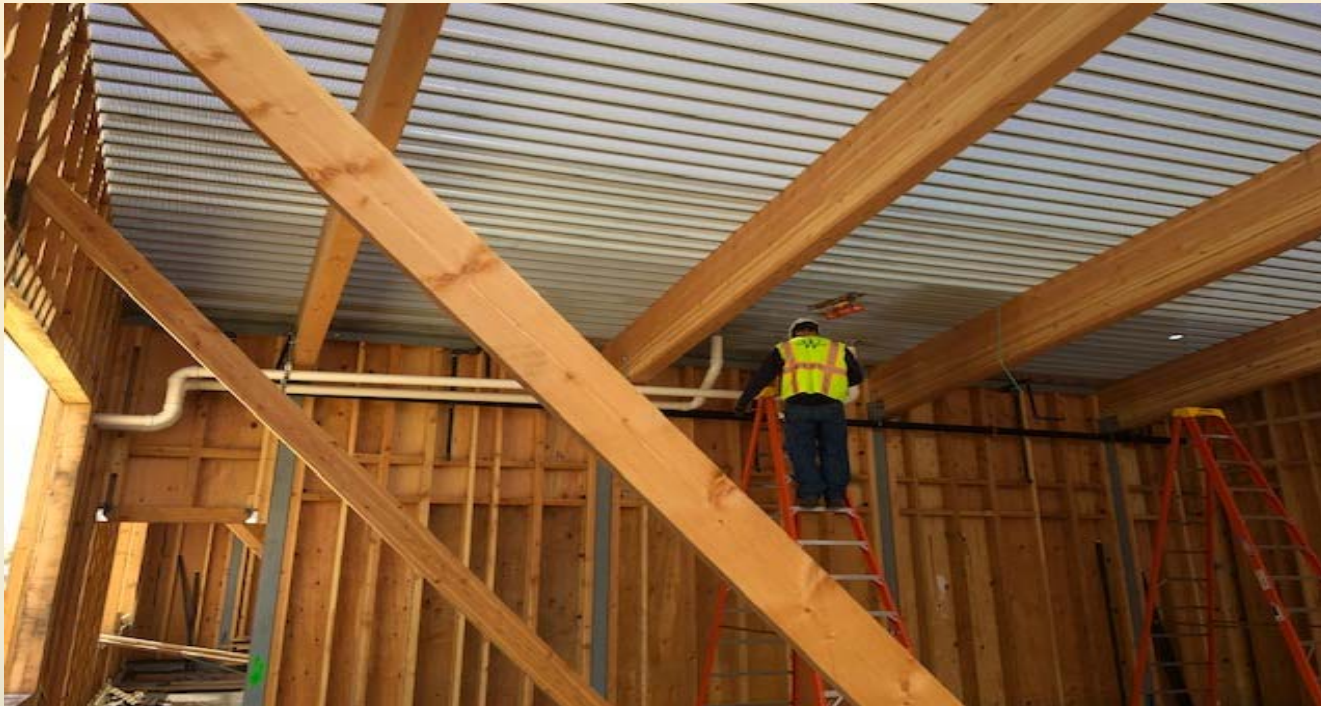
Installing Roof drains and Metal Decking
