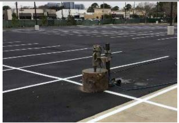
West parking lot being restriped.
