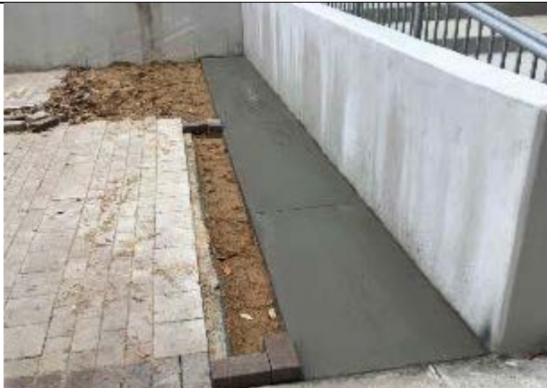
Auditorium Plaza paving work is ongoing
