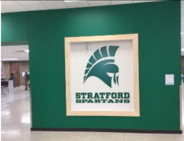
Logo installation at Cafeteria is near completion
