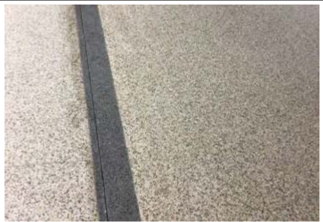
Terrazzo patching at Cafeteria.
