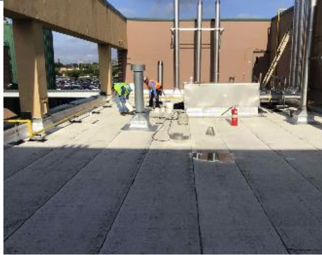
Roof work at existing side of campus.
