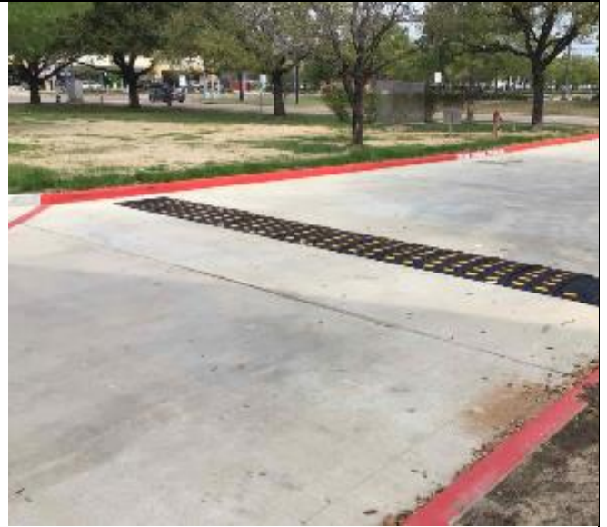
Speed bumps at West parking lot.
