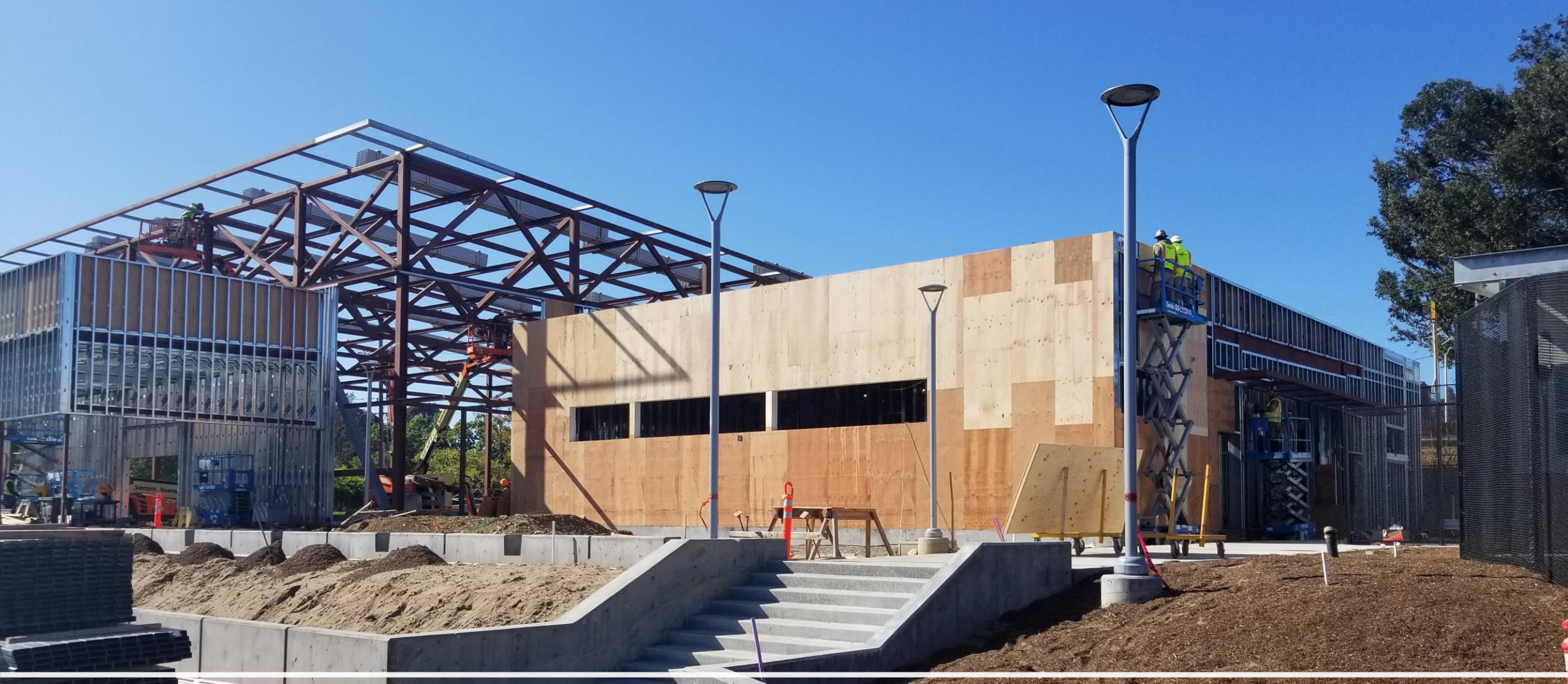
Borel—closer view of new locker room and restroom building
