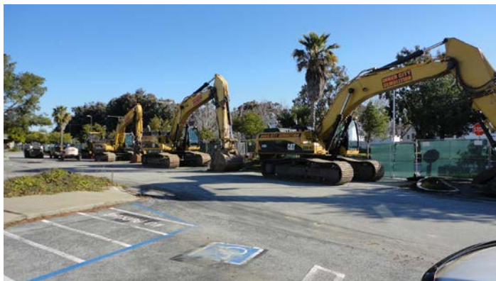
Former Charter Square Shopping Center Demolition
