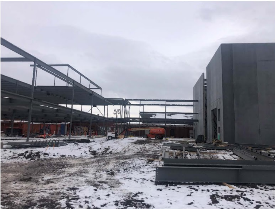
Fig 16: Steel Constructed Between Classroom Wing and Auditorium
