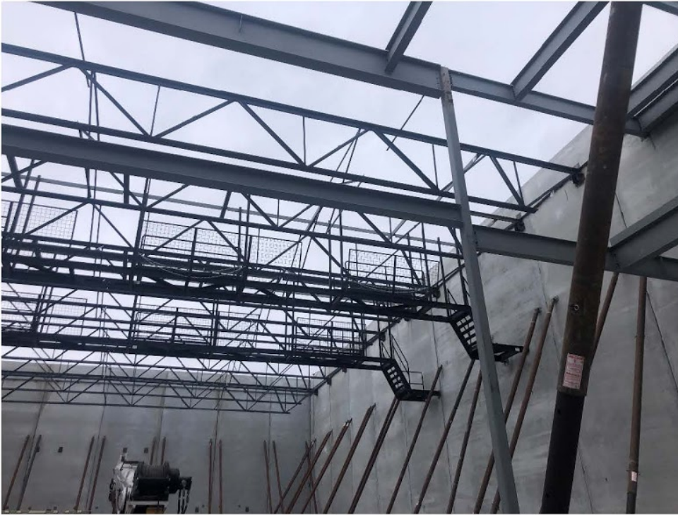
Fig 15: Auditorium Roof Joists and Catwalks
