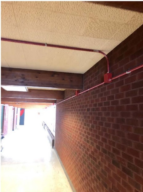
Fig 18: New Fire Alarm Installation at F-wing
