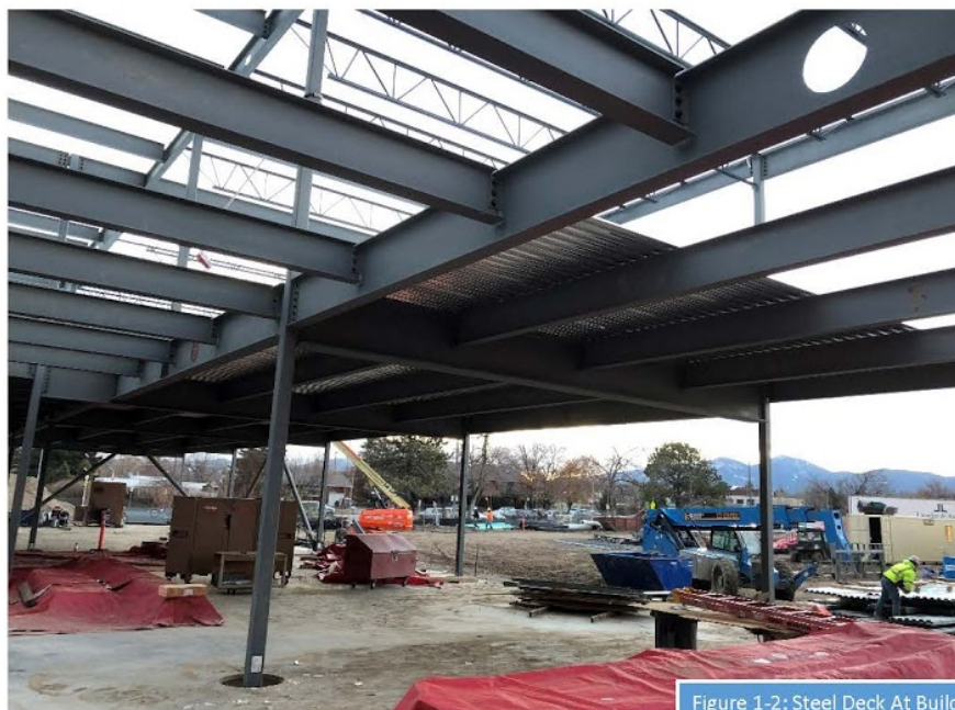
Figure 1-2: Steel Deck At Building 3B
