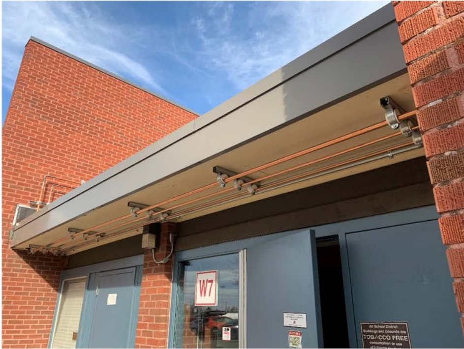
Figure 07: VRF piping for ACCU-5
