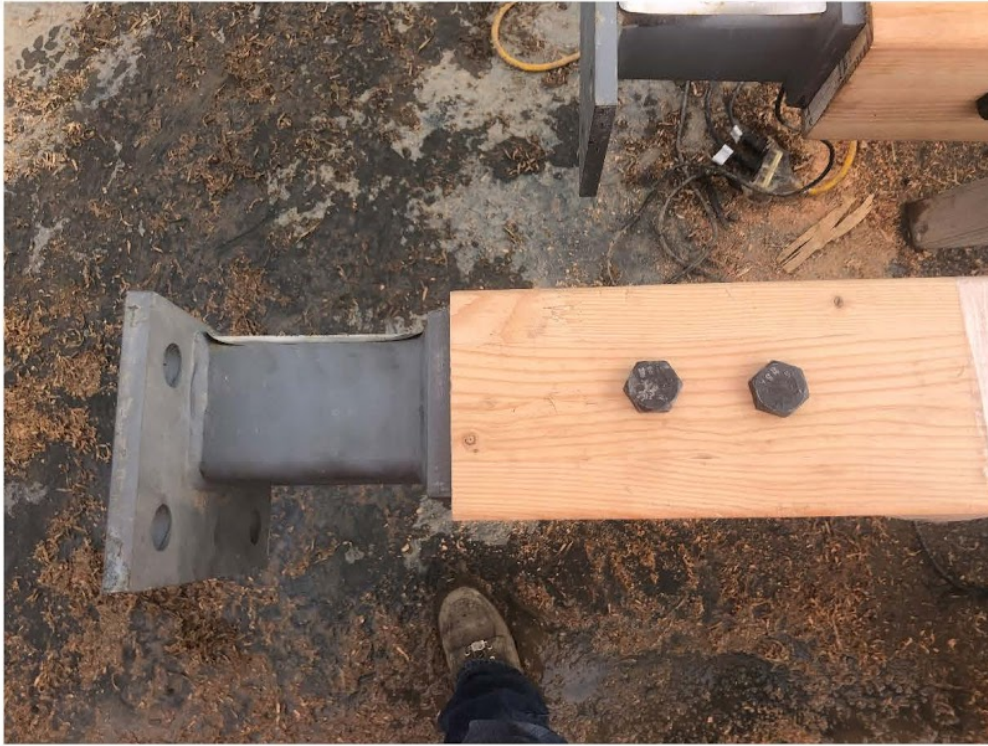
Fig 11: Glulam Column Bases
