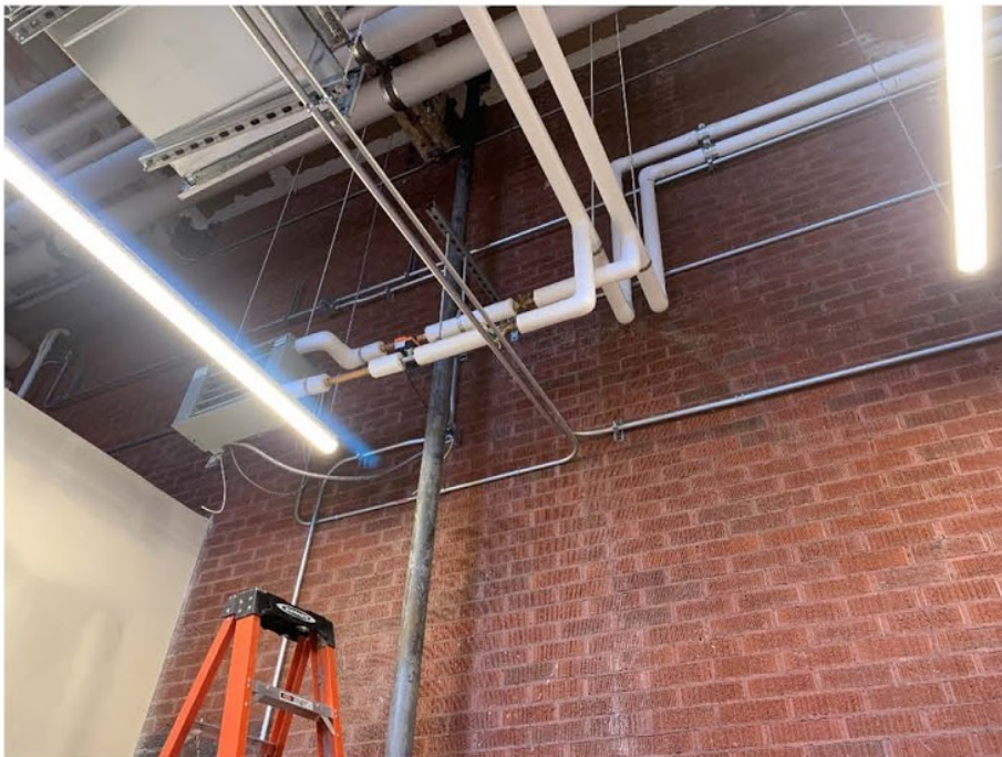
Figure 02: Hydronic Unit Heater installed in F-Wing Mechanical room.
