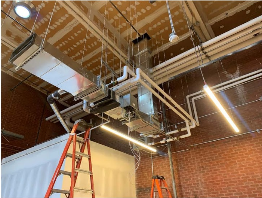
Figure 01: Blower Coil 2 Installed in F-Wing Mechanical room.
