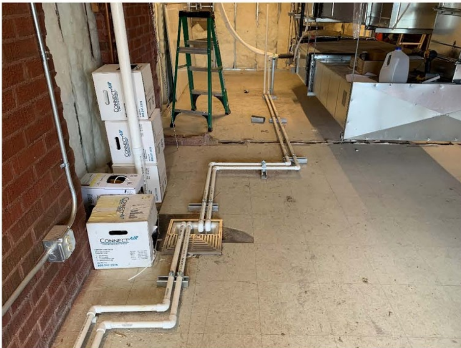
Figure 04: Condensate piping for FCU-F18 and F19.
