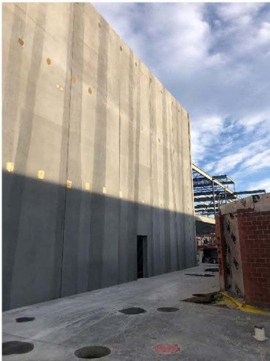
Fig 10: Precast Concrete Panels
