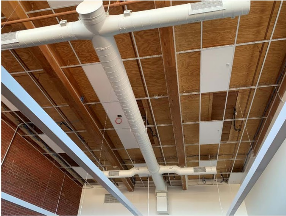
Figure 03: Ductwork painted in F-19 Classroom.
