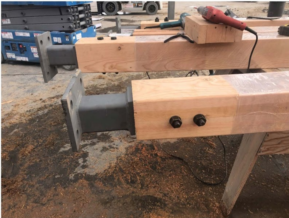
Fig 12: Glulam Column Bases
