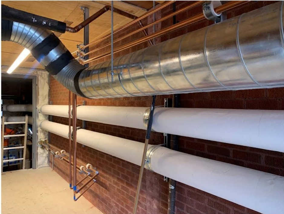
Figure 05: Refrigeration Piping in the mechanical mezzanine
