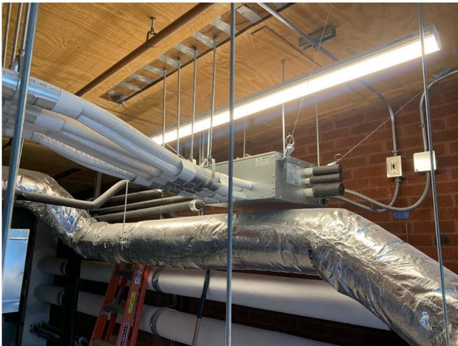
Figure 04: Heat Recovery Box installed in Mechanical Mezzanine. VRF pipe supported.
