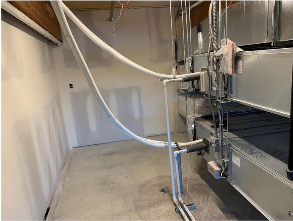
Figure 05: Fan coil installation in mechanical mezzanine.
