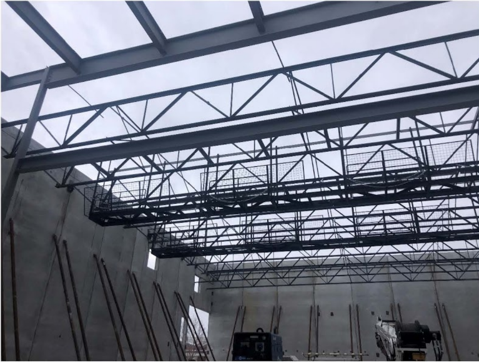
Fig 13: Auditorium Roof Joists and Catwalks
