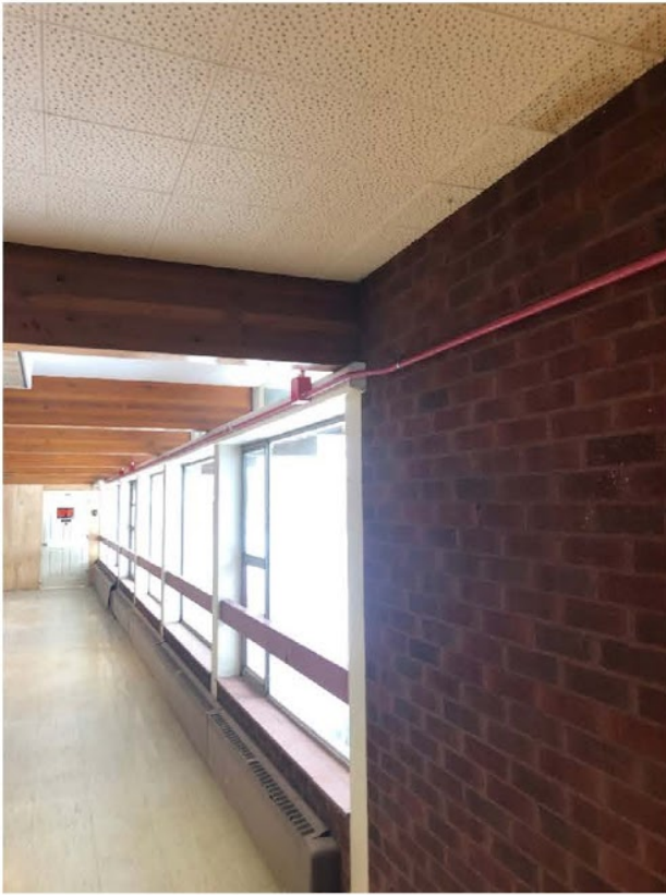
Fig 19: New Fire Alarm Installation at F-wing
