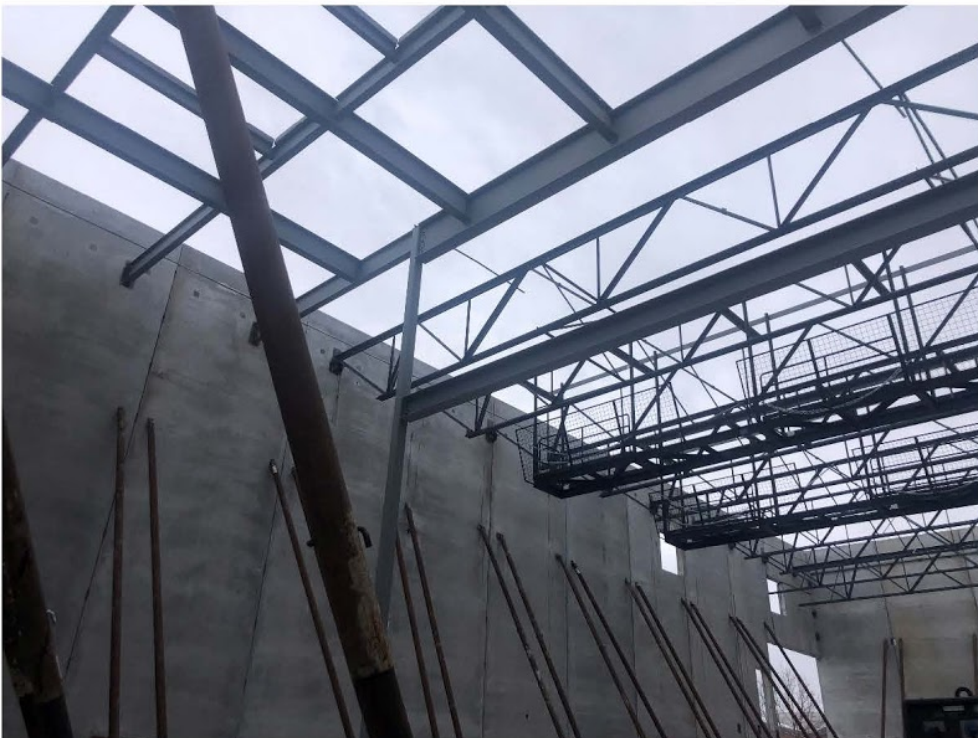
Fig 14: Auditorium Roof Joists and Catwalks
