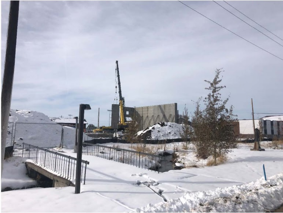
Fig 08: Erection of Precast Panels
