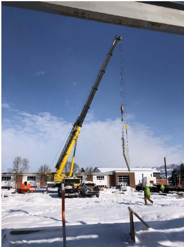
Fig 07: Erection of Precast Panels
