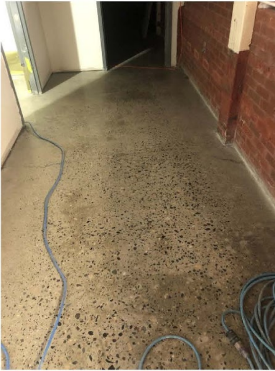
Fig 14: Concrete Polishing at F-wing Classrooms
