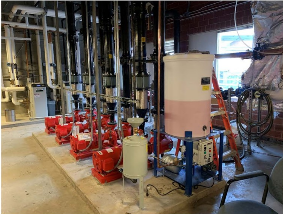
Figure 05: Hydronic Pumps and Glycol feeder installed in Mech H-3.
