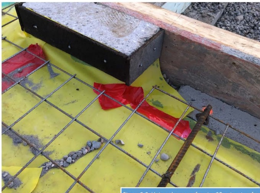
Figure 3-2: Untaped corner of easter 3B entry storefront had been taped
