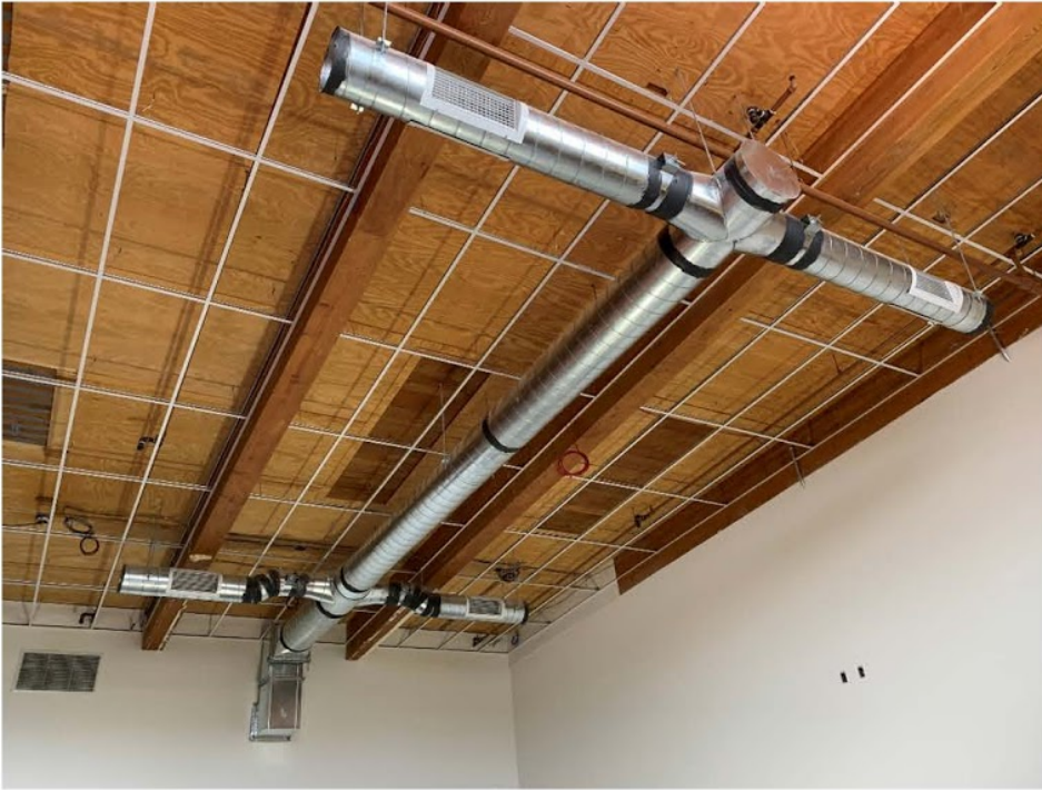
Figure 03: Ductwork installed in F-Wing Classroom.
