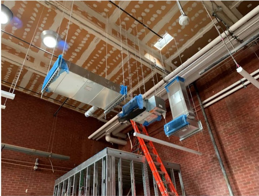
Figure 01: Blower Coil 2 Installed in F-Wing Mechanical room.
