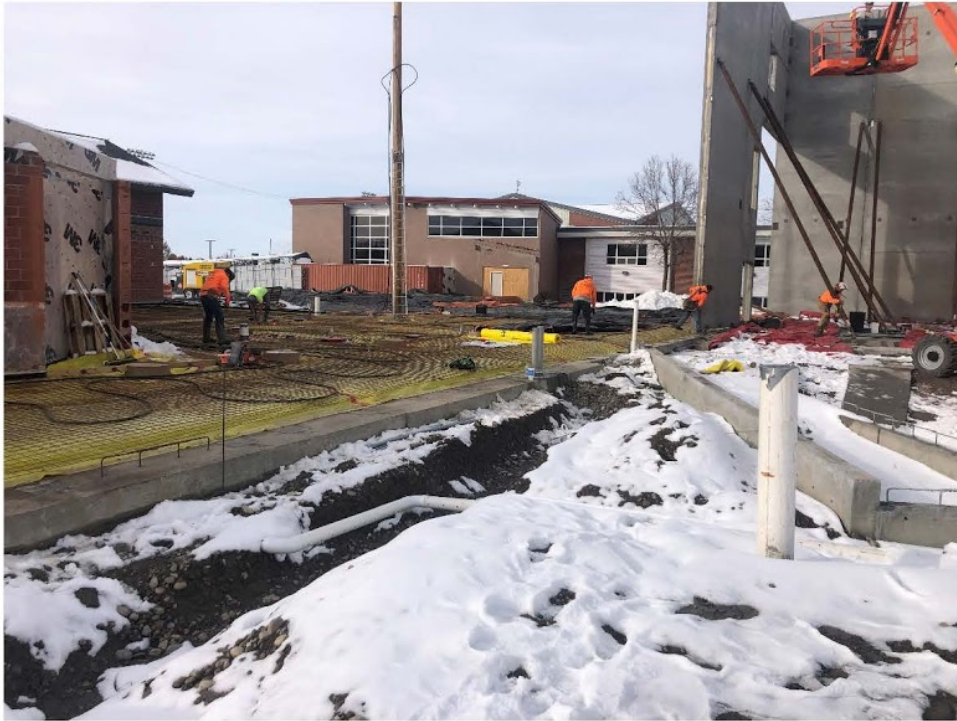
Fig 09: Underslab Preparation Work
