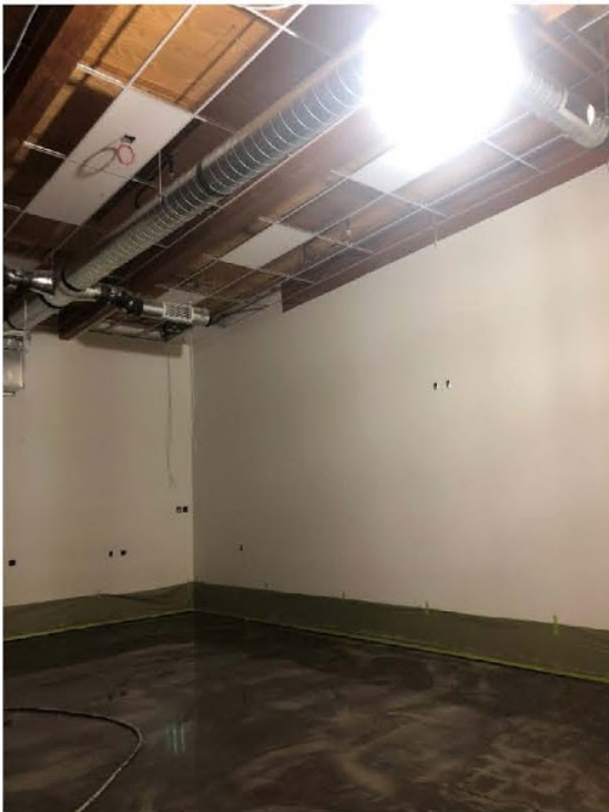
Fig 15: Ceiling Installation and Concrete Polishing at F-wing Classrooms
