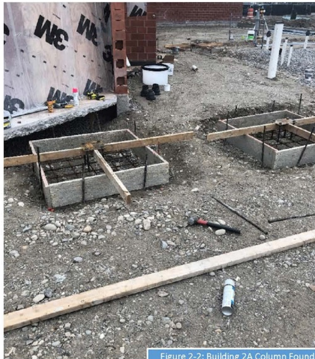
Figure 2-2: Building 2A Column Foundation Formwork
