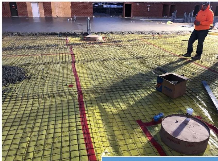
Figure 4-2: Pedestals were installed as pour progressed
