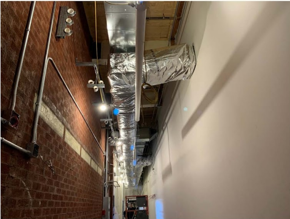
Figure 04: Insulated Ductwork installed in F-Wing Corridor.
