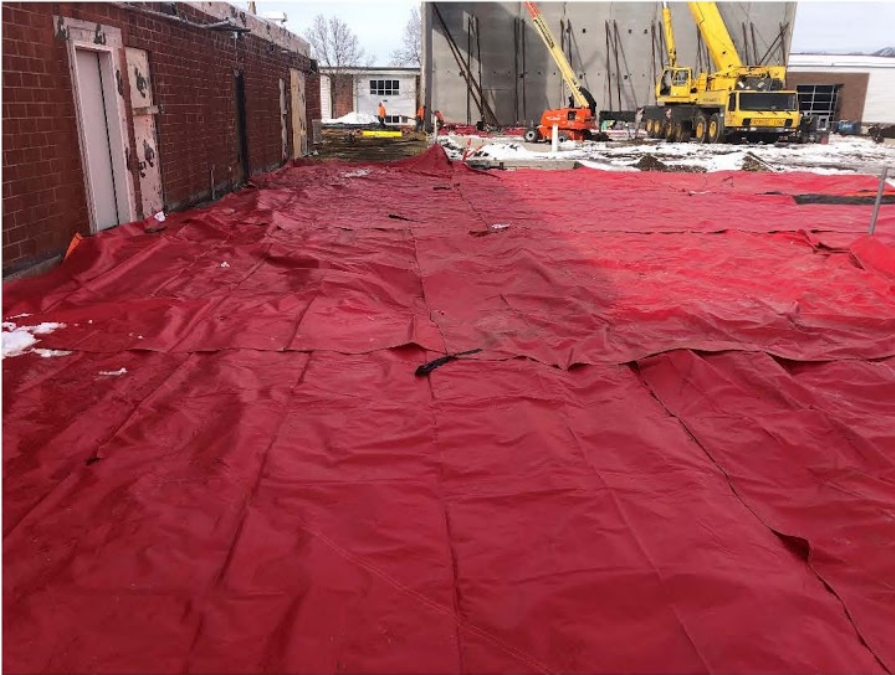
Fig 10: Heating Blankets for Concrete Slab
