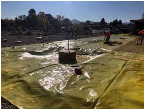
Fig D5: Vapor barrier installation and under slab preparation at learning community.
