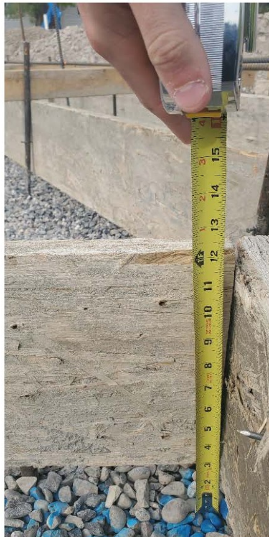
Image 6: Interior spread footing at auditorium C7. Depth to be adjusted
