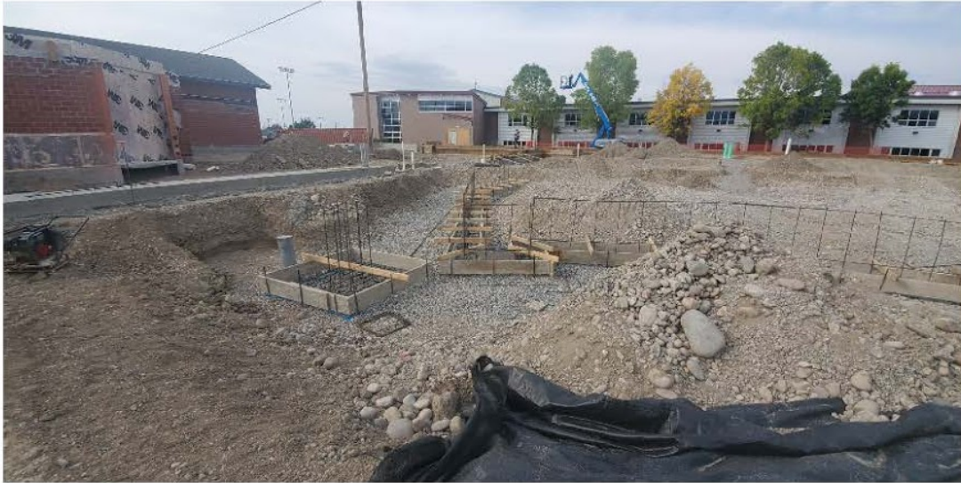
Image 1: Overall stage wall footings
