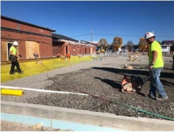
Fig 07: Vapor barrier installation and under slab preparation at learning community.
