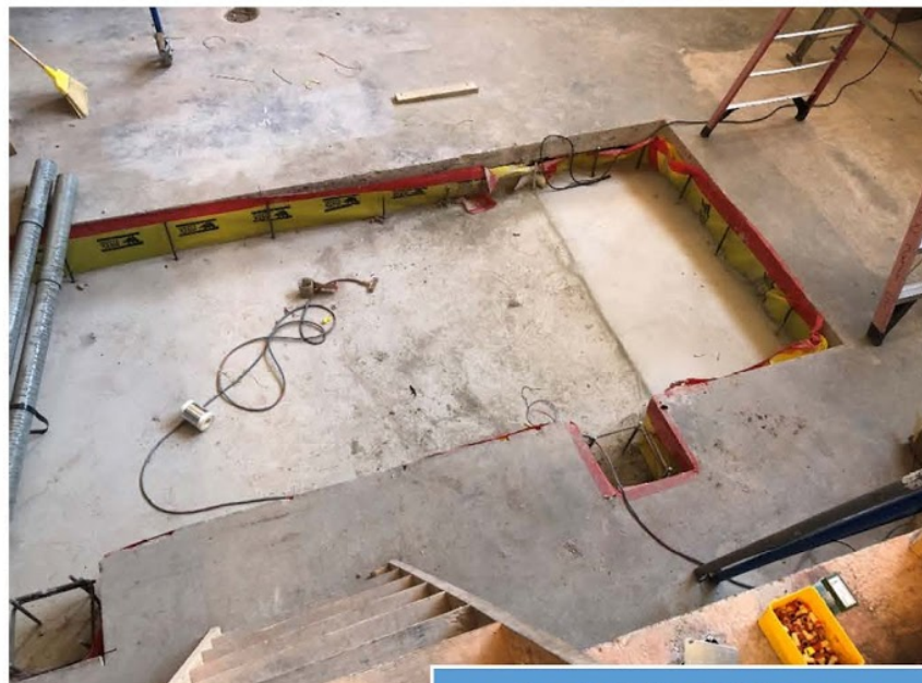
Figure 3-2: Building 4A Lift Pit Concrete
