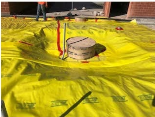
Fig D6: Vapor barrier installation and under slab preparation at learning community.
