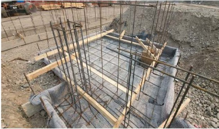
Image 1: Elevator pit foundation.
