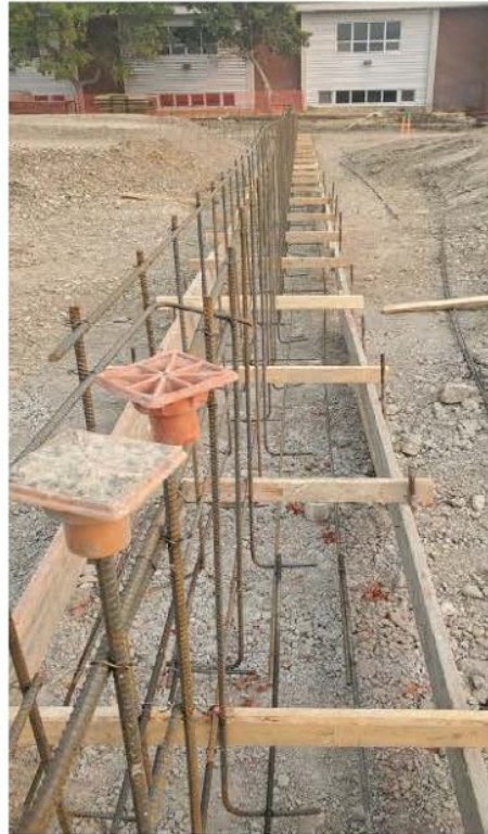
Image 6: Grid 1 footings and dowels.
