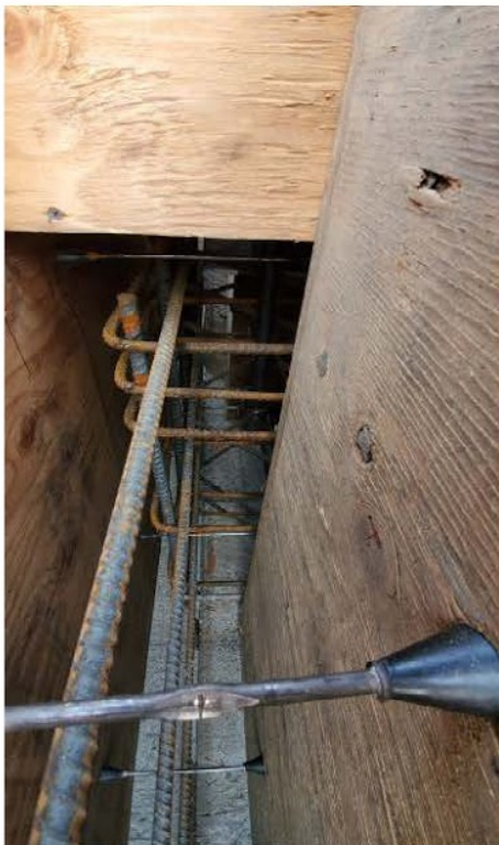
Image 3: Pier reinforcement along Grid BB.
