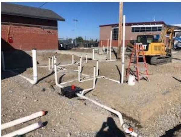
Fig 03: Underslab utility preparation at student commons.
