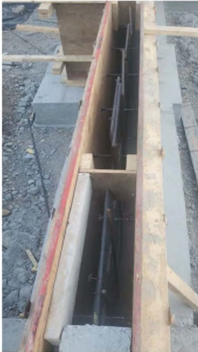
Image 1: Wall reinforcement and blockout and reinforcement at Grid F.
