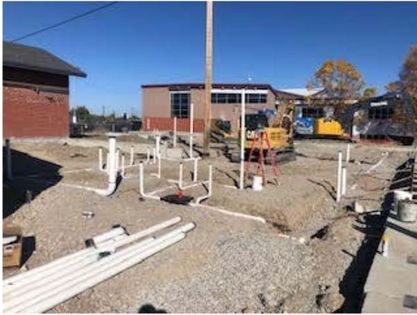
Fig D4: Under slab utility preparation at student commons.
