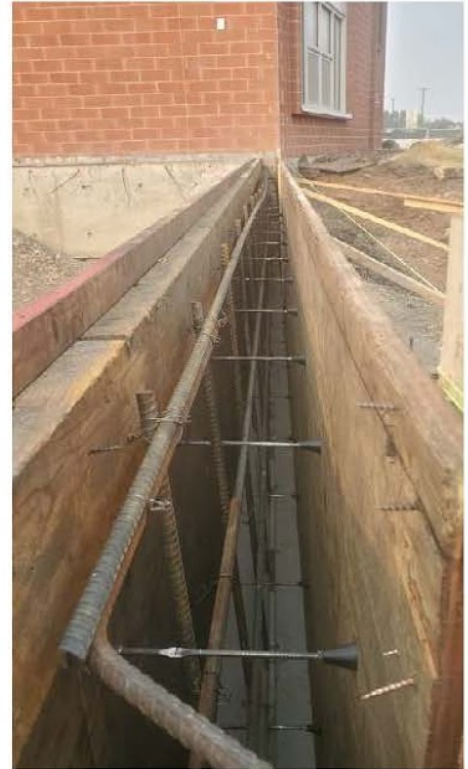
Image 2: Wall reinforcement north of Grid 4.
