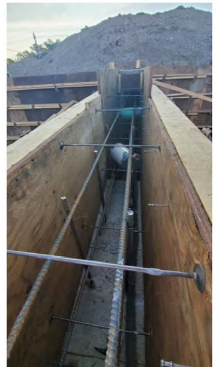
Image 6: Wall reinforcement at Grid 5.
