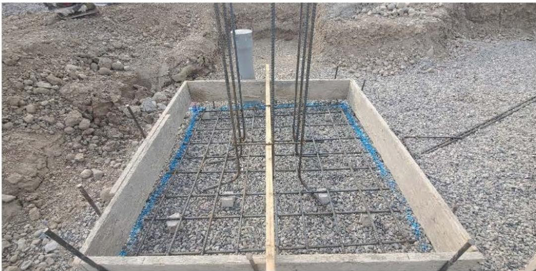
Image 2: Interior spread footing at auditorium C7
