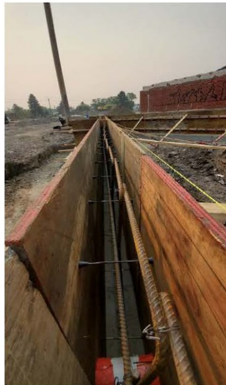
Image 4: Slab pourover dowels along Grid BB.
