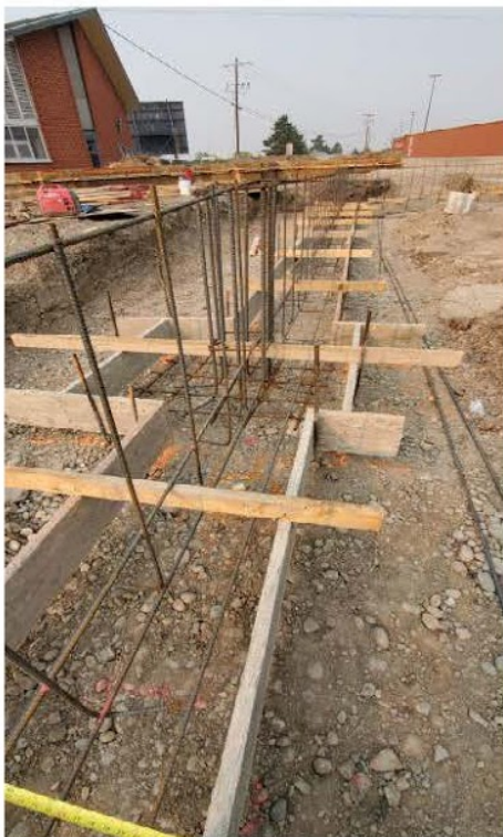
Image 7: Grid 2 footings and dowels.
