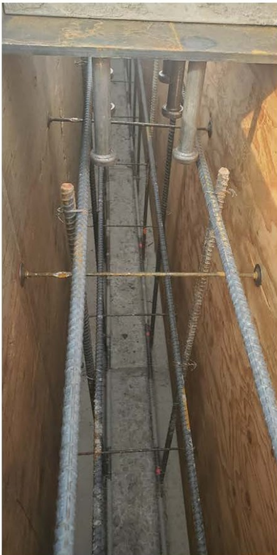
Image 5: Typical 12" wall reinforcement at precast walls
