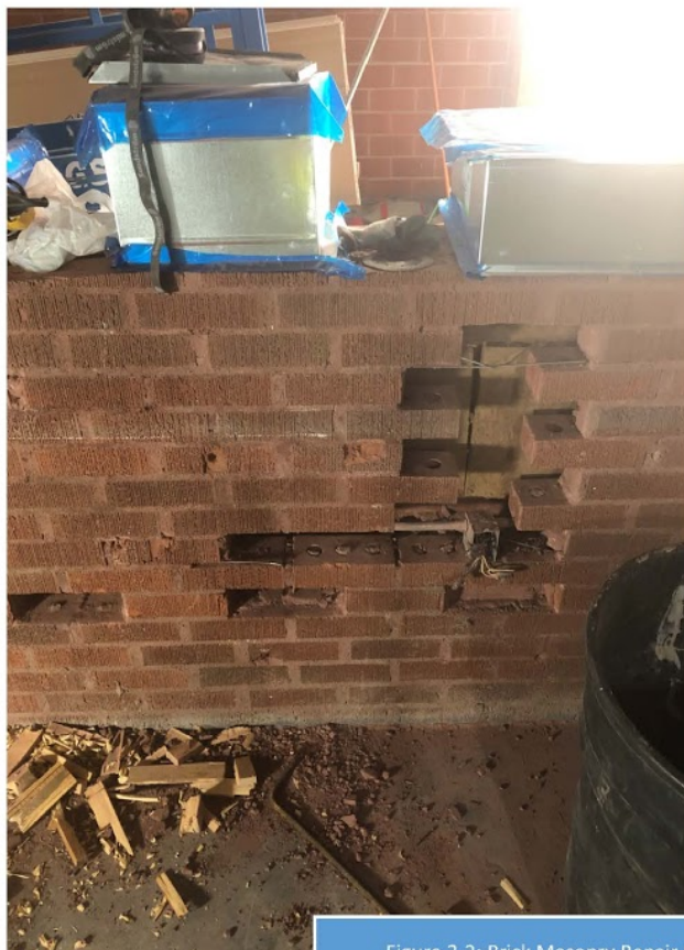
Figure 3-2: Brick Masonry Repair in F-wing
