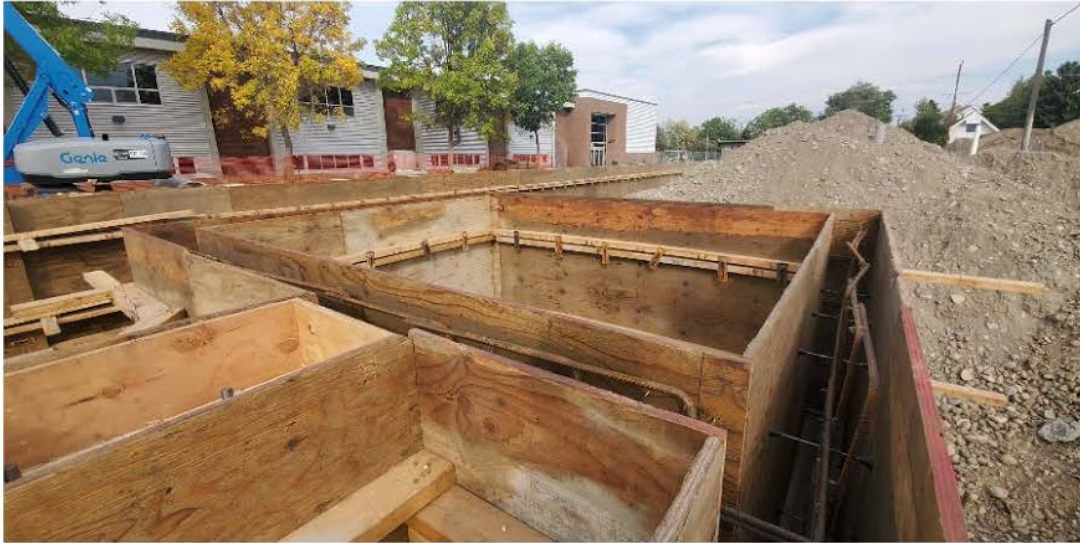
Image 4: Overall elevator pit wall forms
