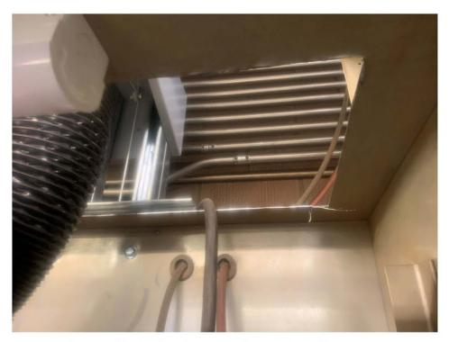
Figure 05: Hole cut in welding booth needs protective edging to safe guard fume arms
