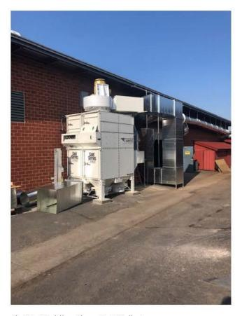
Fig 01: Welding Shop Dust Collector
