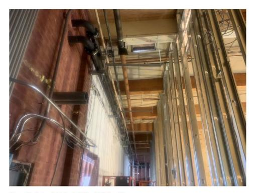
Figure 06: Hydronic Mains in F Wing (Building 4A)
