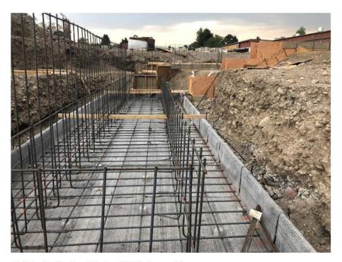
Fig 03: Auditorium Rigging Pit Waterproofing
