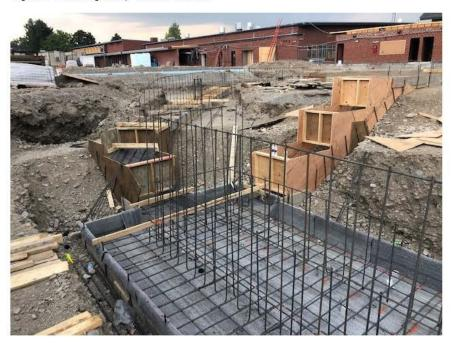
Fig 02: Auditorium Rigging Pit Waterproofing
