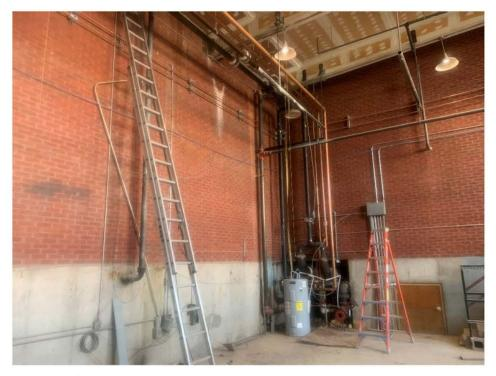
Figure 05: Hydronic piping connections to existing pipe
