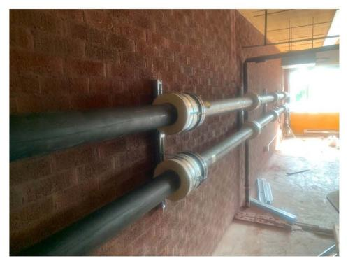
Figure 10: Hydronic mains in mechanical mezzanine
