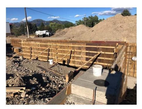
Fig 04: Foundation Formwork
