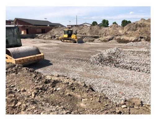
Fig 06: Site fill & Grading
