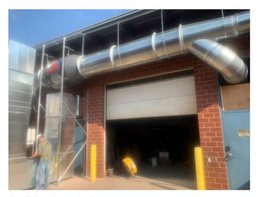
Figure 10: Ductwork over overhead door
