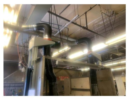
Figure 11: Duct connections at remote booths
