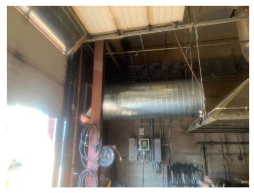
Figure 07: Perforated Supply Duct
