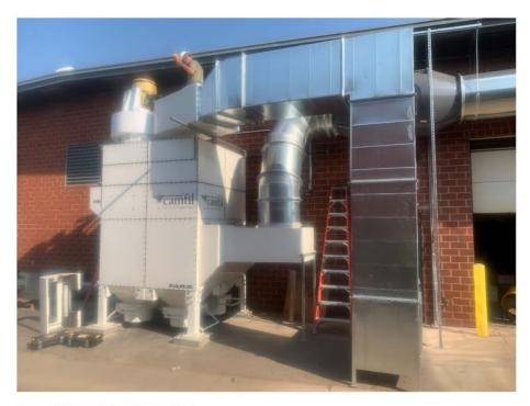
Figure 01: Metal Shop Dust Collector
