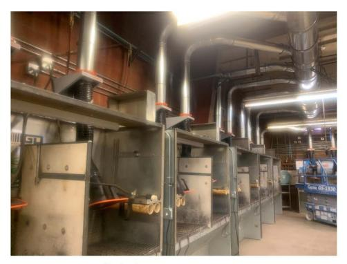
Figure 03: Connections at welding booths.
