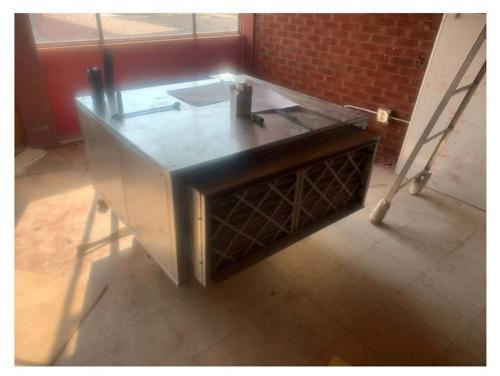
Figure 08: Blower Coil BC-1 not covered
