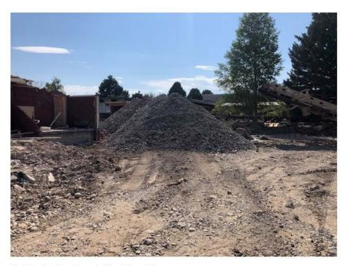
Fig 07: Crushed Foundation Material
