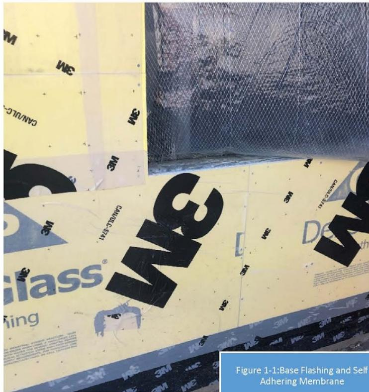
Figure 1-1: Base Flashing and Self Adhering Membrane
