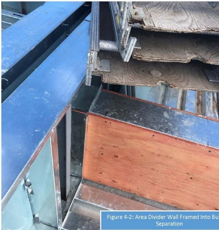
Figure 4-2: Area Divider Wall Framed Into Building Separation
