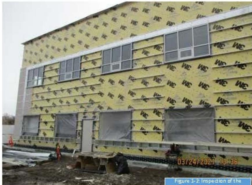
Figure 1-2: Inspection of the building's installed air/moisture/vapor barrier
