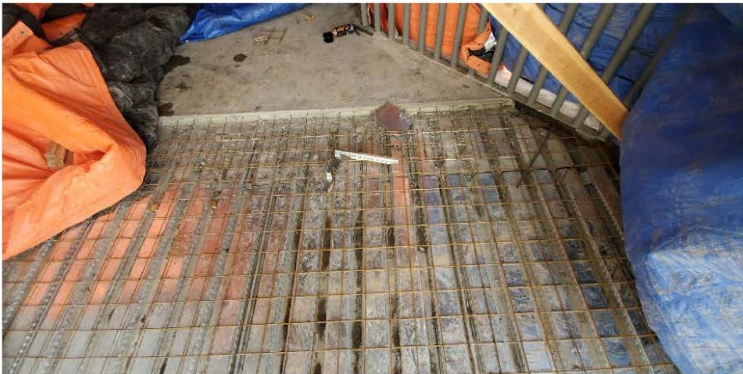
Image 5: Typical lapped welded wire at slab joint
