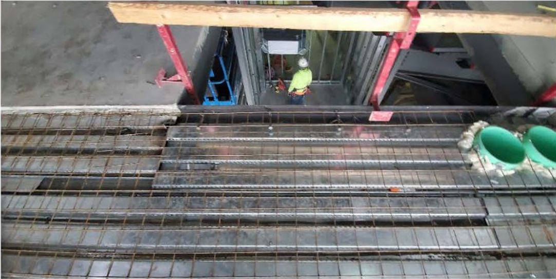
Image 1: Typical HAS at slab edge.
