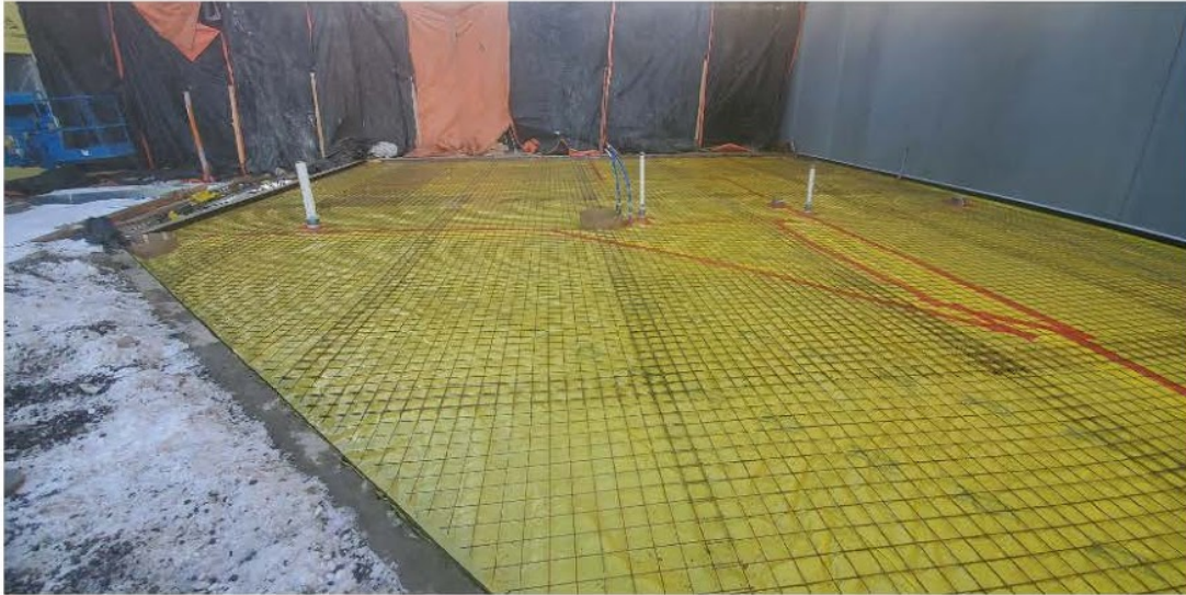
Image 1: Typical reinforcement (unchaired)
