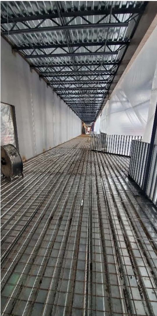
Image 2: Typical Welded Wire Reinforcement (unchaired) second floor.
