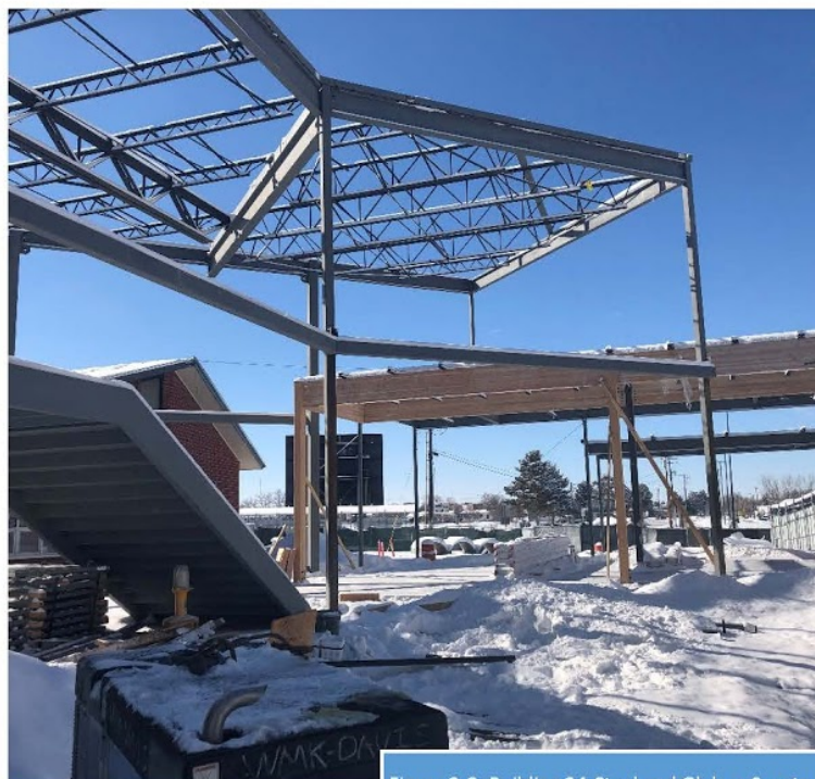
Figure 3-2: Building 2A Steel and Glulam Construction
