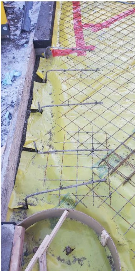
Image 2: Pourover reinforcement and missing trim bars at column
