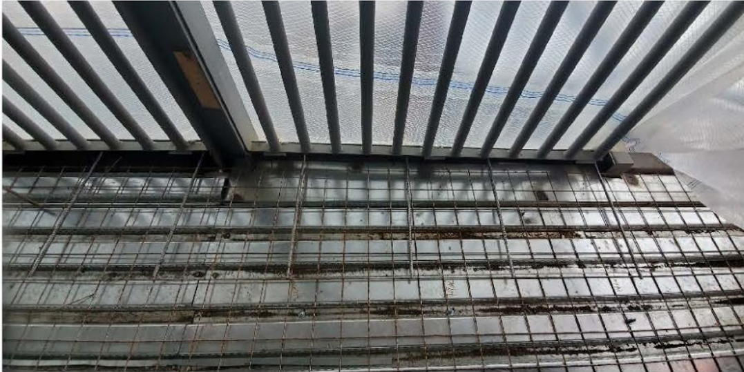
Image 4: Typical welded rebar at slab edge.
