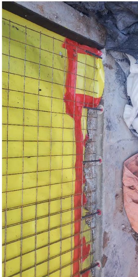
Image 3: Smooth dowels at slab joint
