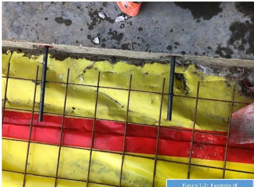
Figure 1-2: Example of Penetrations in Vapor Barrier
