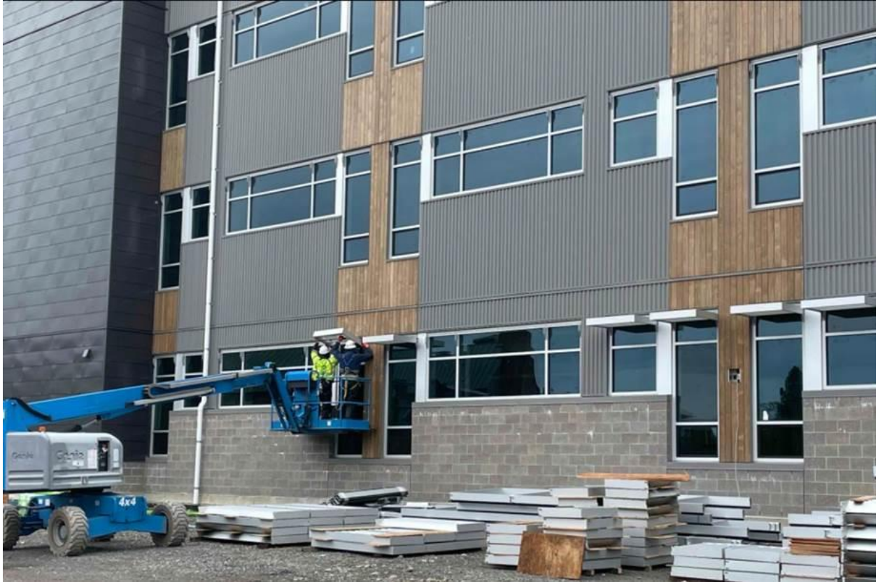
Installing sunshade on the south side of the Academic Wing
