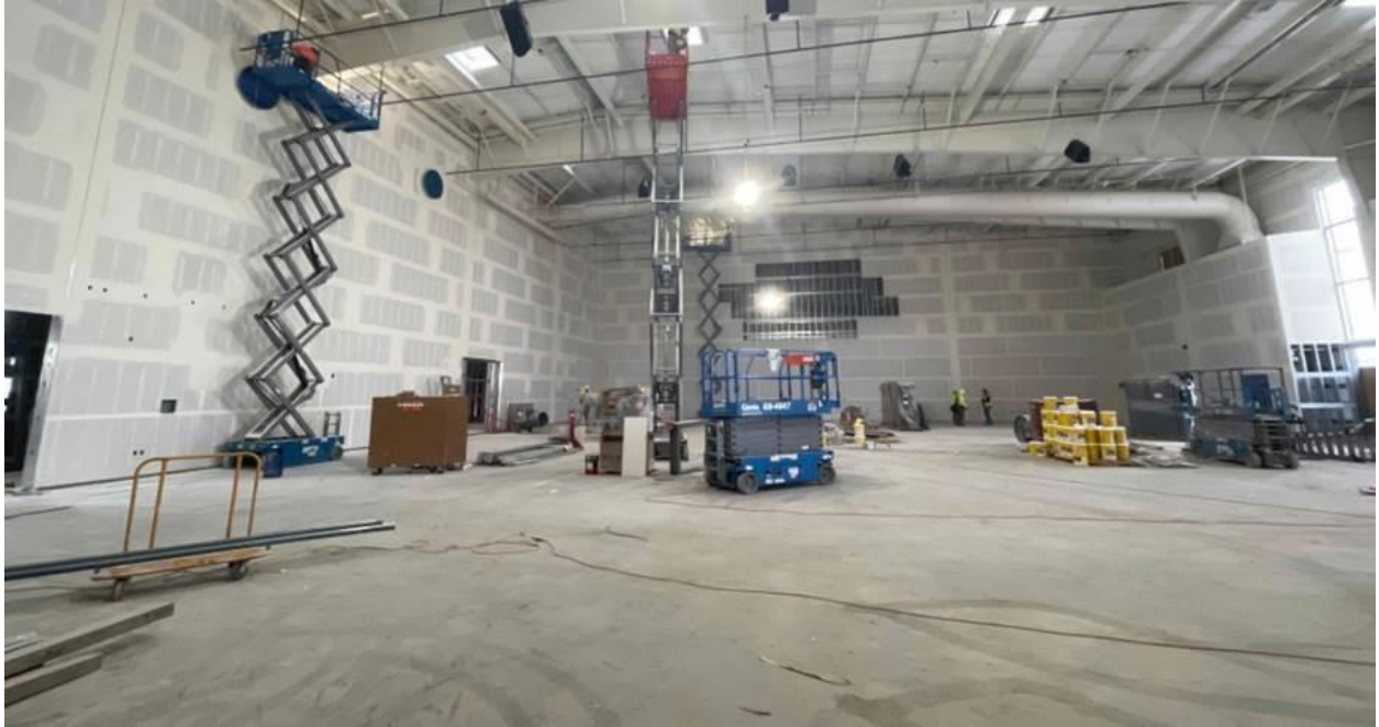
Mudding and taping the sheetrock joints in the Main Gym
