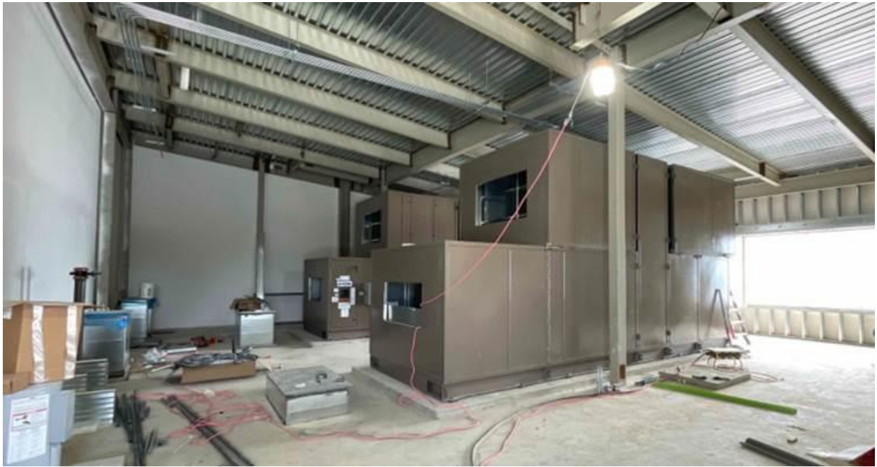
Installing air handling equipment in the Academic Wing
