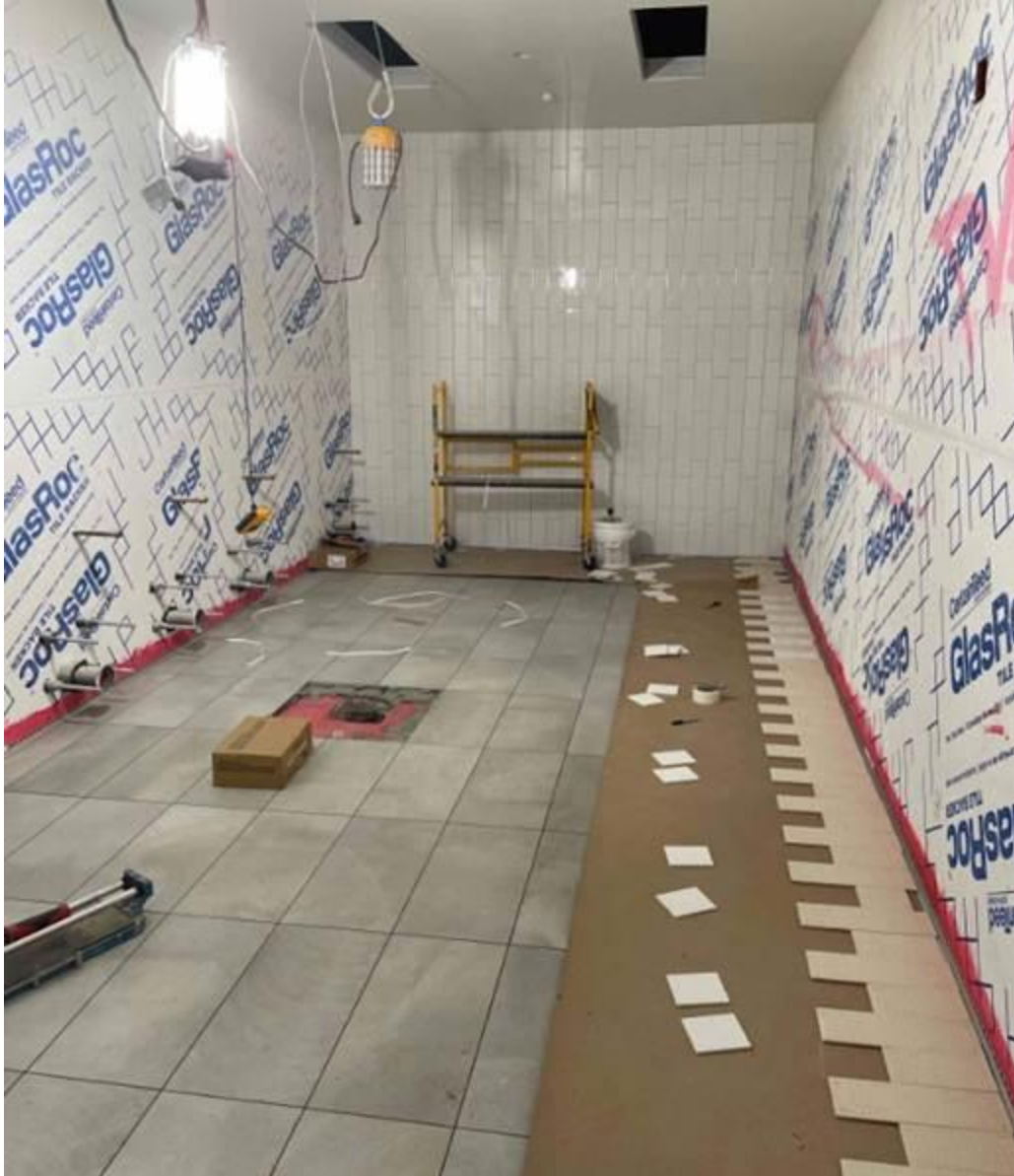
Installing bathroom tile in the Academic Wing
