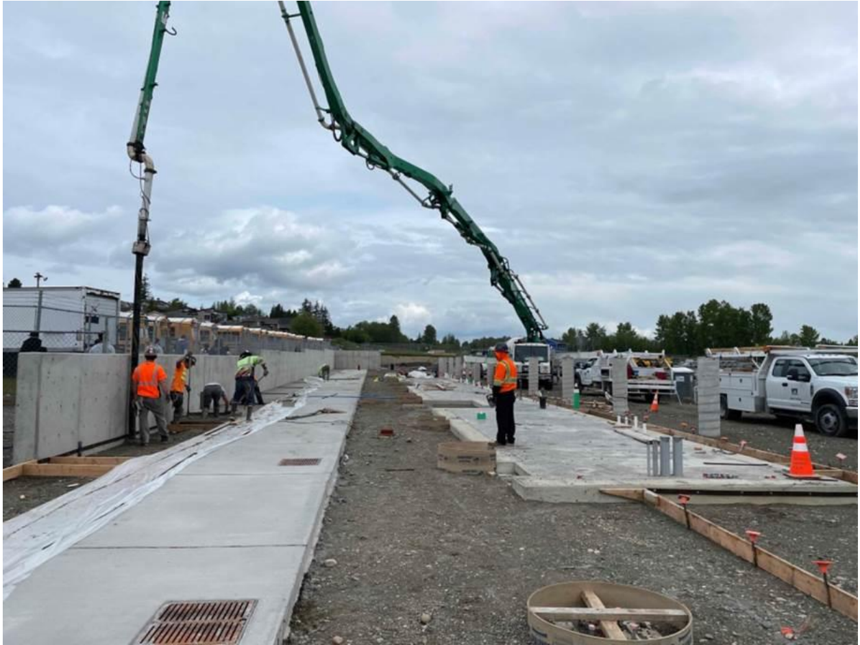
Pouring hardscapes around the Grandstand area
