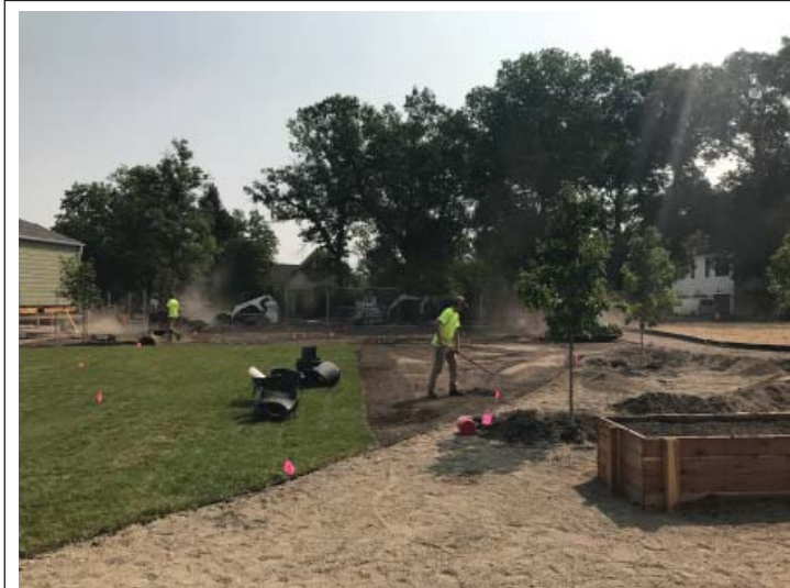
Final grading, sod installation and tree planting on north end of playground area.
