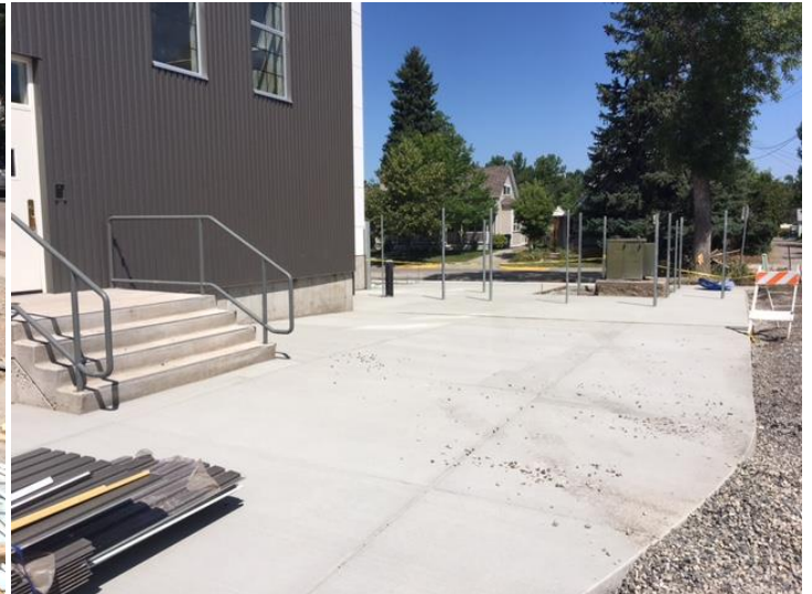
New Concrete Apron Slabs
