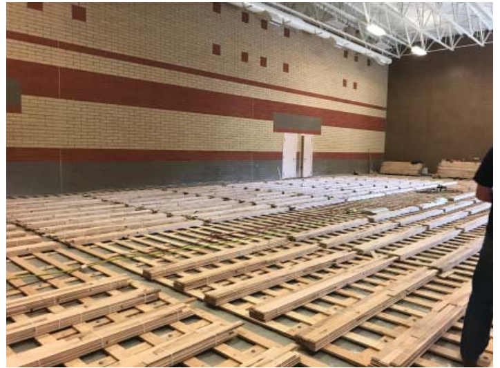
New secondary gym space. Wood flooring being acclimated prior to installation.
