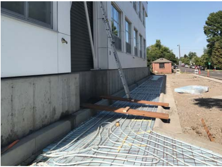
Snow melt system installed along sidewalk section north of the new addition.
