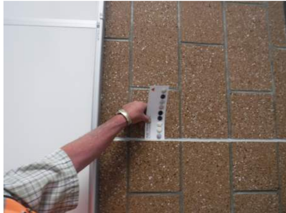
New joint color selected to match darker grout with anti-graffiti
