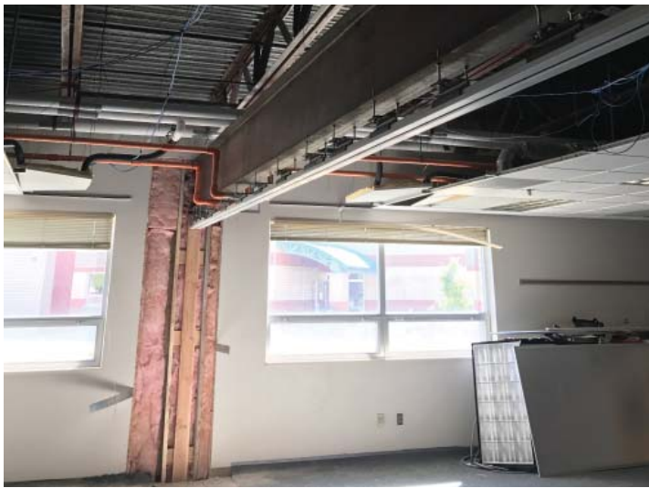
Demo and prep work for new classroom operable partition wall.
