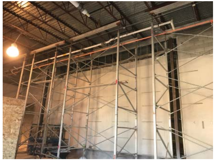
Falsework for wall removal to make space for new music rooms.
