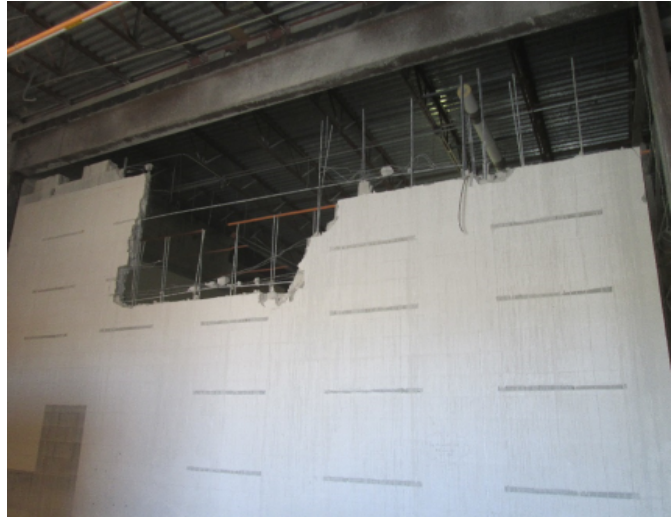
Area B 8 grade wing Operable Partition track and Framing
