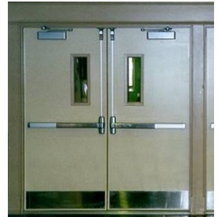
Panic Hardware required by code at rooms over 1000 sq. ft (Requires a key)
