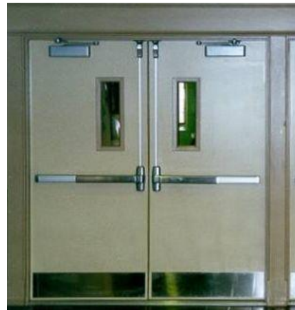
Panic Hardware on inside of exit doors
