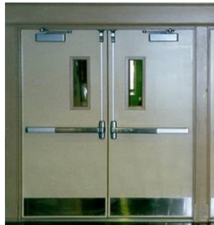
Panic Hardware on inside of exit doors
