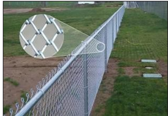
Chain link perimeter fencing
