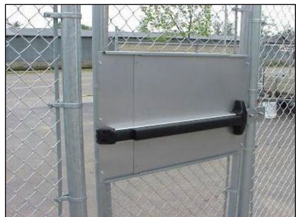
Gate with exit device for safe dispersal
