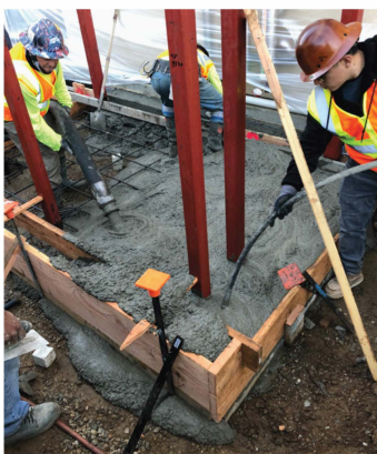
Pouring concrete for air conditioning at Alvarado Elementary School
