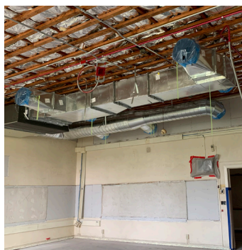
Installation of air conditioning equipment in a classroom at Madison Elementary
