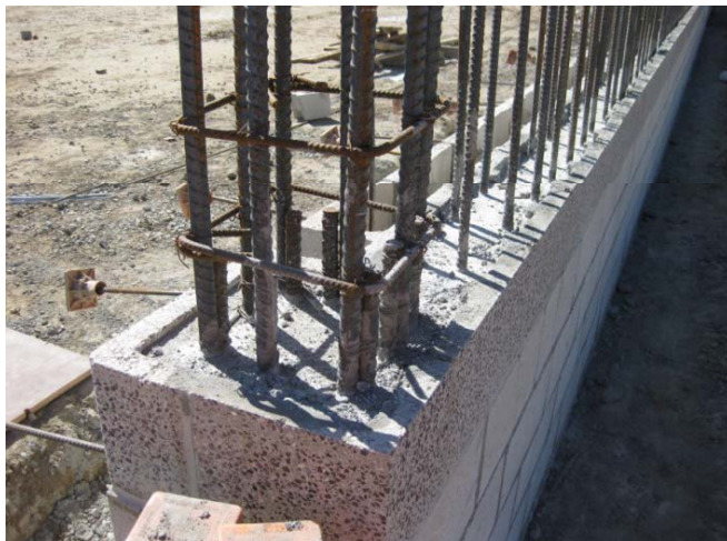
CMU First Lift Grout
