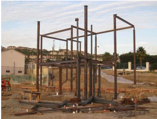
Early Steel Erection
