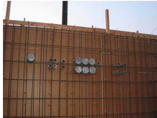
Electrical Sleeves through Retaining Wall
