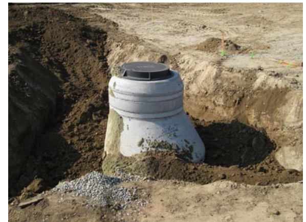
Courtyard Sewer Manhole
