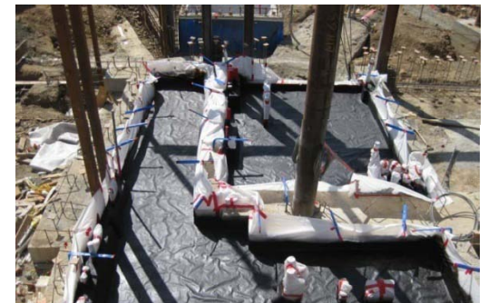
Electrical Room Methane System
