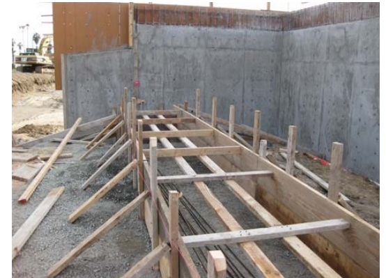
Grade Beams and Retaining Walls
