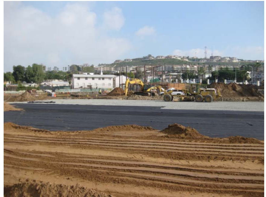
Athletic Fields Backfill
