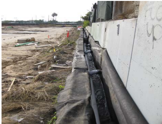
North Storm Drain Line
