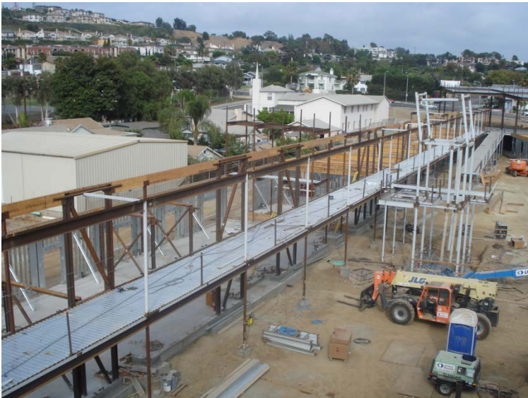
View of Buildings B and C with Access Ramp
