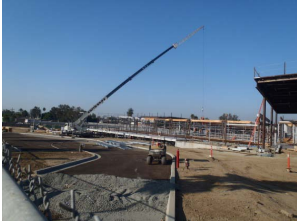
View of Building A from Entrance Drop-Off Area
