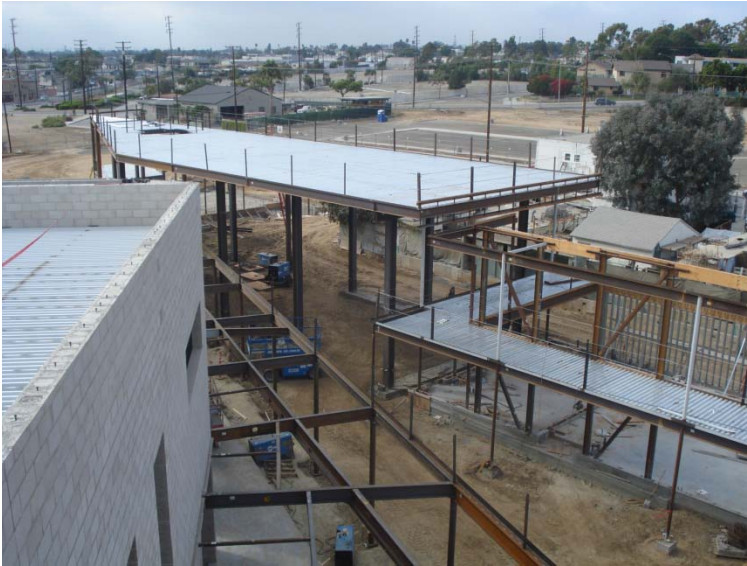
View of Eating Shelter with Building E behind
