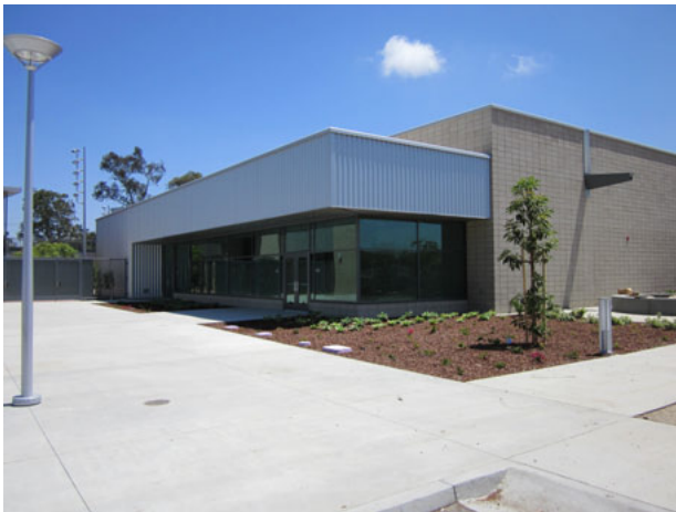
View of Bldg. I (Lecture Hall)
