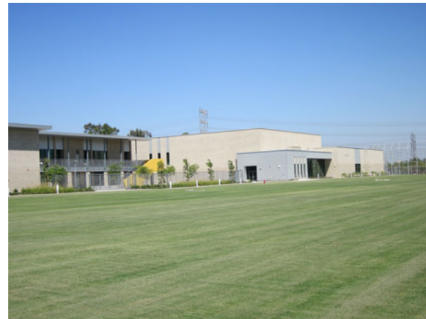
View of Bldg. E (Gymnasium)
