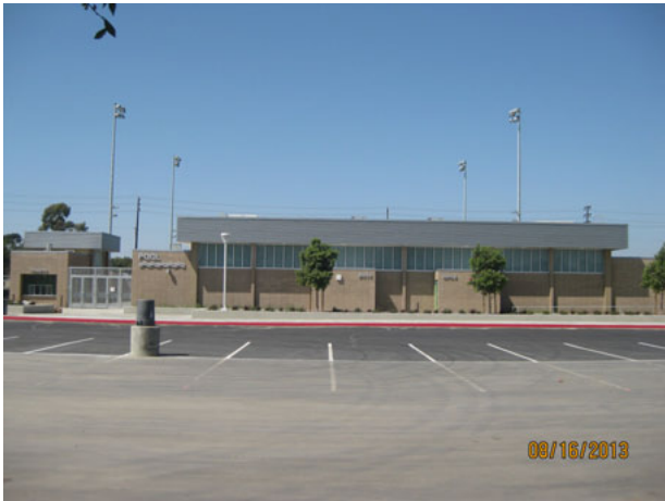
Ticket/Concession and Locker Room Bldg.
