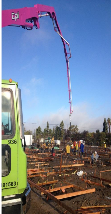
Building A North Foundation
