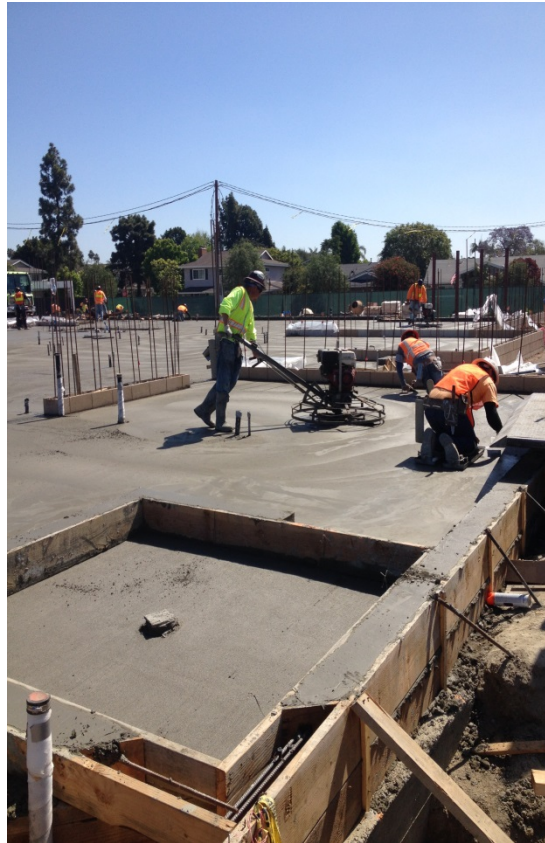
Finishing Concrete Bldg A
