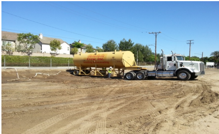
Setting up water tower for dust control
